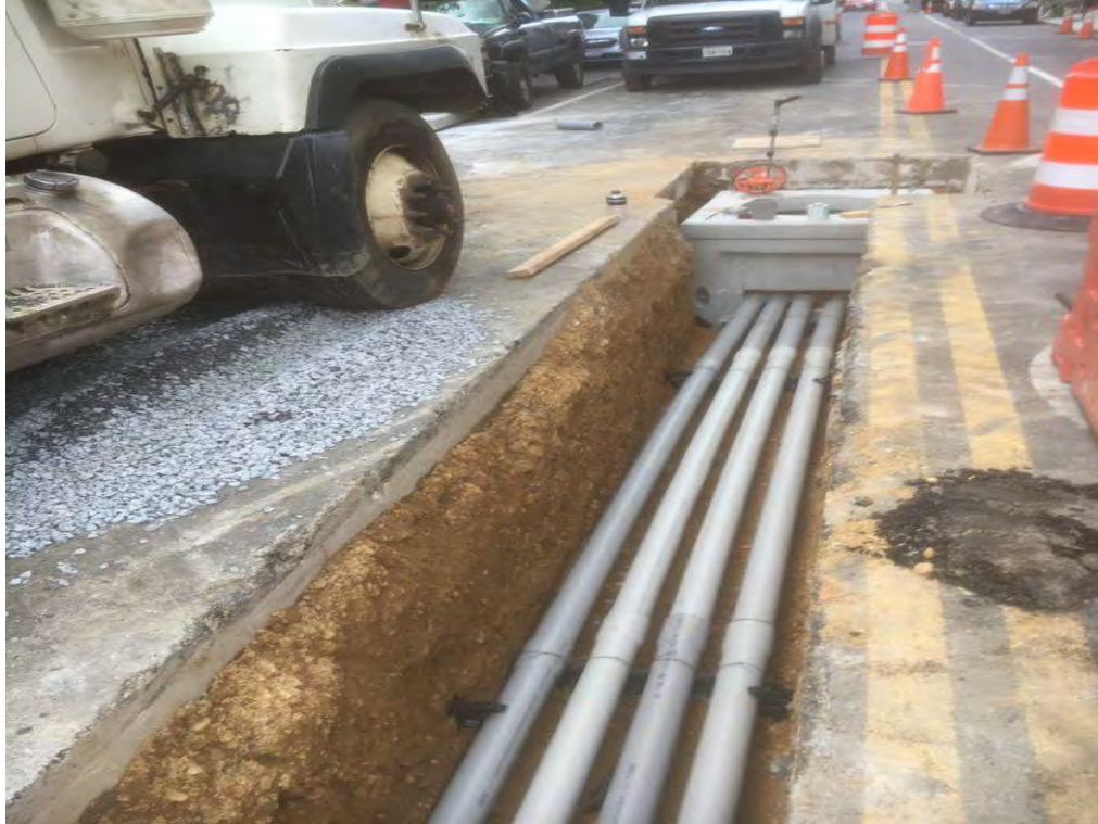
Installation of PVC Conduit on the Westside of N Street
