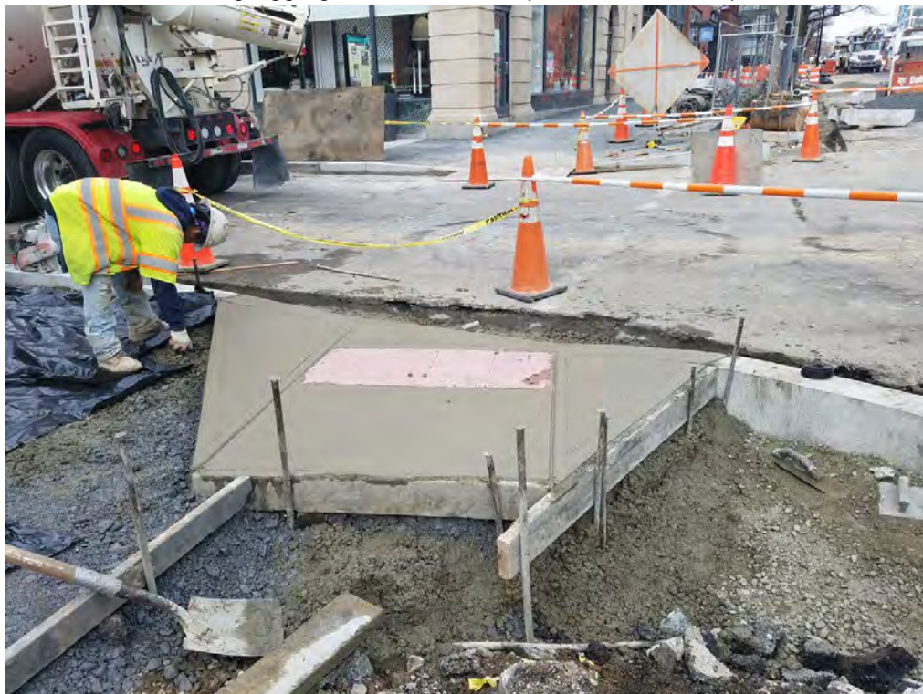
Installation of ADA Ramp at SW Corner of Church Street
