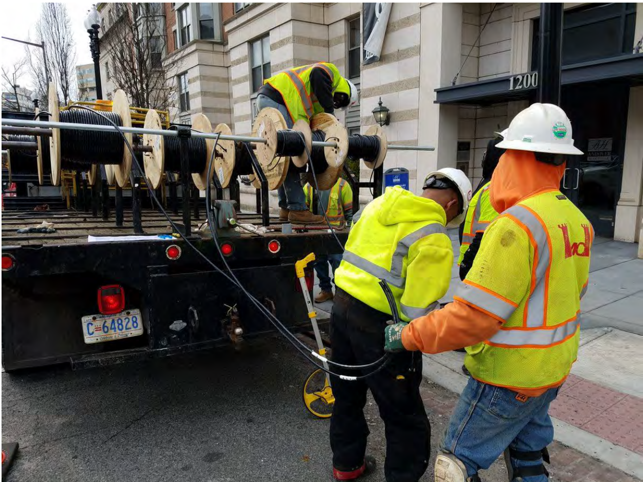
Installation of New Traffic Signal Cables at 14 th and N Street
