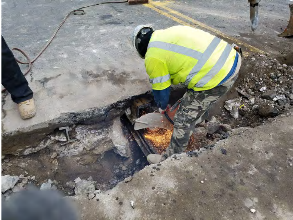
Removal of Street Car Tracks between Swann and T Street
