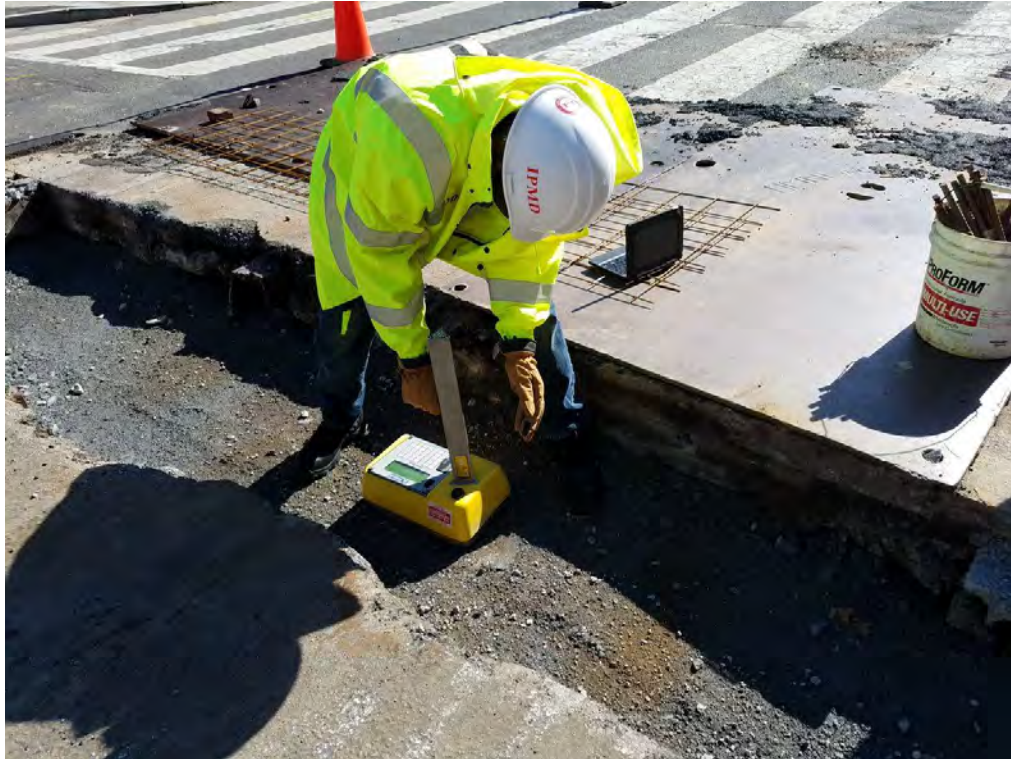
QA/QC testing Aggregate Base Material prior to PCC Base placement
