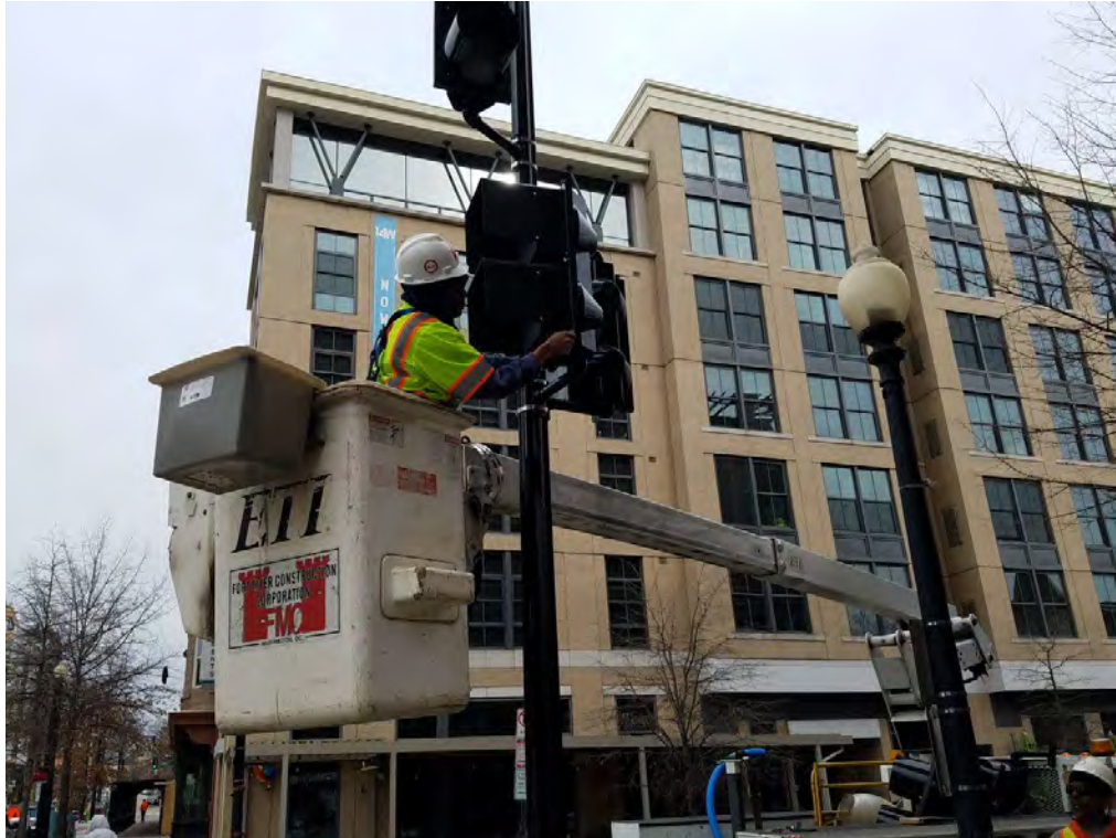
Construction of Temporary Traffic Signal
