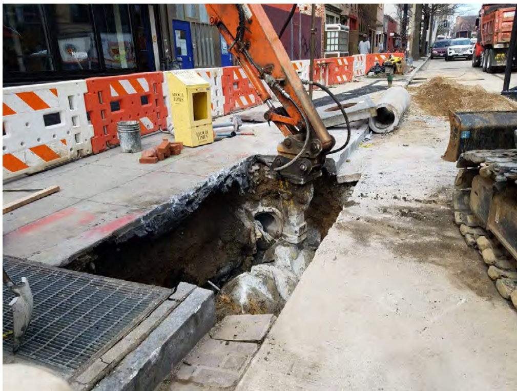
Abandonment of existing catch basin at 14 th and W Street
