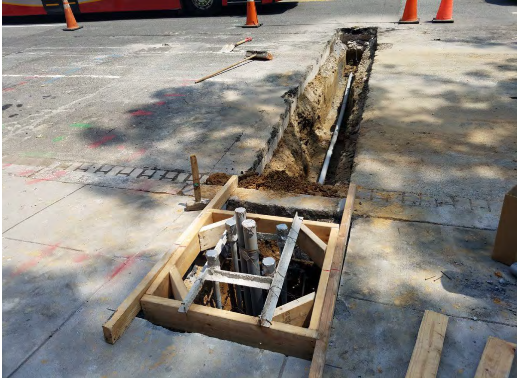
Installation of new Streetlight Foundation between P Street and Church St.
