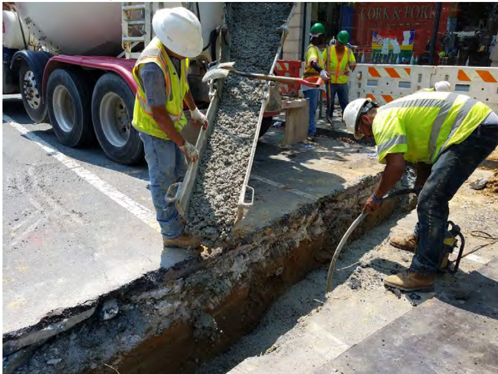
Encasement of 2" PVC Conduit for Lateral between P Street and Church St.
