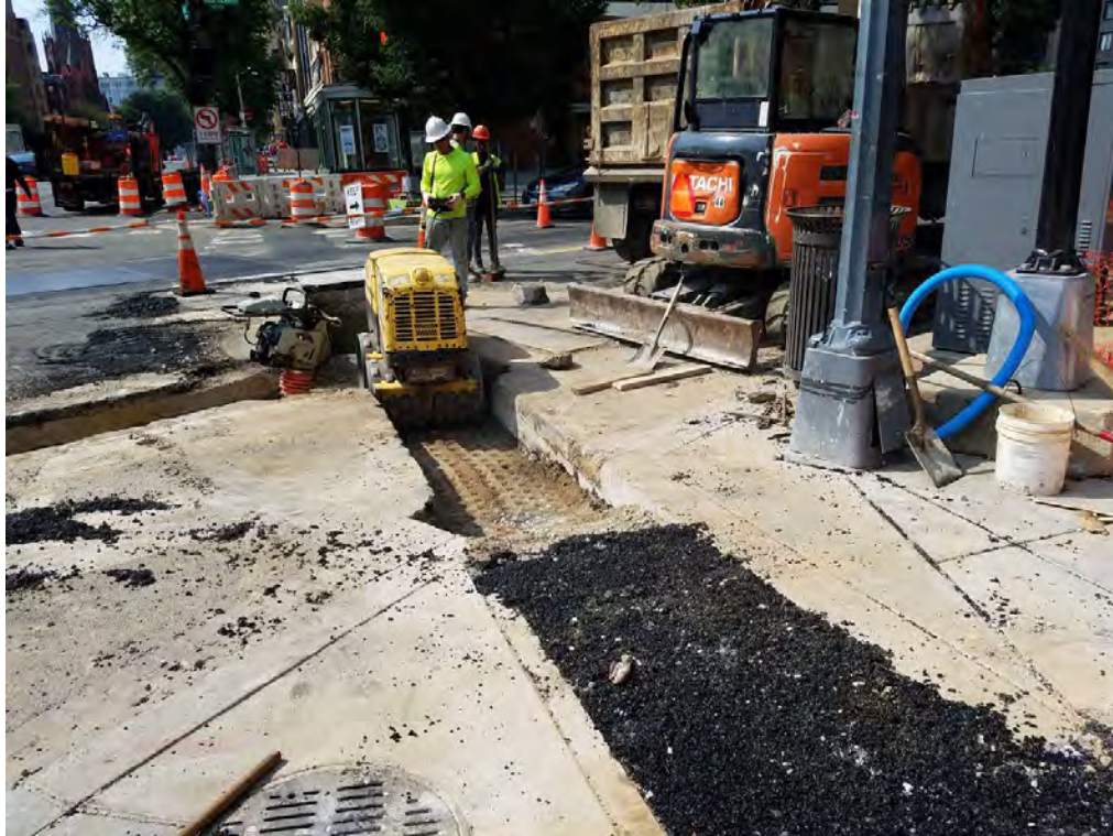
Compaction of RC-6 material at the NW corner of P Street
