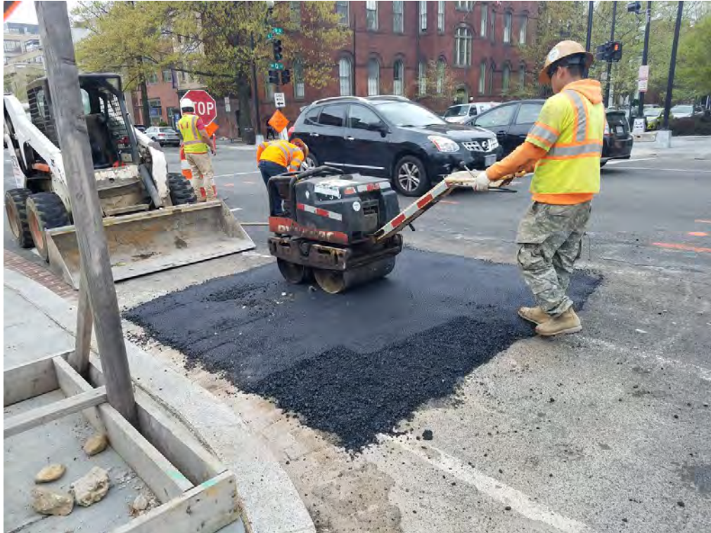
Compaction of Temporary Asphalt over Water Main work
