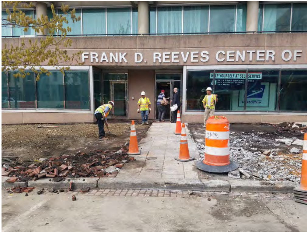
PCC Sidewalk Replacement on 2000 Block of 14 th Street
