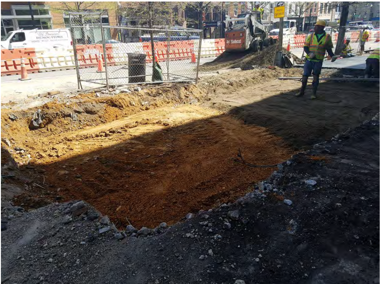
Installation of Structural Soil on the 2000 Block of 14 th Street
