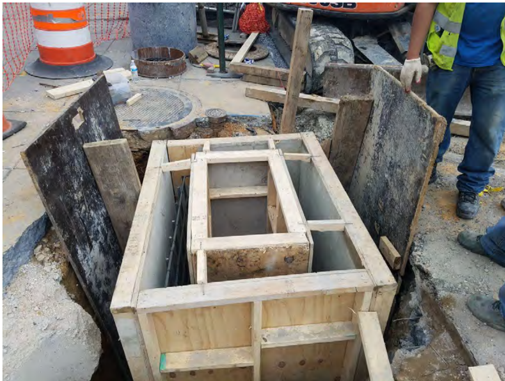
Formed and Poured Cast in place Catch Basin (CB-15)
