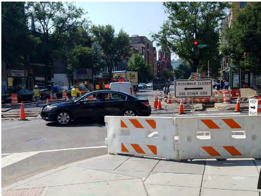
MOT Setup for Crosswalk Closed with Sign and Barricade
