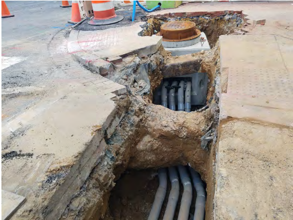
Installation of Manhole on the NW corner of Rhode Island Ave
