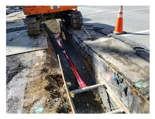
Placing Metal Tracking Tape in between backfill per Specifications
