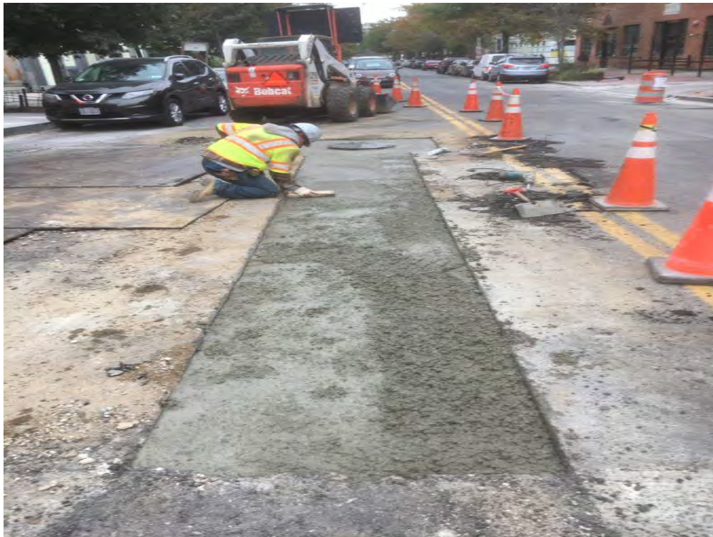
Placement of PCC Base on the Westside of Florida Ave
