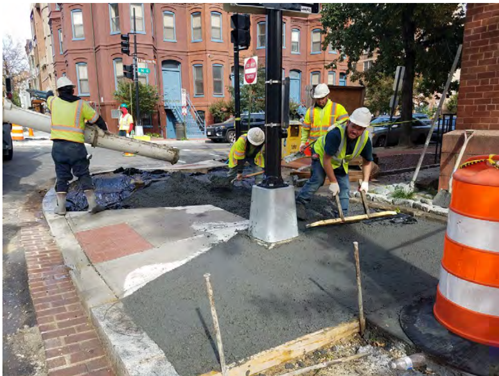
Placing PCC Sidewalk at SE corner of 14 th and N Street
