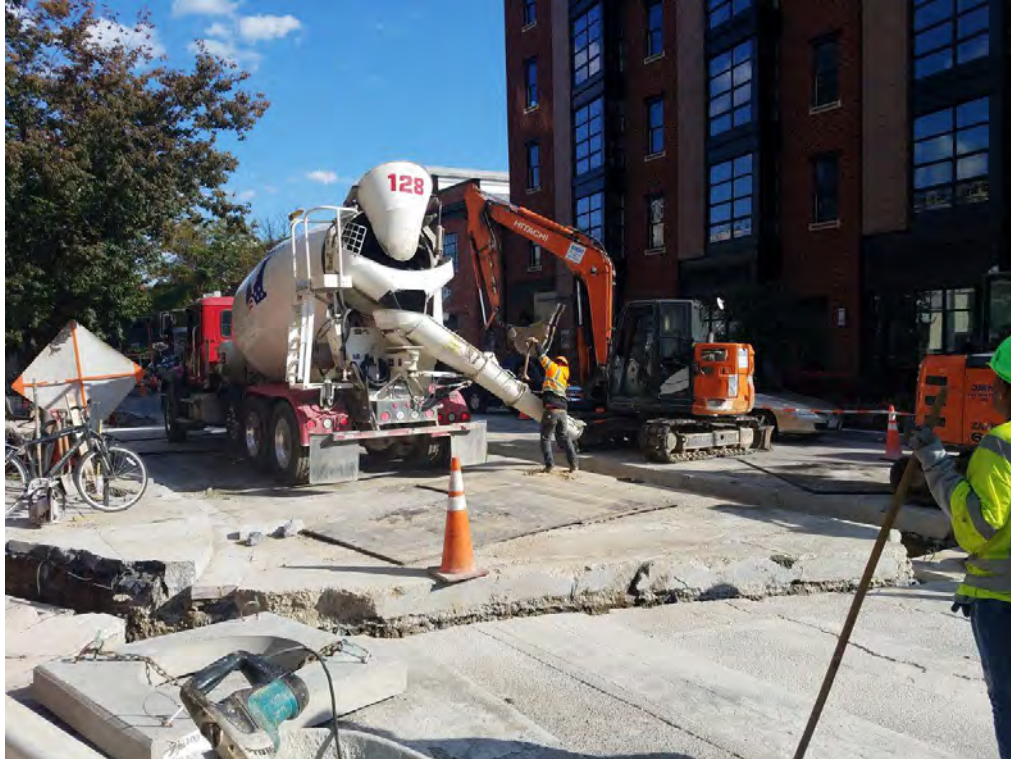
Encasing PVC Conduit in Electrical Trench at 14 th and Florida Ave
