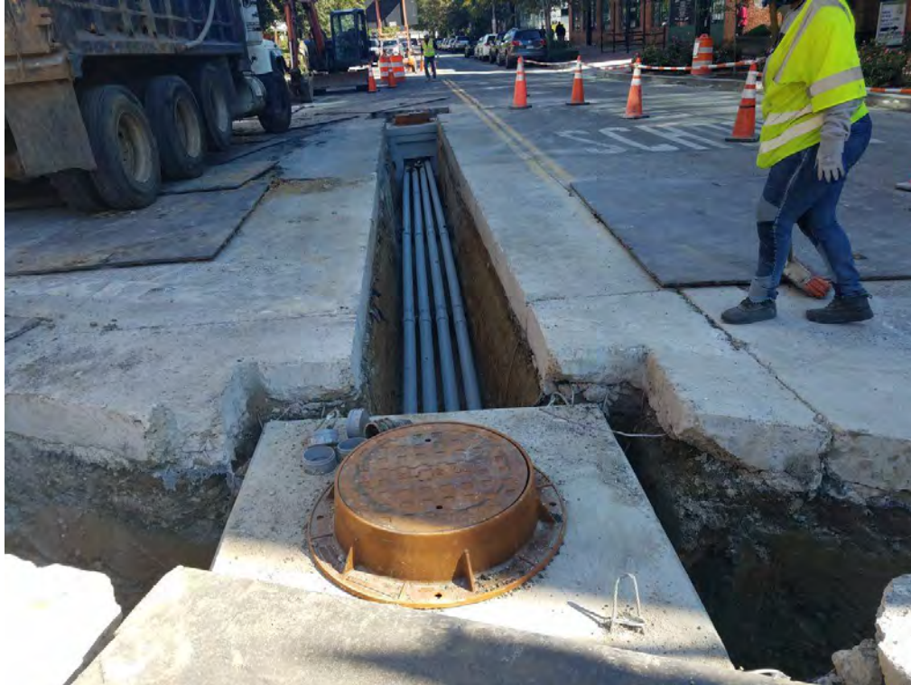
PVC Conduit installed in Electrical Trench at 14 th and Florida Ave
