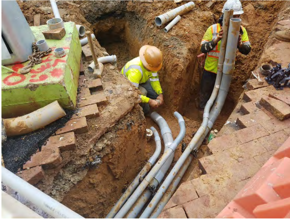
Installation of PVC Conduit for Traffic Signal and Street Lights
