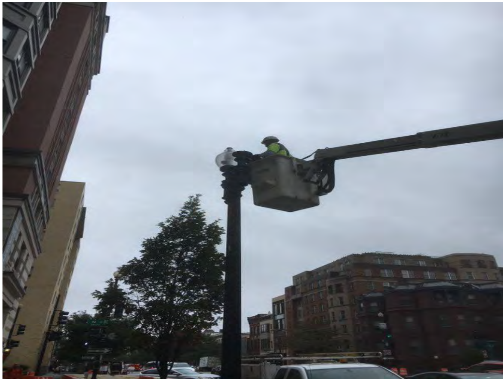
Installing the 100-watt LEDs and Globes on Twin 20 Street Lights
