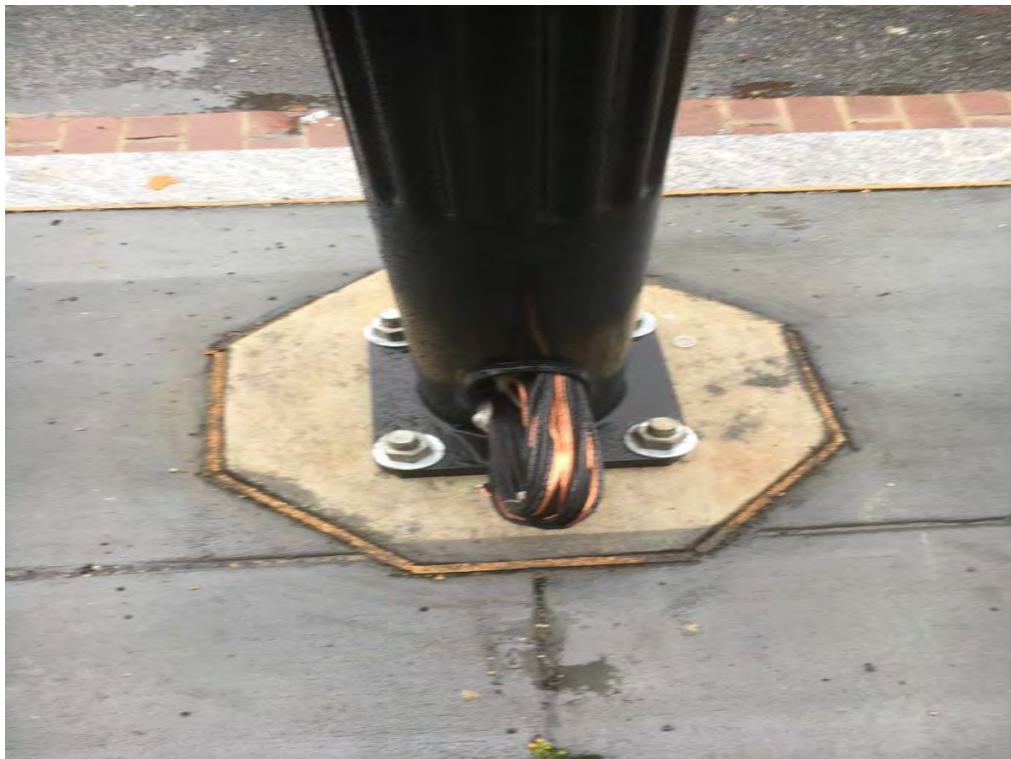
Pulling #10 and #8 wire for Street Lights
