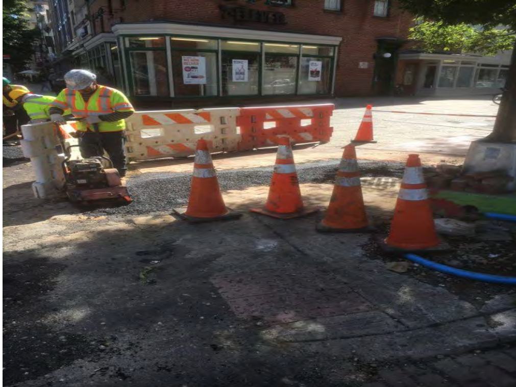
Placing Temporary Asphalt over Electrical conduit trenches
