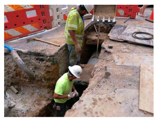
Installation of 15" PCC Connection Pipe for the Double Catch Basin on the NE Corner of P Street
