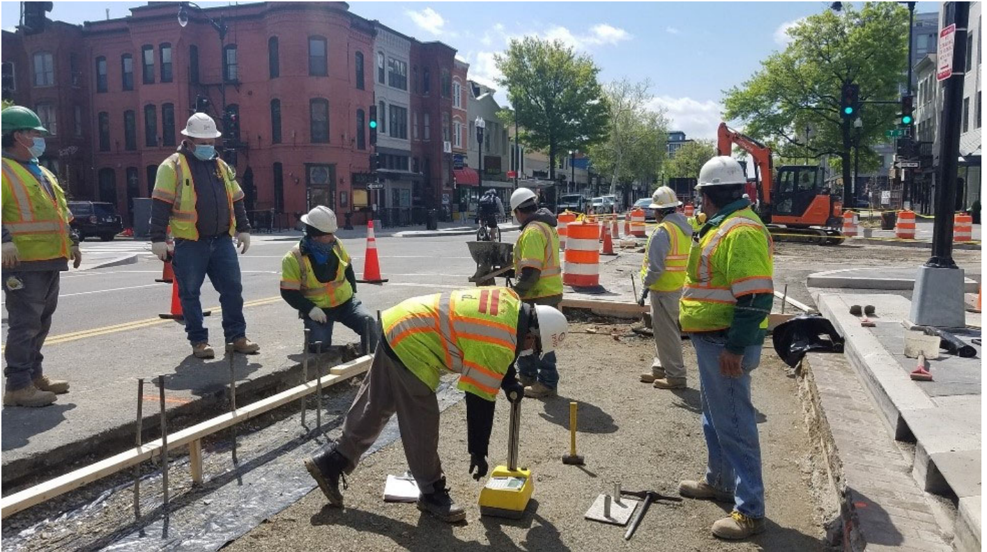
DDOT Tech onsite to perform compaction test
