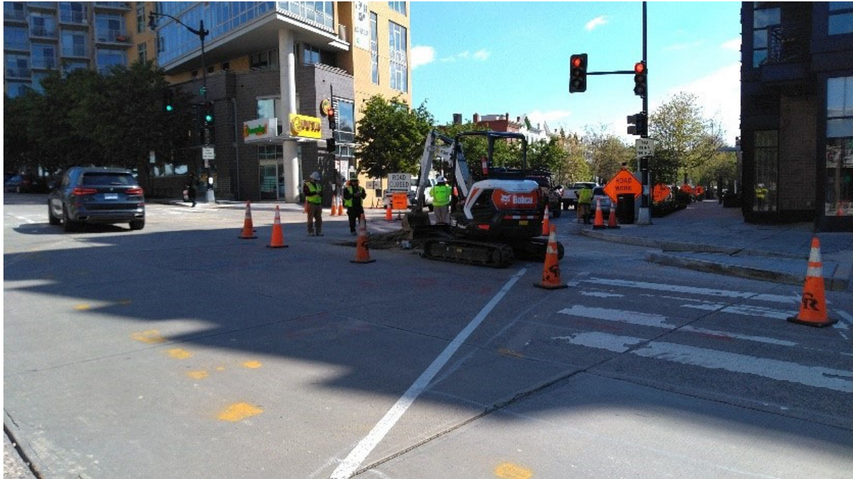
MC Dean Repairing Broken Conduit At Florida Ave.
