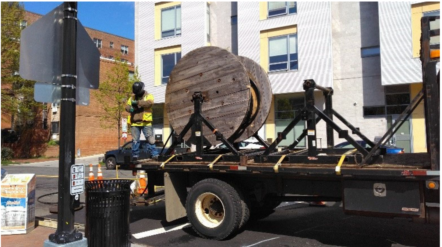
Installation of 1-100 pair Cable at Florida
