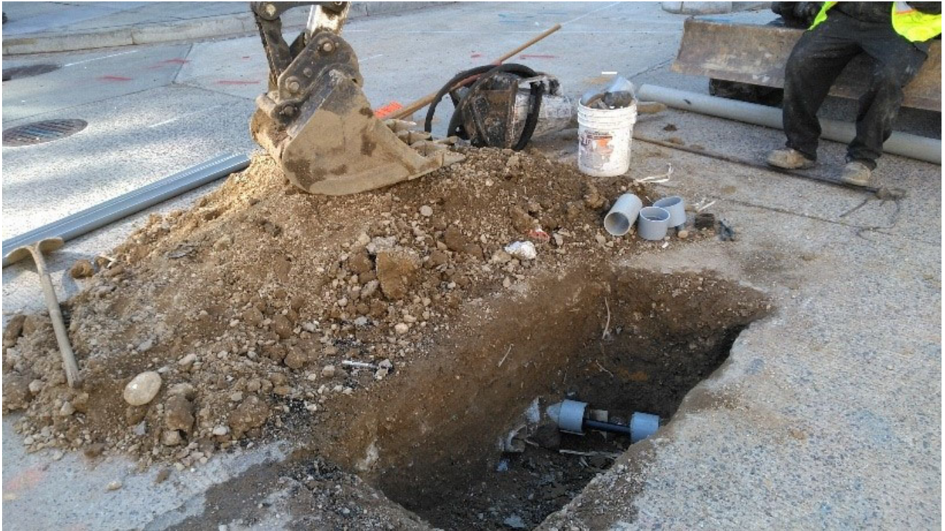
Broken conduit repair by MC Dean
