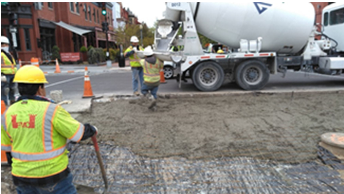
Placing Concrete PCC base repair
