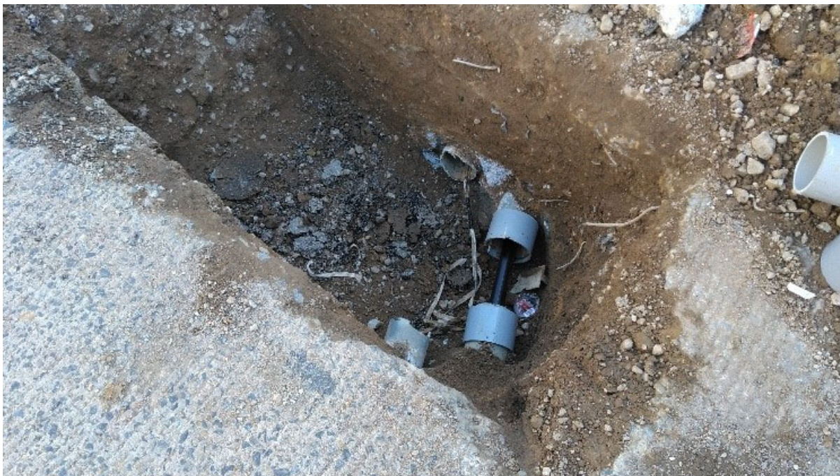
Broken Conduit was found
