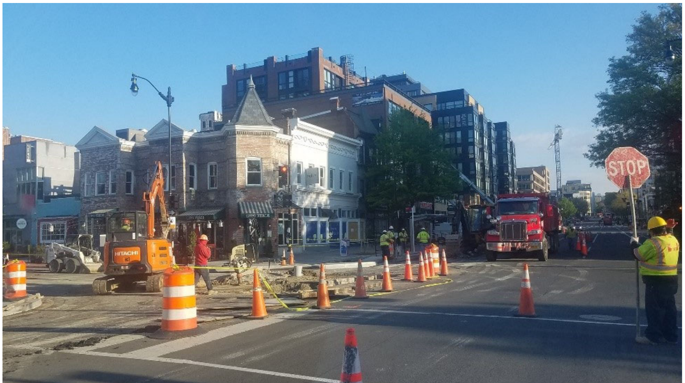
Backfilling to prepare for concrete placement in the proximity of T Street
