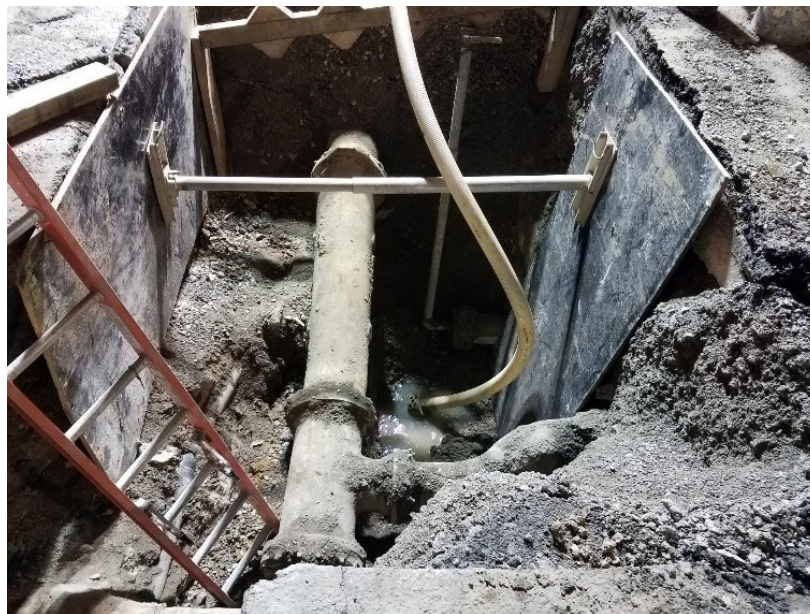
T Fitting . Night work .- T street
