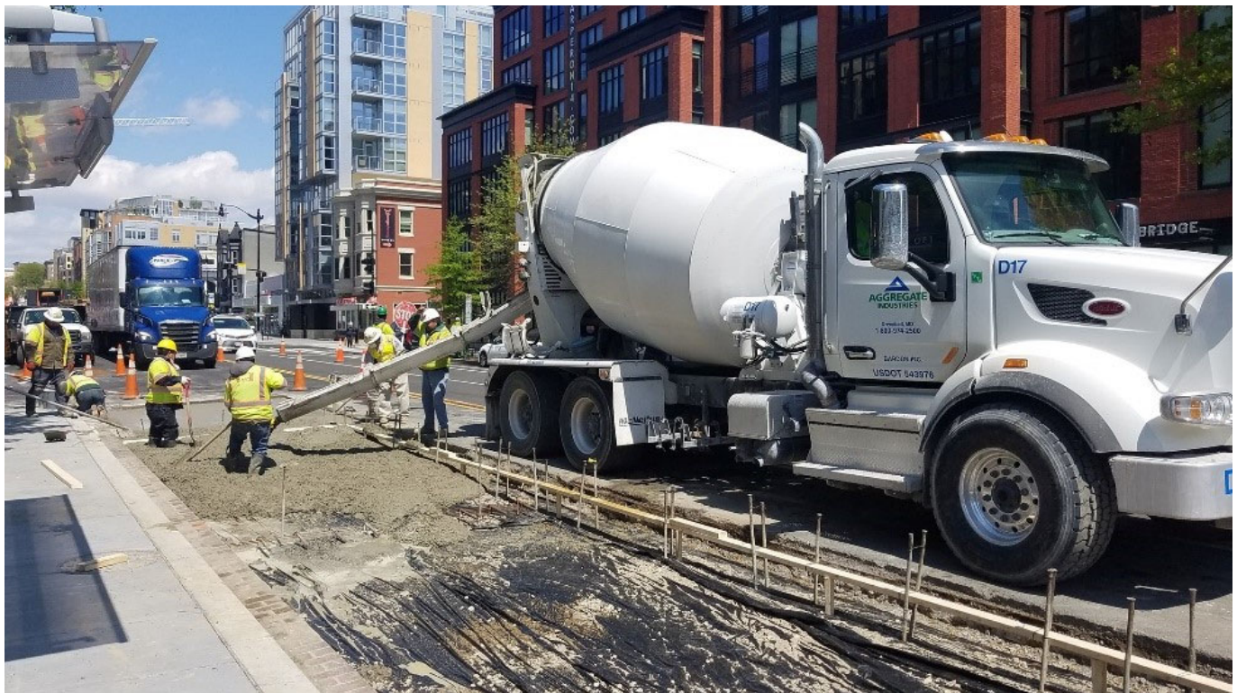
Concrete placement for the bus pad
