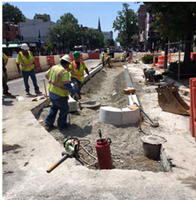
Circular curb installation.
