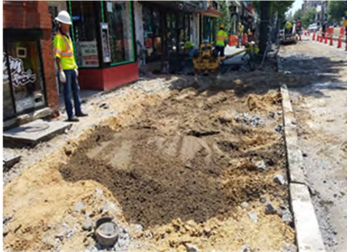
Tree zone at 1841 14 th St with structural soil placement.
