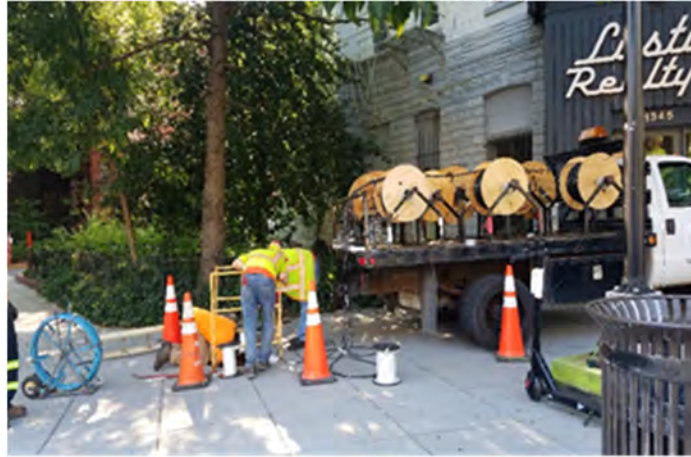
Cable pulling truck at SEC of 14 th & RIA near M18 manhole.
