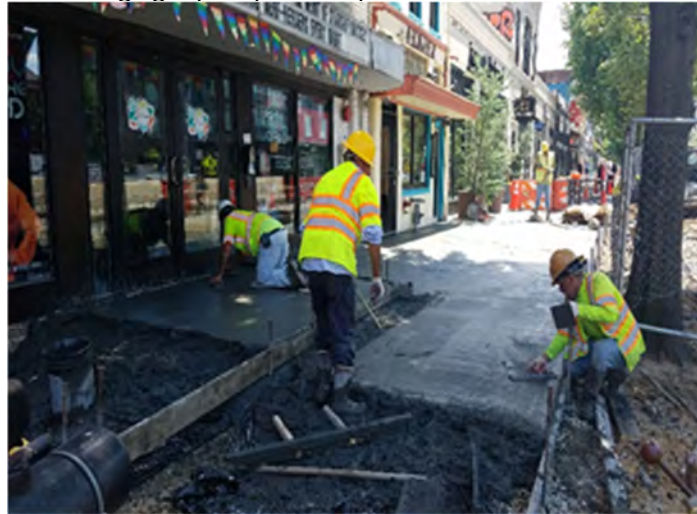
Omni framing light pole/pendant pole TS-16 and PVC installation
