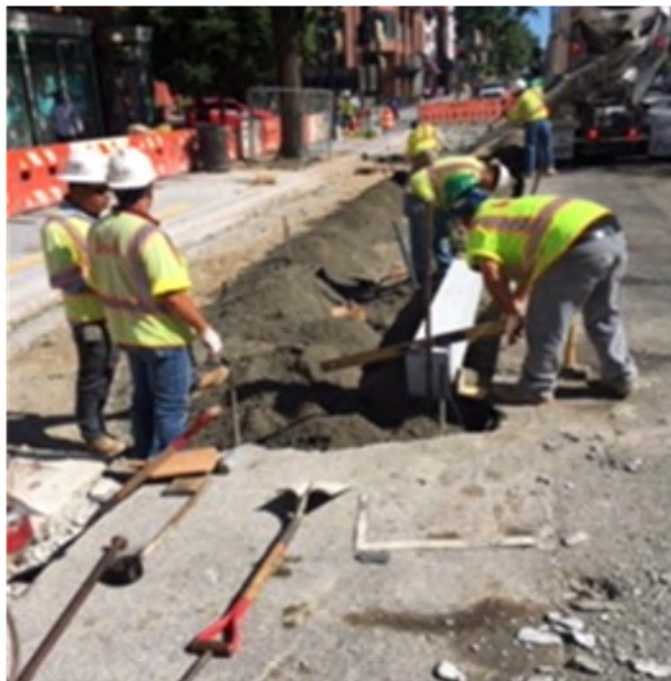
Granite Curb installation
