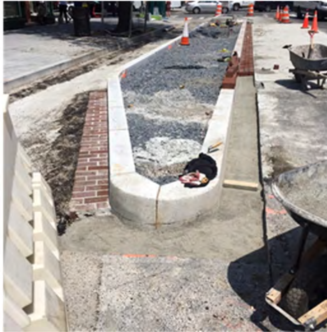
Brick gutter installation
