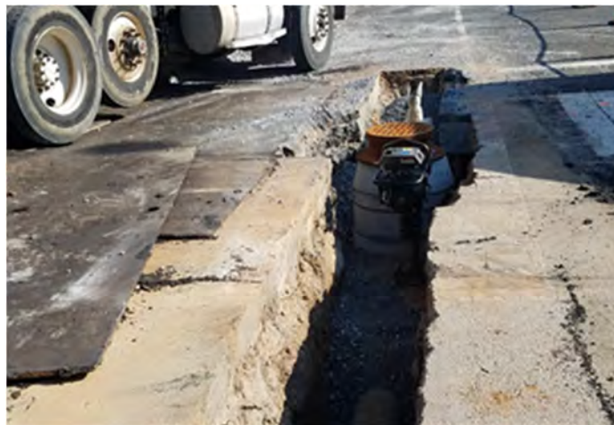
Valve casing at 12" gate valve installed by Omni Excavators
