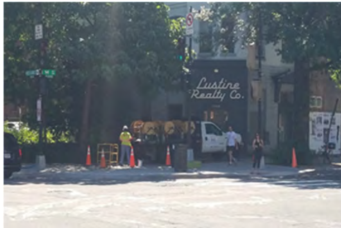
Completion of 7 conductor cable nearing completion.
