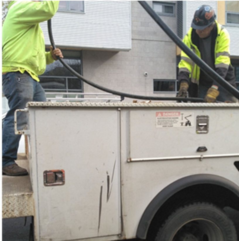
Pulling Comm Cable Florida avenue West side
