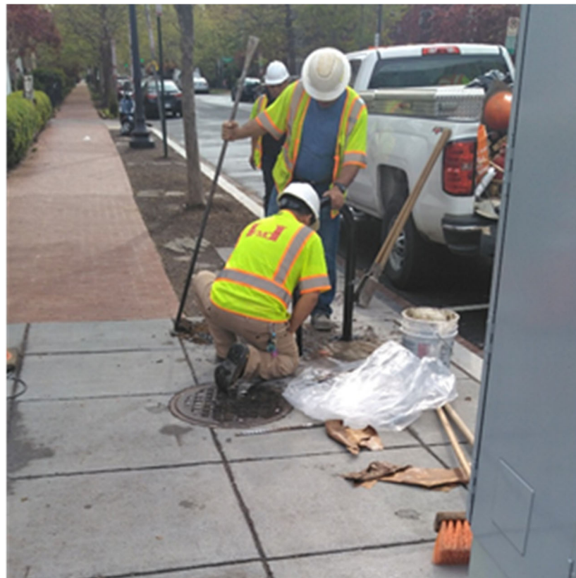
Installation of Bike Racks NEC Q street
