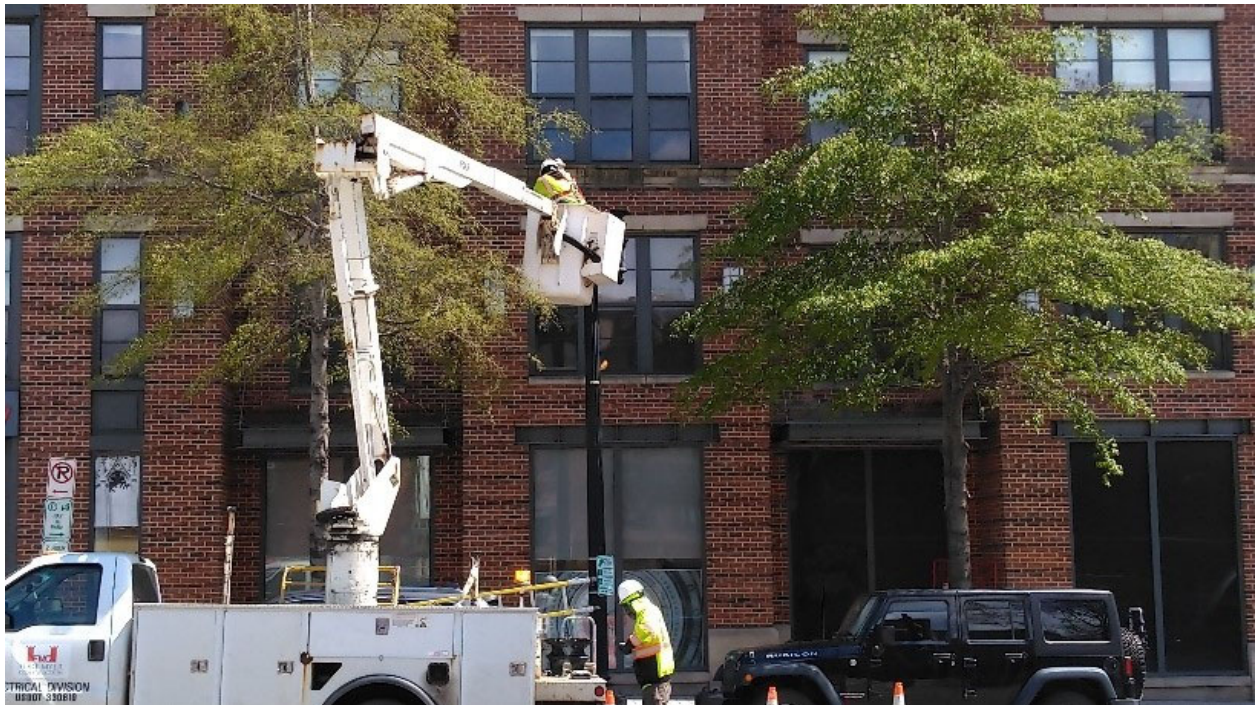
Electrician Swapping Light fixtures
