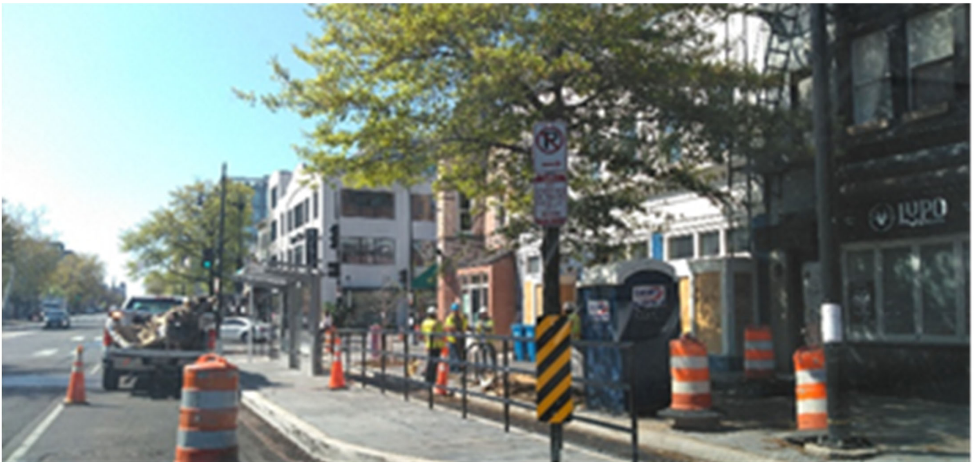
FMCC crew near T street installing missed Bike racks
