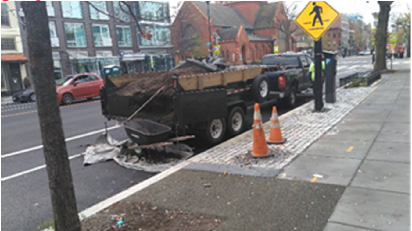
Cooper Placing Mulch near bio retention # 3
