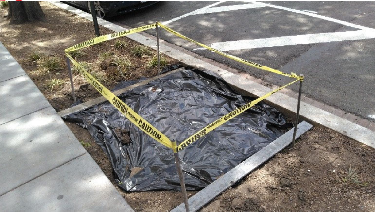
Areas prepared by DEN for concrete
