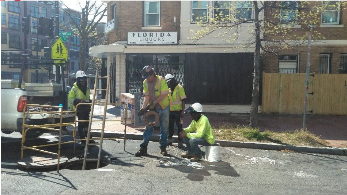
Electrical Crew at Florida, Pulling Comm Cable
