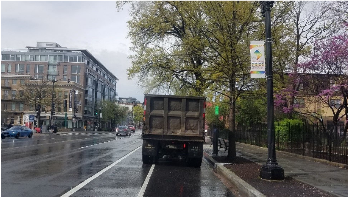
Cooper Enterprise was onsite placing mulch along the corridor
