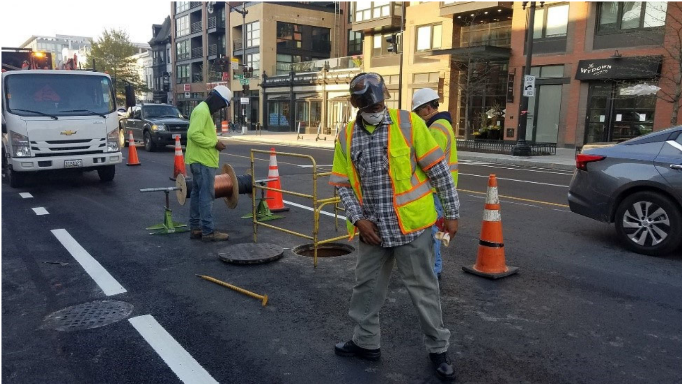
FMCC Electrical Crew on site working at Wallace Street
