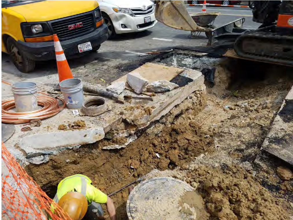
Insttation of New Water Service Line between R and S Street
