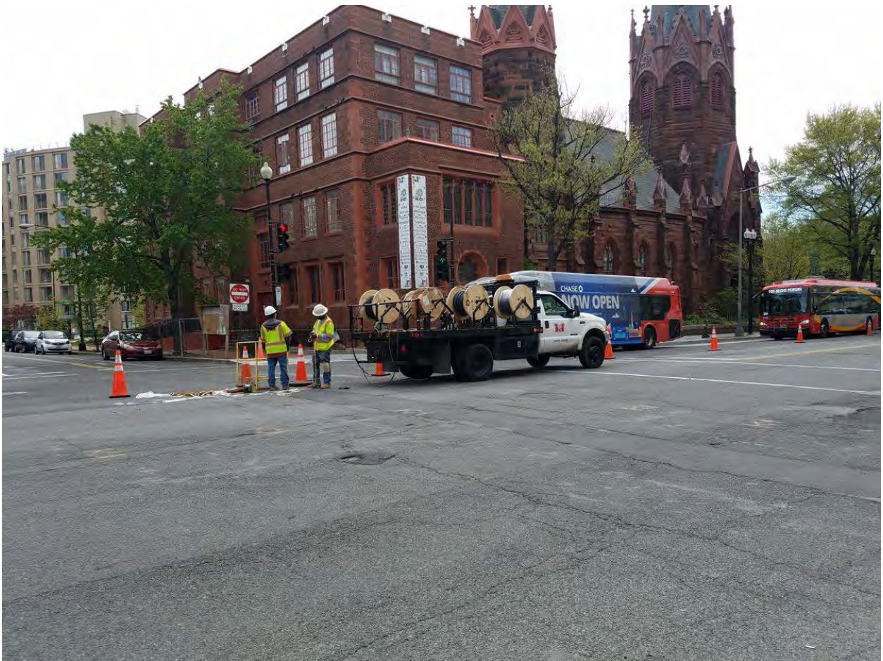
Installation of Traffic Signal Cables at 14 th and N Street
