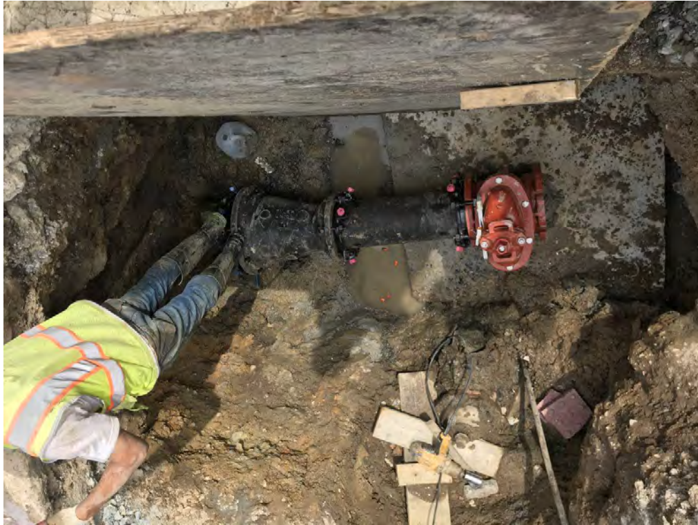
Installation of Gate Valve at 14 th and W for New Fire Hydrant
