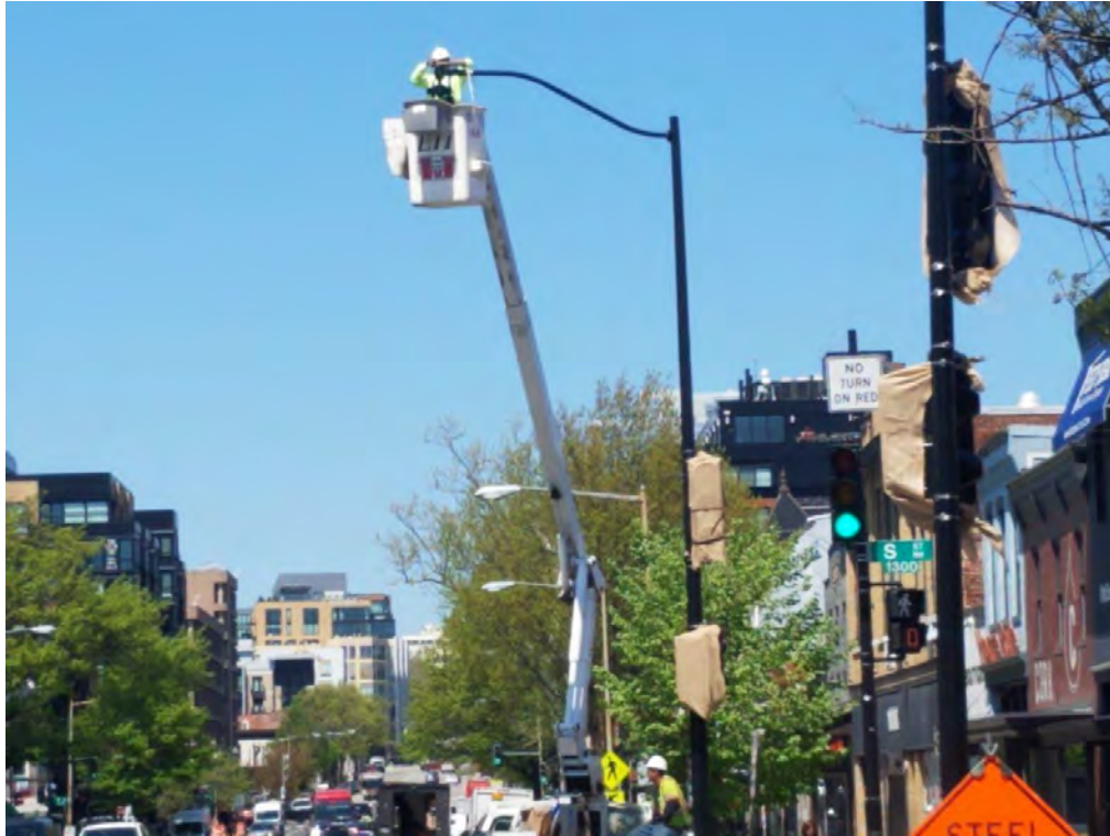
Installation of 150-Watt LED Luminaire on Pendant pole
