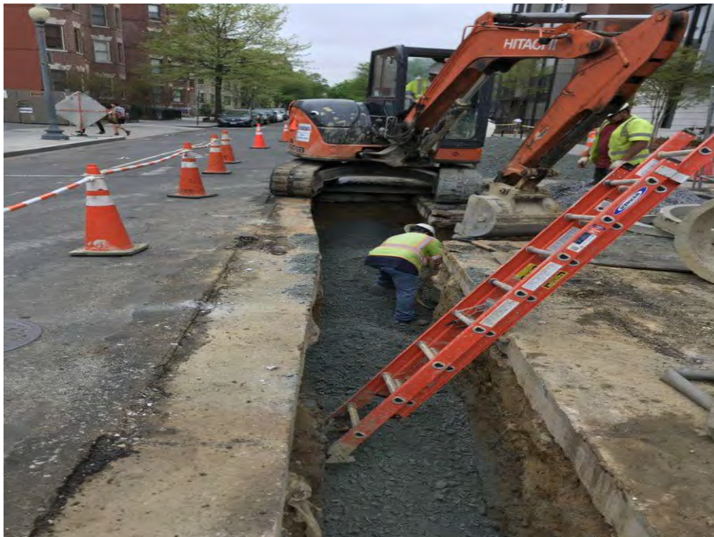
Installation of Gate Valve at 14 th and W for New Fire Hydrant
