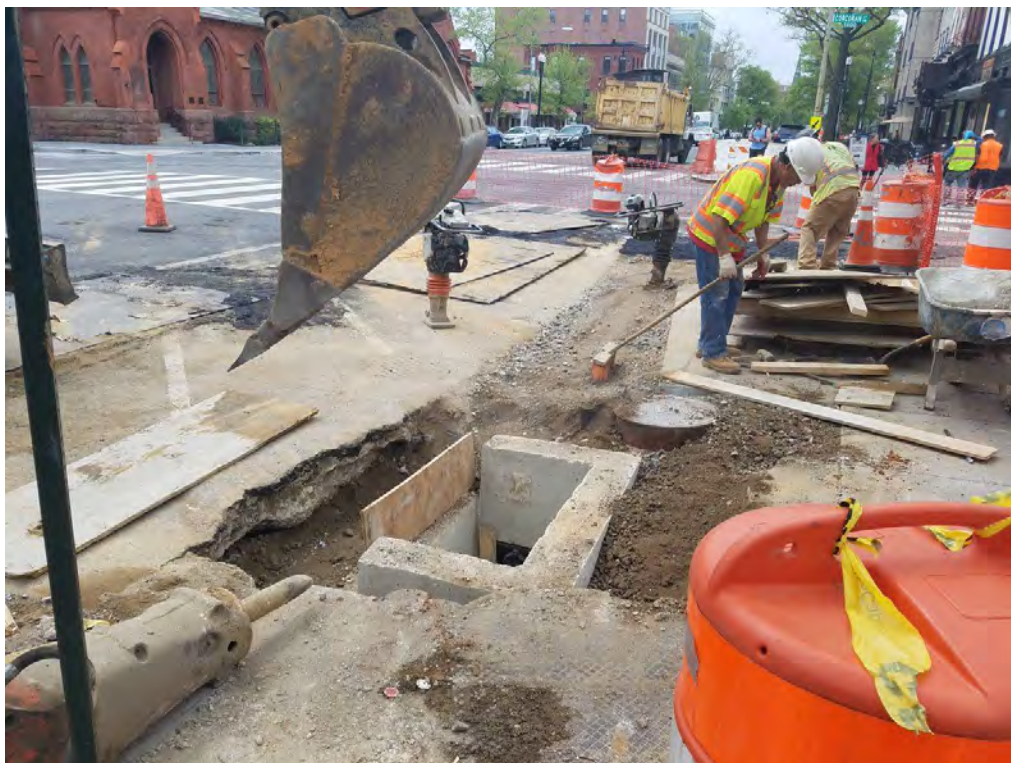
Backfilling Connection Pipe and Catch Basin (CB-15)
