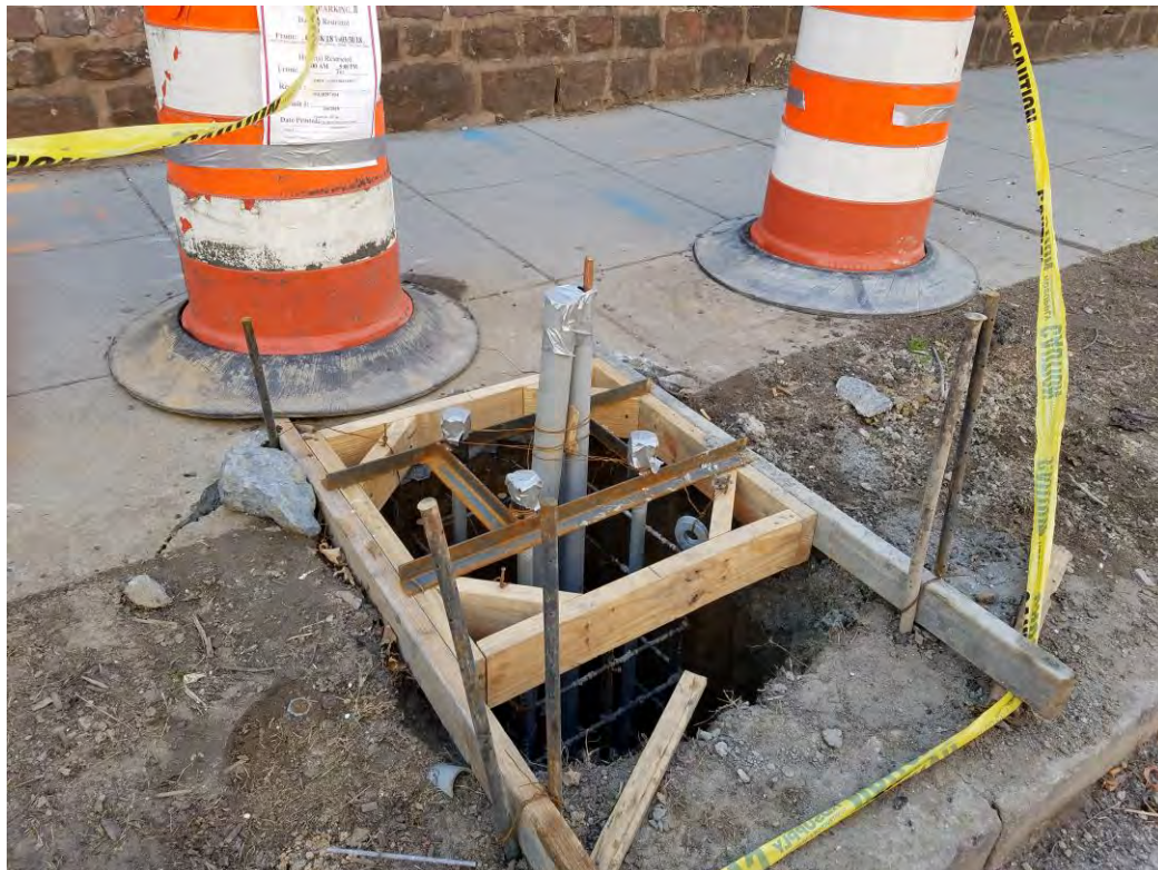
Forming of Streetlight Foundation
