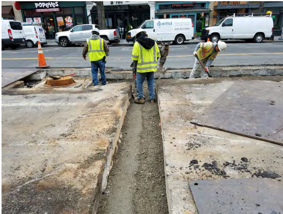
Contractor compacting Backfill Material Between N Street and Rhode Island Ave
