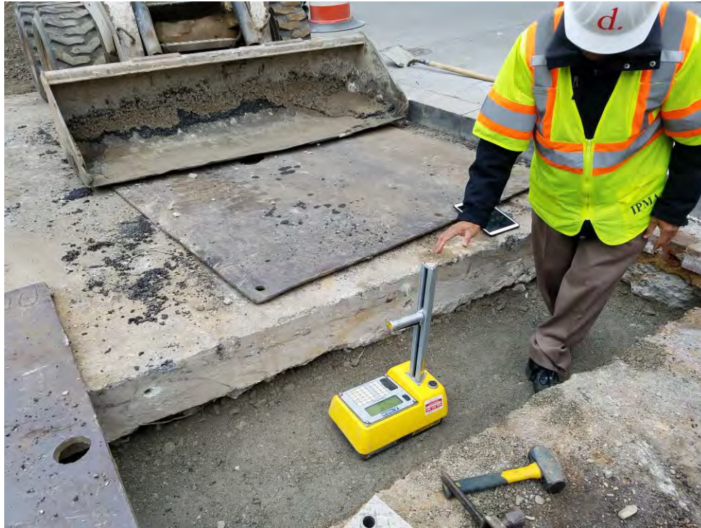
QA/QC taking compaction Test on Aggregate Base Material
