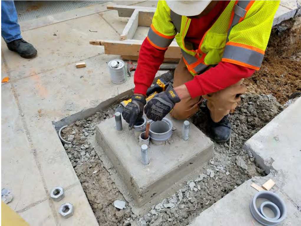
Installation of Ground Rod and Conduit Rings
