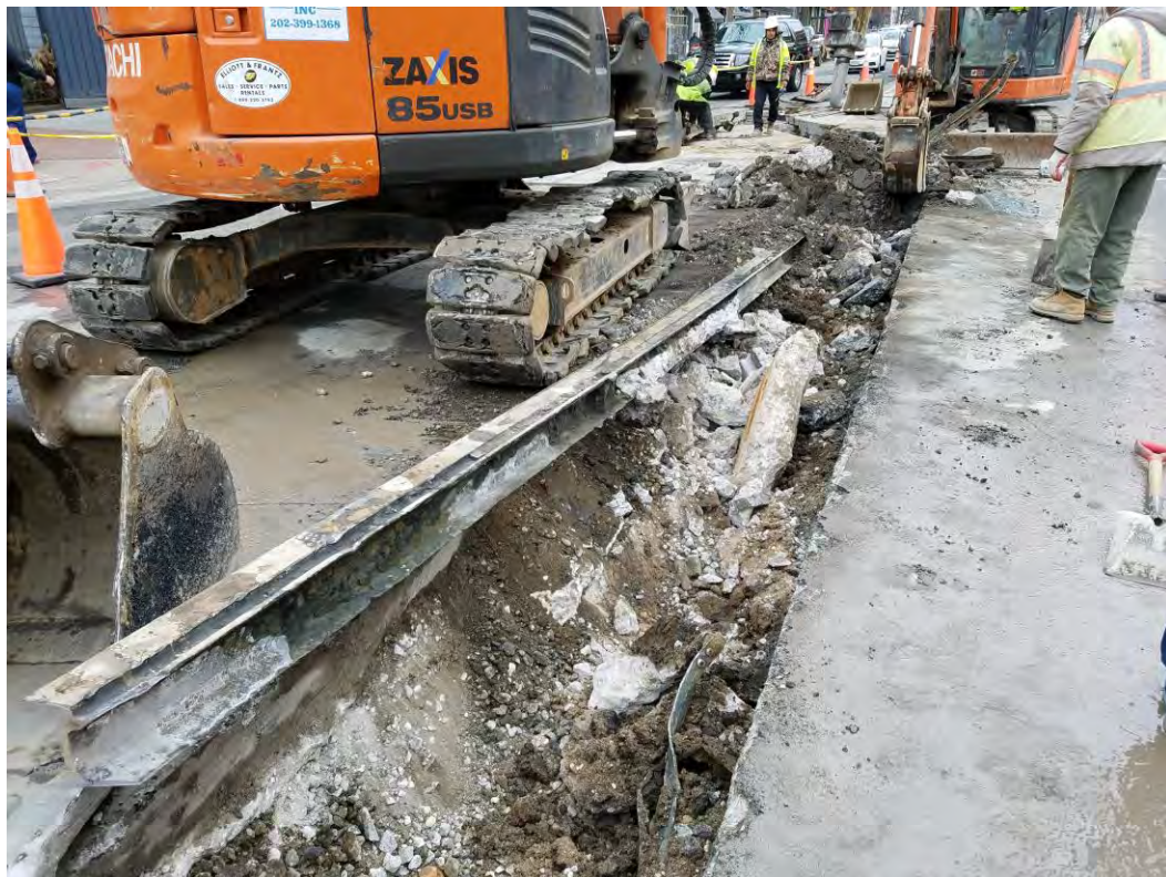
Removal of Old Streetcar Rail
