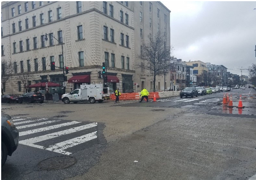
DCWater crew onsite testing existing 48" water main at 14 th & R St
