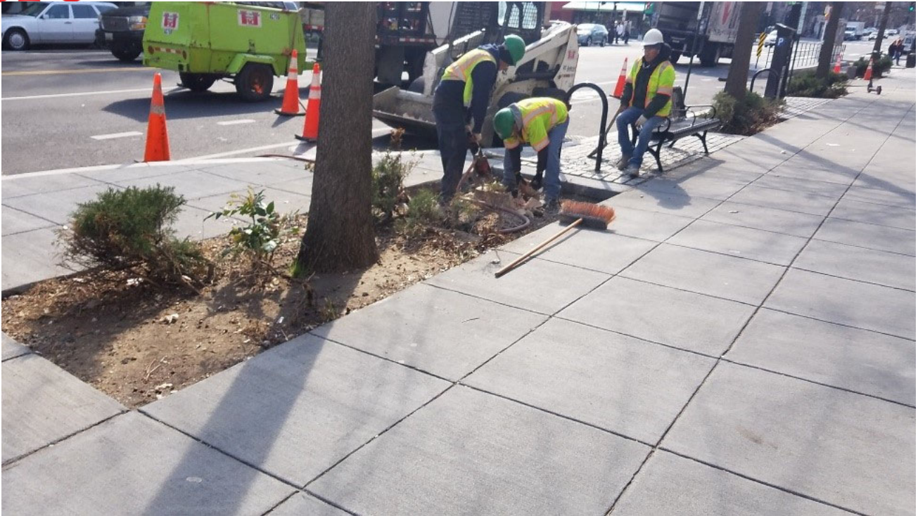
Drilling and removal of the streetlight foundation
