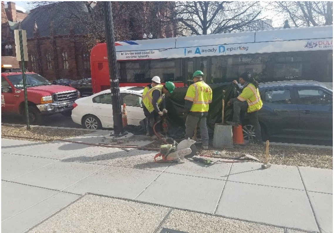
FMCC civil crew removing transformer bases
