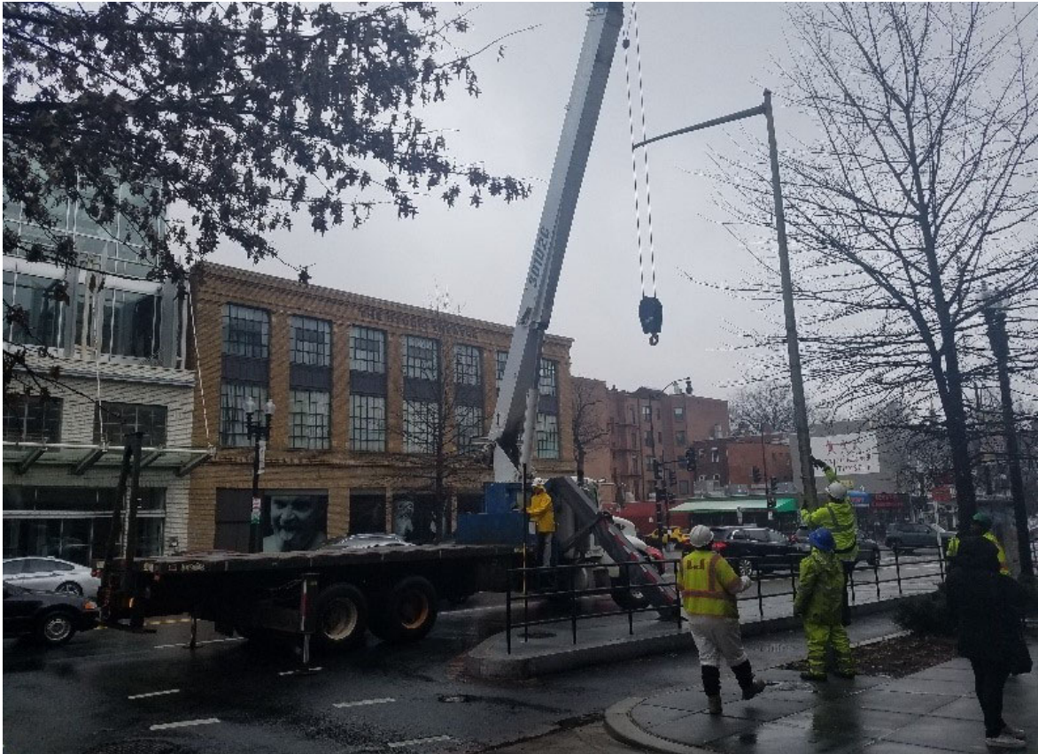
FMCC Boom truck used to remove existing pendant pole
