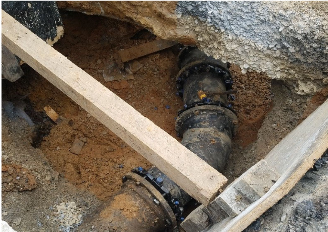
45° bend connected to 12" D.I.P.
