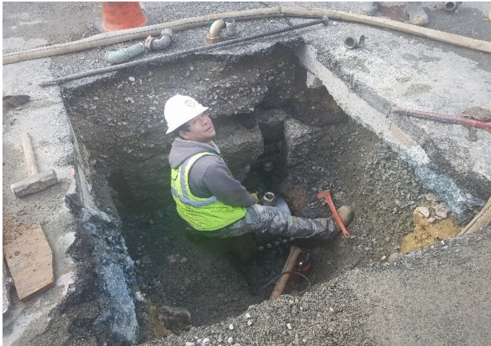
Collar used to repair existing main
