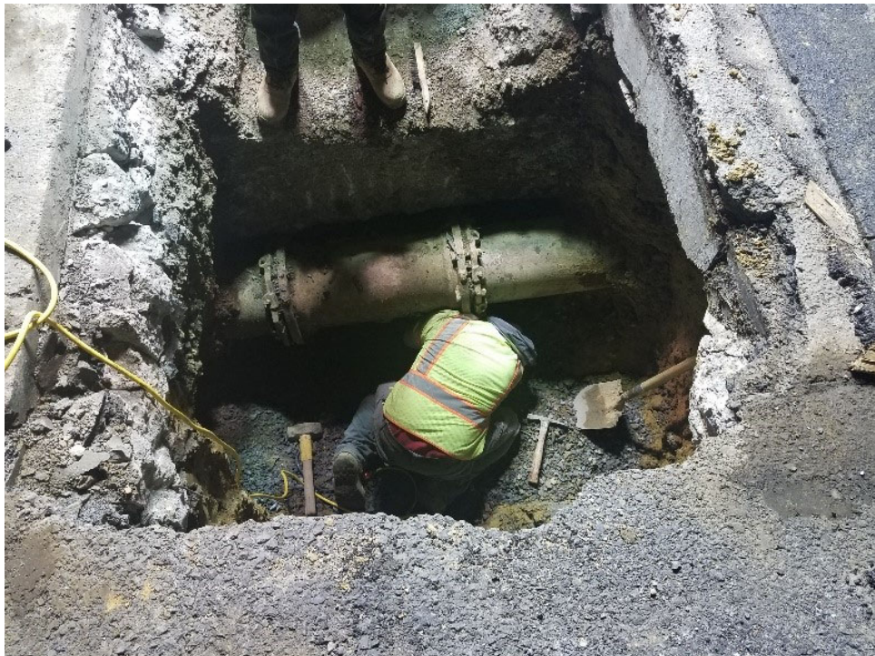
Connection to 6" hydrant underway
