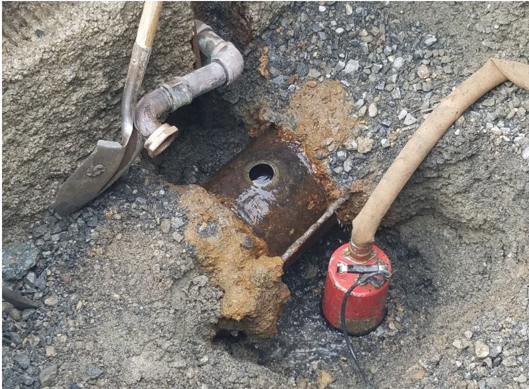
Water pump used to remove water from trench
