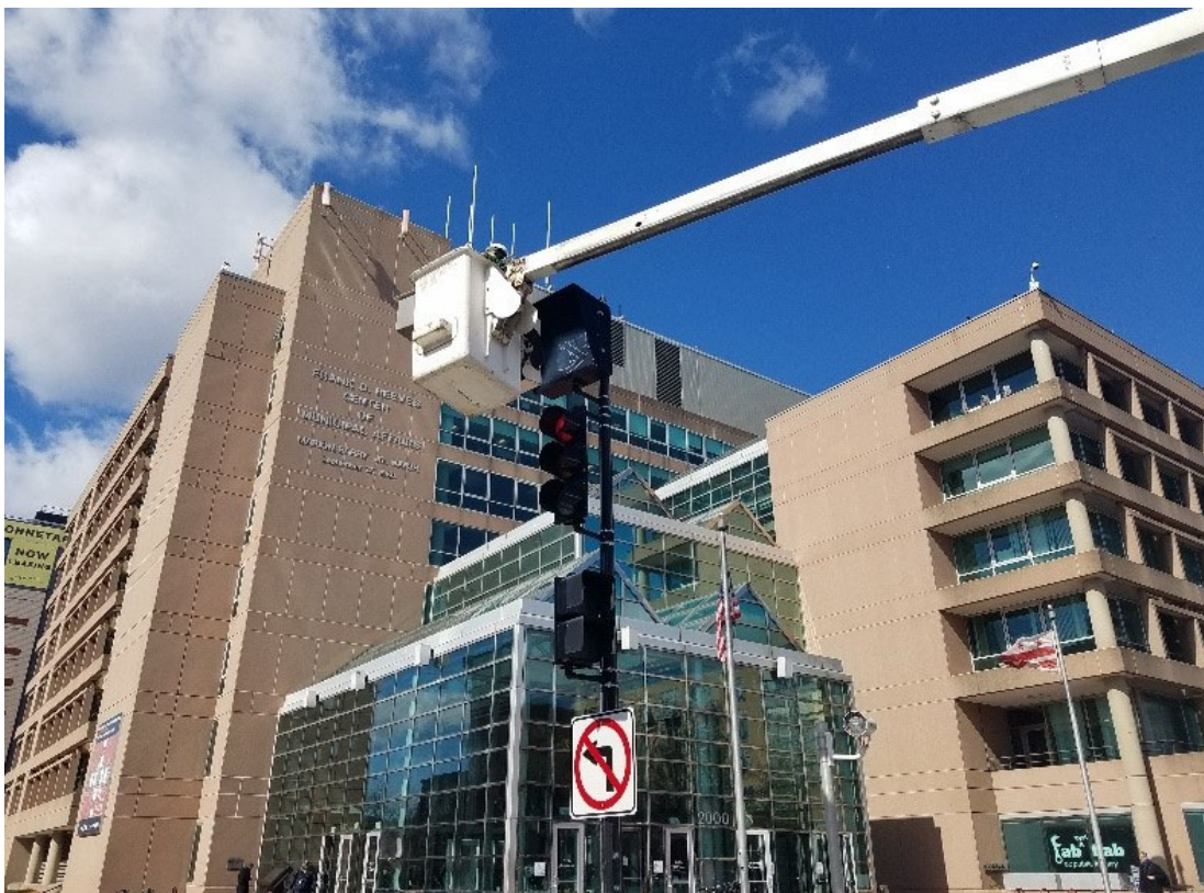
FMCC Electrical crew installing No Left turn LED signal at TS-38.
