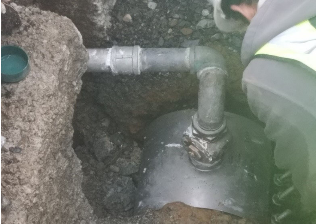
Connections repaired at 12" main by Omni
