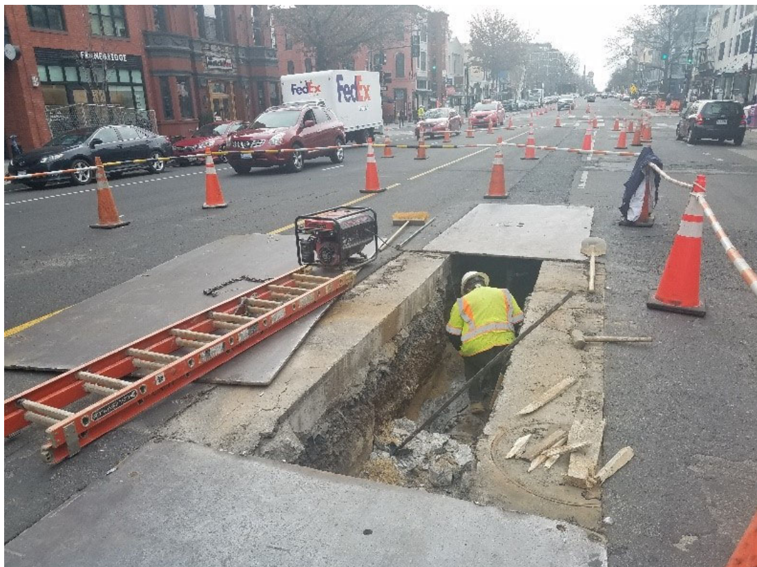
Water pump used to remove water from trench
