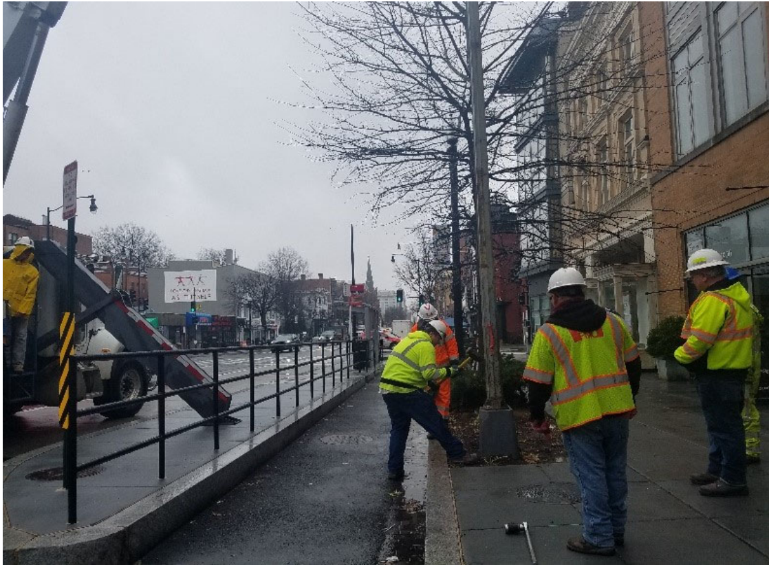
Poles unbolted from transformer before removal
