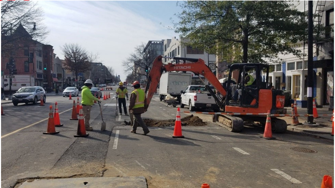
Excavating at NWC of T Street for the water service line
