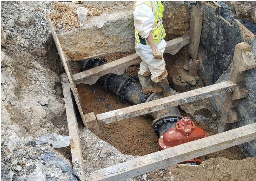
12" ductile iron pipe installed including gate valve
