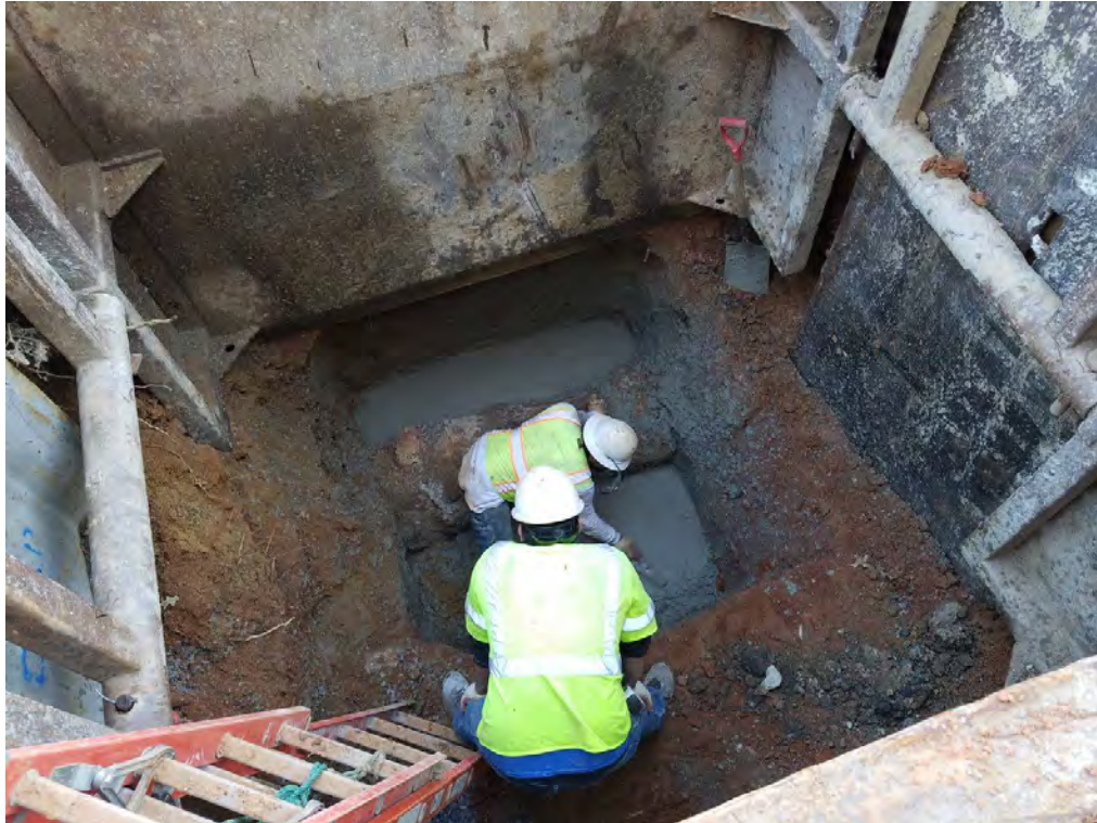
Placement of PCC base for Brick Combine Sewer Manhole
