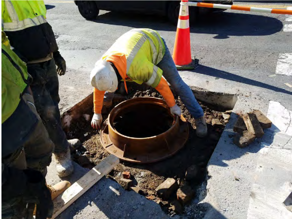
Replacement of Frame and Cover of Old Traffic Signal Manhole (EM03)
