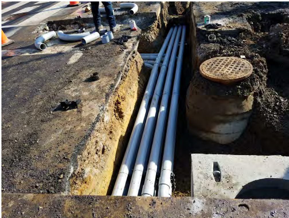
Installation of 4" PVC Conduit between MH66 to MH68 on T Street
