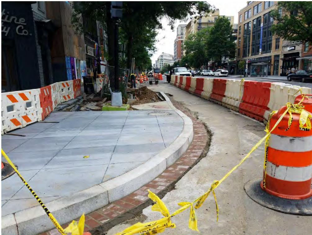
*Installation of Granite Curb and Brick Gutter at the SE corner of Rhode Island Ave*
