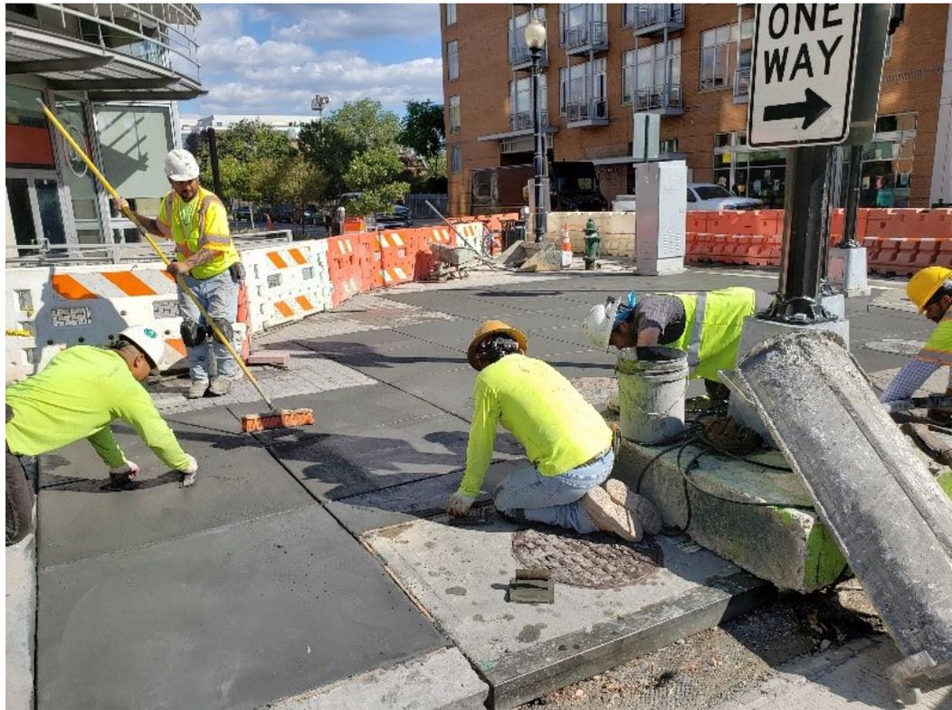
DEN crew placed PCC Sidewalk with Class F Concrete, 3500 PSI as well as Class E for WC Ramps at V & 14th St. NW. Crosswalk-NEC.
