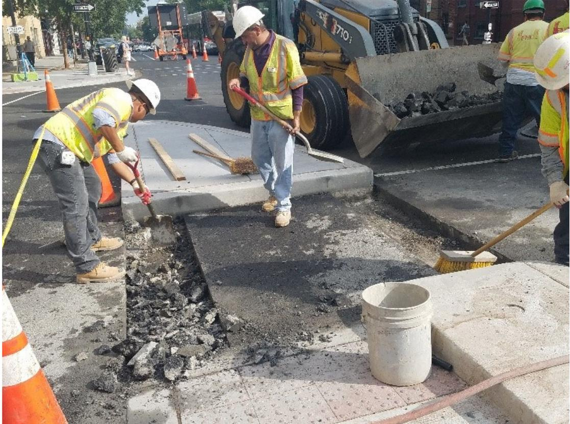
FMCC working at SWC of 14th & N St installing truncated dome surfaces.
