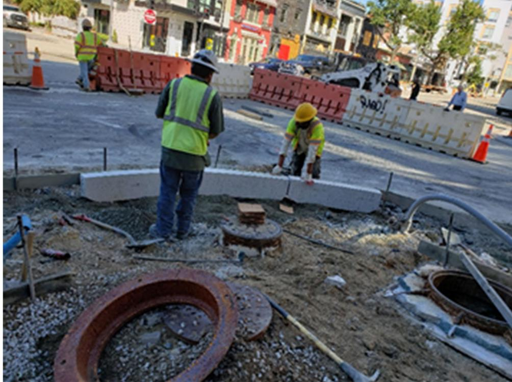
DEN crew installed Straight and Curved Granite as well as they also adjusted 3 Utility Manholes at Sidewalk at W St. & 14th St. Intersection at CVS Store, on Wed. 9-25-2019.
