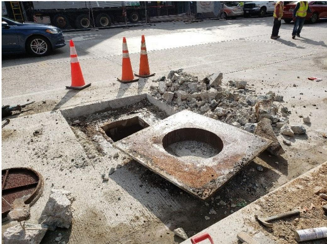
Left Picture: Capitol Paving Inc. crew saw cut and installed a new PEPCO Manhole near 2216 Block 14th St. to power new Signal Lights at Florida Ave. & 14th St. Intersection.
