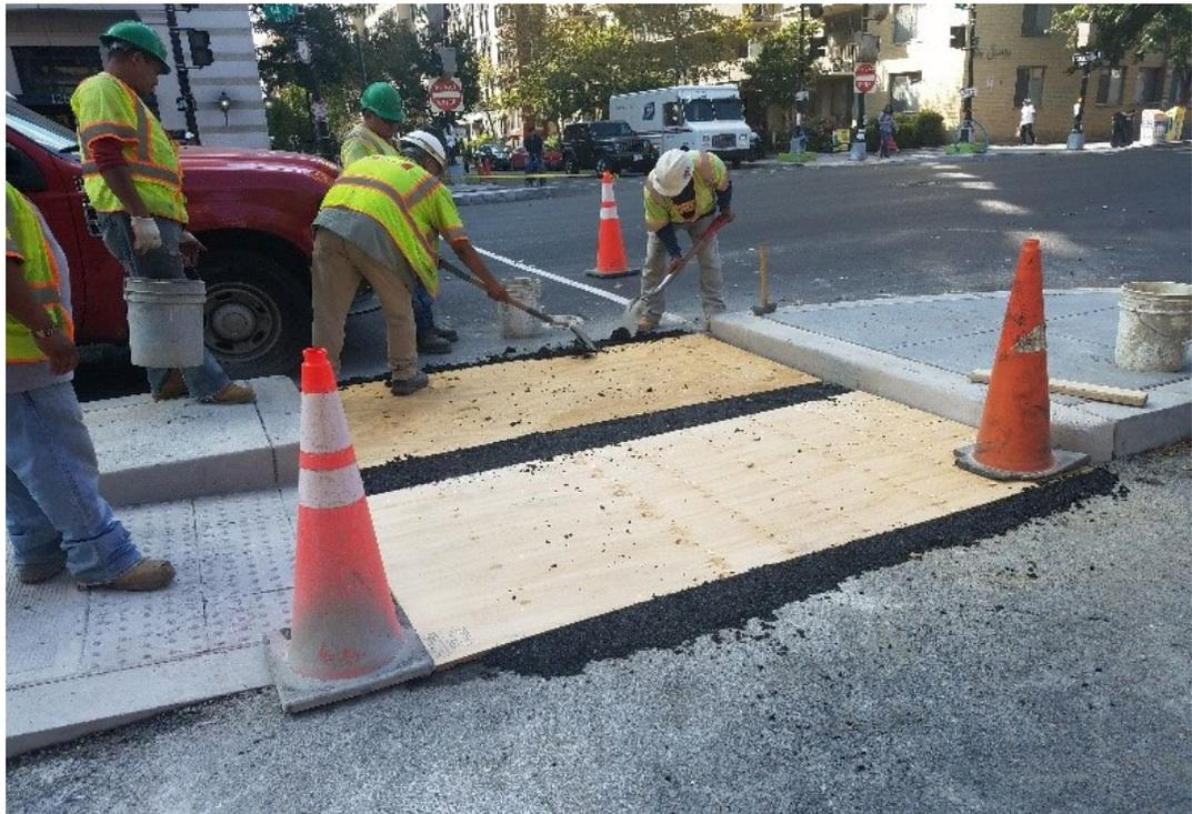
SEC of 14<sup>th</sup> & N St warning surface completed and covered temporarily during concrete curing.
