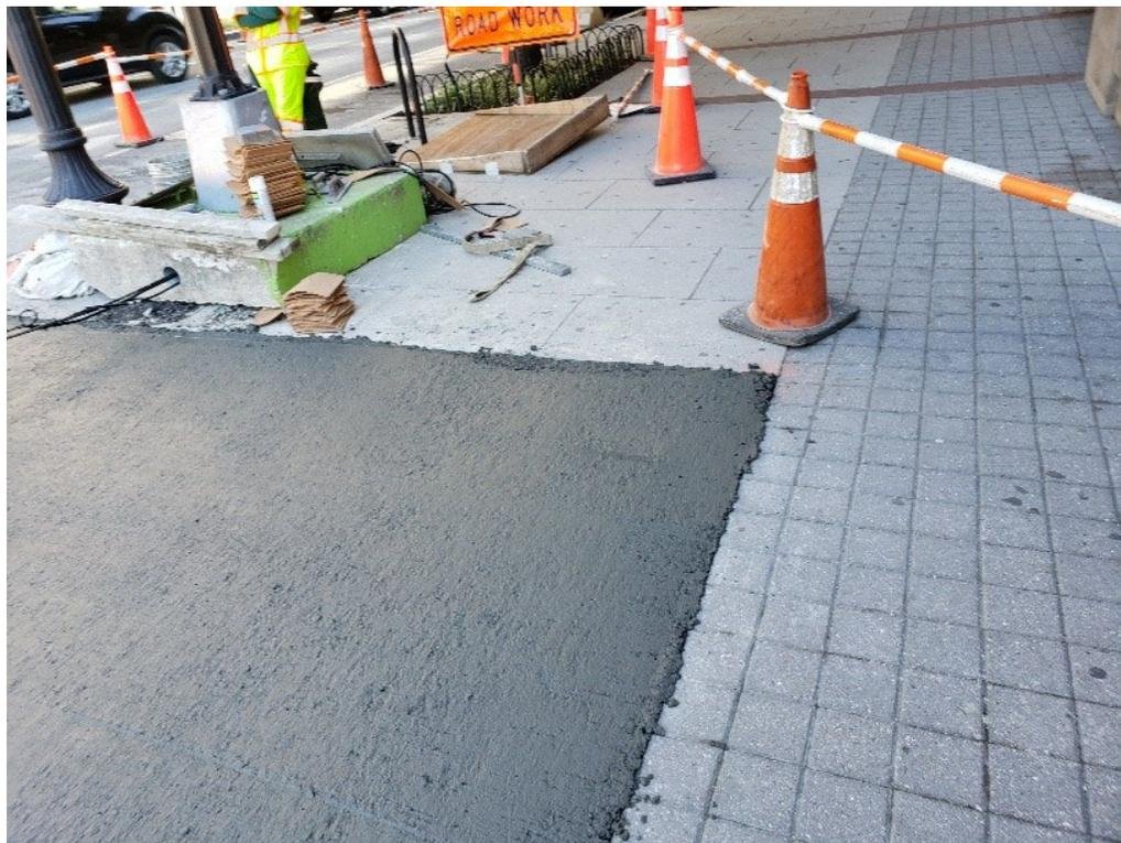
DEN excavated and removed old PCC Sidewalk plus damaged brick pavers then placed new PCC sidewalk with Class F, DC-DoT Concrete, 3500PSI .
