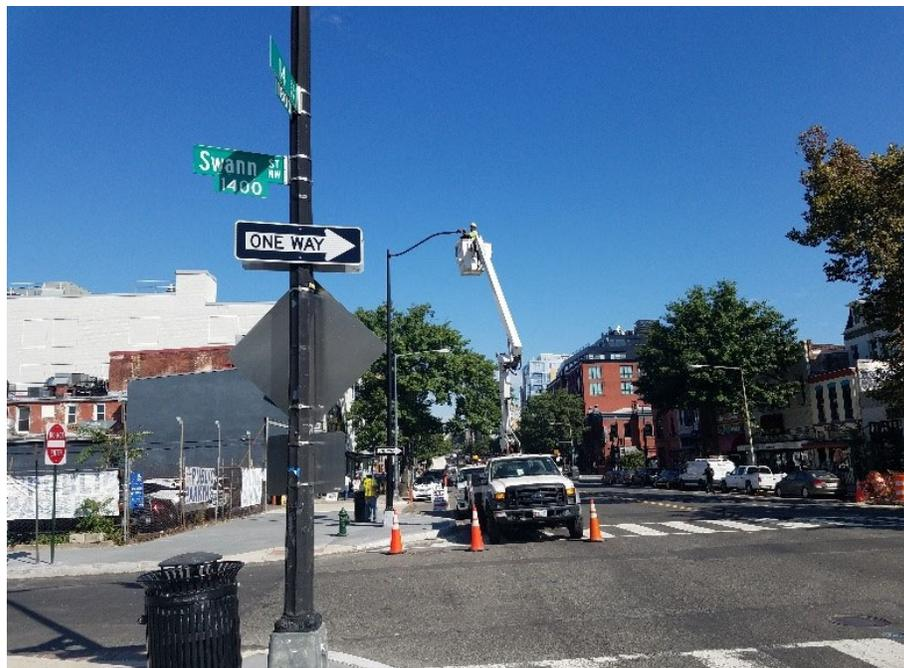
FMCC electrical crew installed 150W teardrop fixture at NWC of 14th & Swann St
