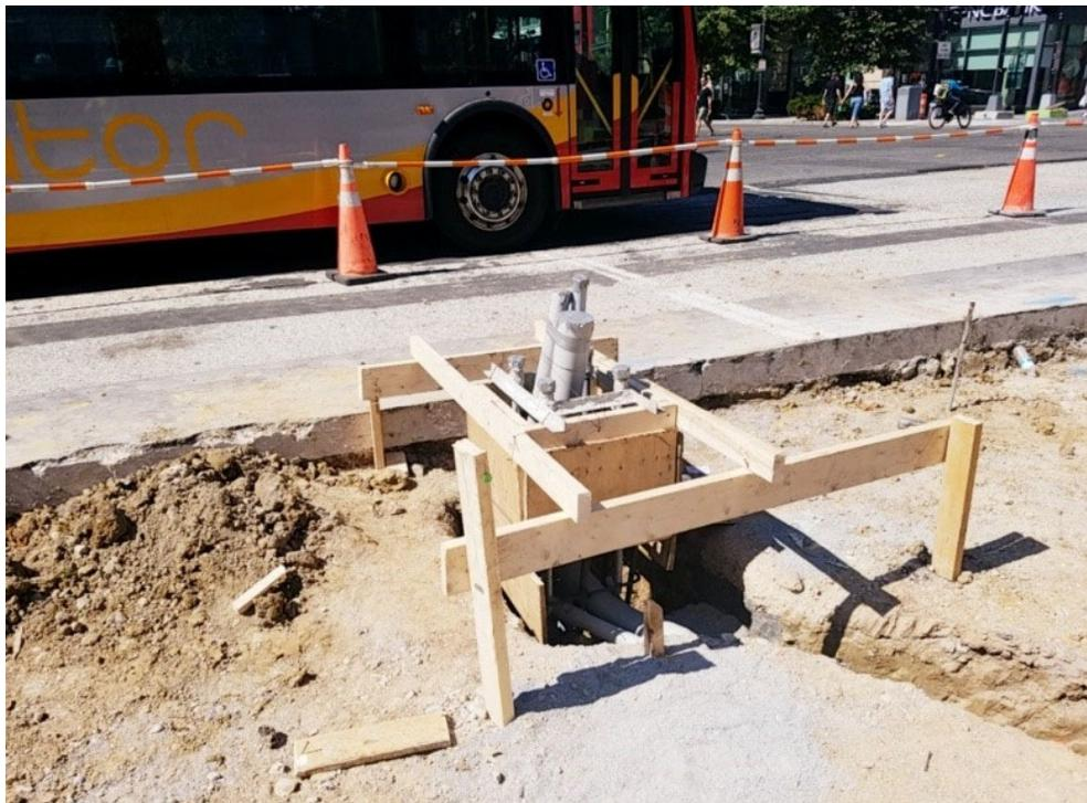
TS13 foundation formed and ready for concrete placement
