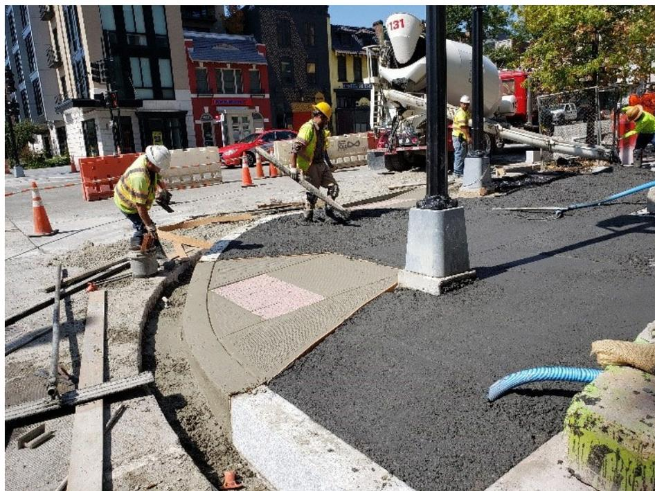
D.E.N crew poured 2 wheel Chair Ramps ; DEN crew poured Class F for PCC Sidewalk at NEC W & 14th Sts.
