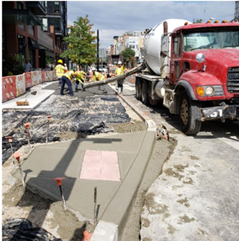
DEN crew placed PCC Sidewalk with DC-DoT Class F Concrete, 3500 PSI as well as Class E for WC Ramps at Wallach Place & 14th St. NW
