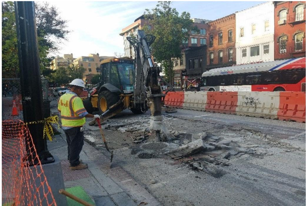
Demolition at SEC of 14th & P St for directional bus island
