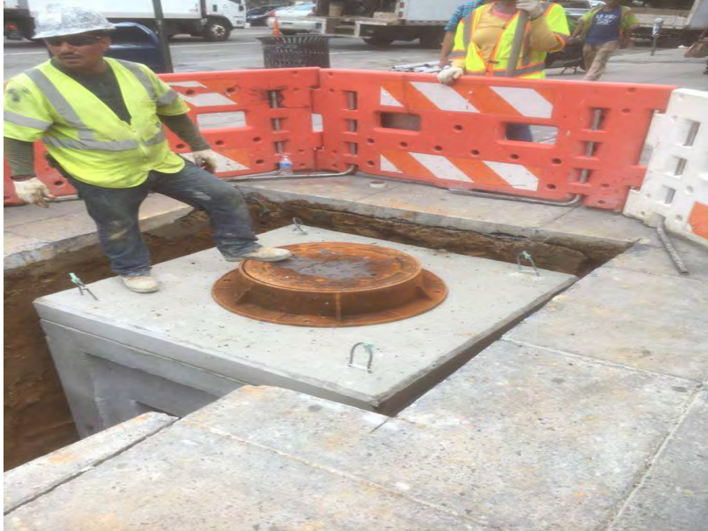
Installation of Manhole at the NW corner of P Street
