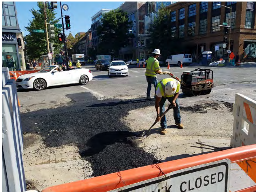
Placement of Temporary Asphalt over Electrical Trench
