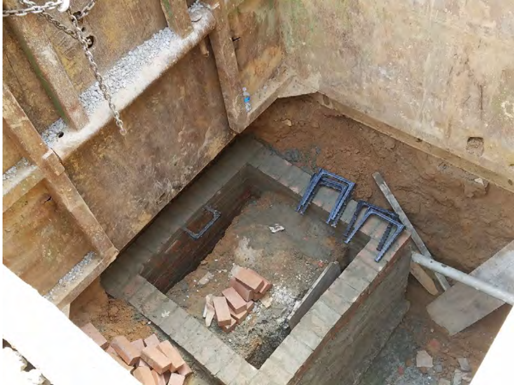
Construction of Brick Combine Sewer Manhole
