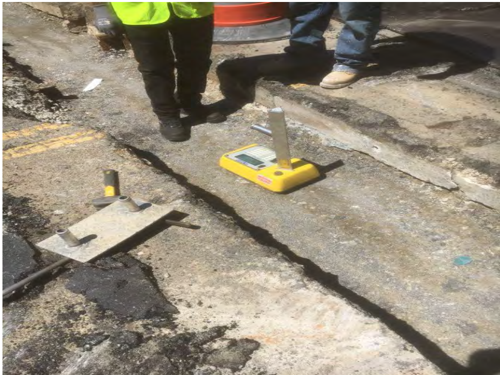
Density Testing of Aggregate Base Material prior to PCC Base placement
