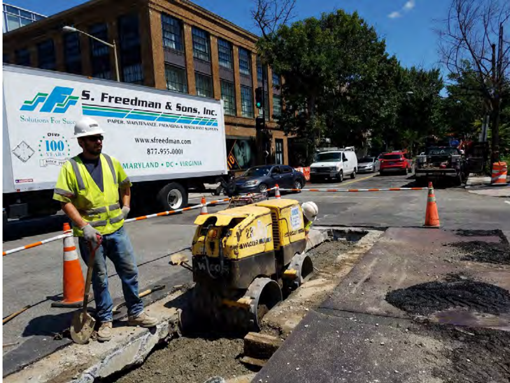
Compaction of Conduit Trench on P Street Westside
