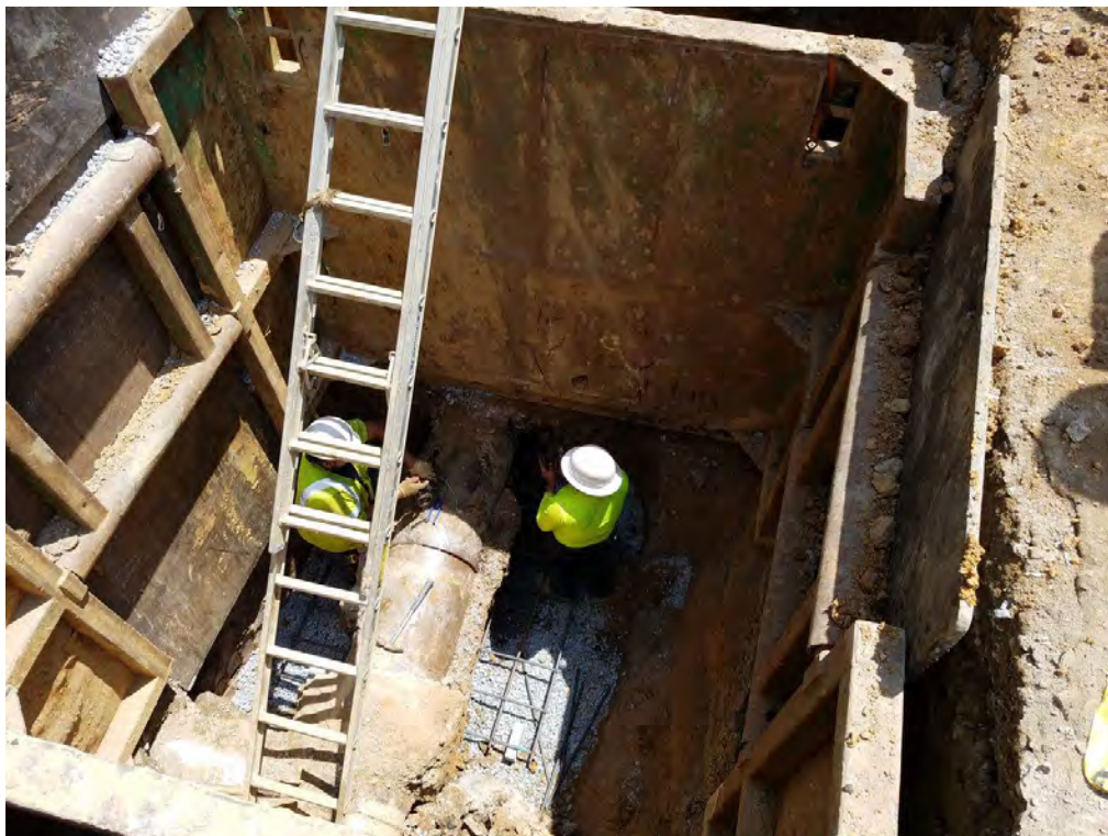
Placement of #57 stone and #5 rebar for Foundation Mat of MH-07
