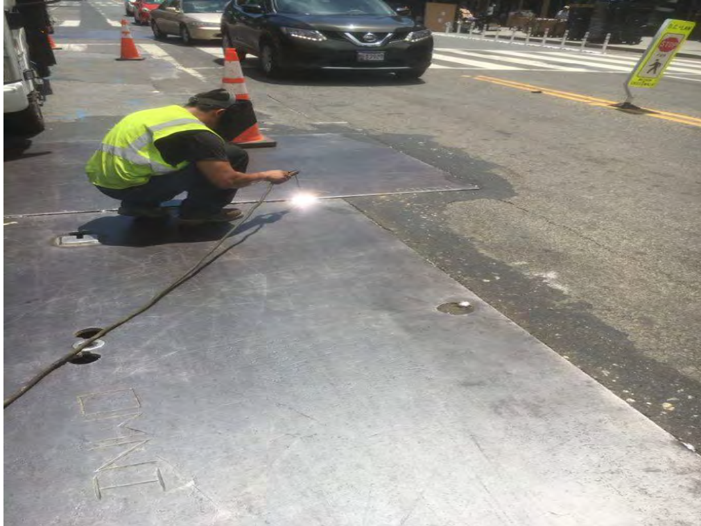
Rewelding Steel Plates between Wallach and U Street
