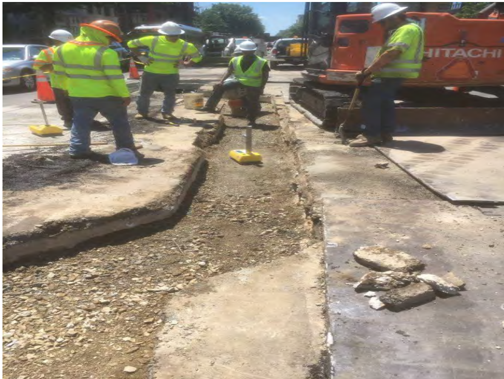
Compaction Testing of Aggregate Base Material between Wallach and U Street
