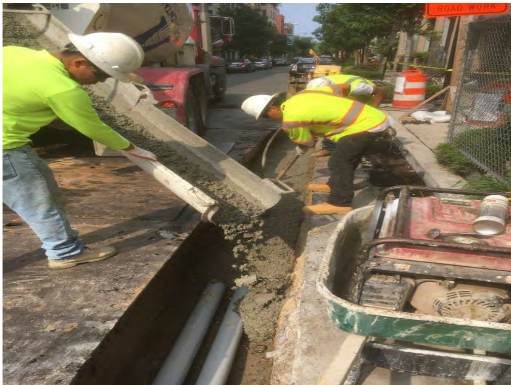
Encasement of PVC Conduit on Church Street
