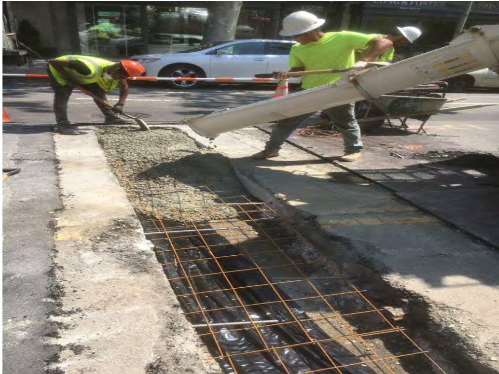
Pouring Class E Concrete for PCC Base over Laterals
