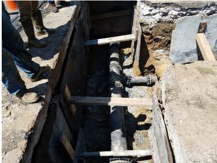
12"x6" Tee connection completed.
