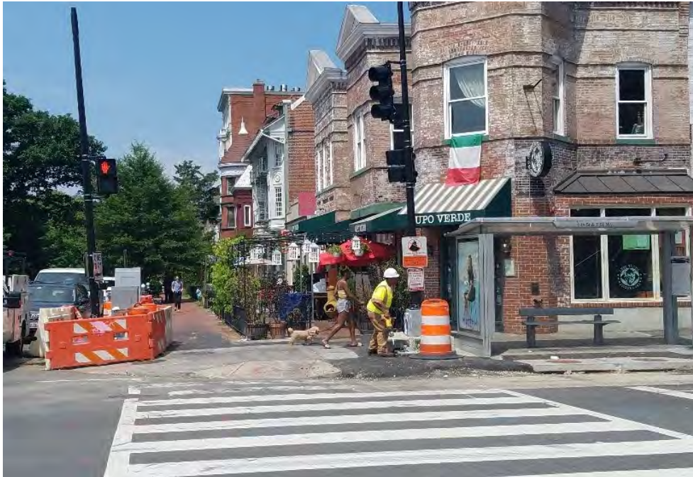
Signal pole to be installed at NWC of 14 th & T St.
