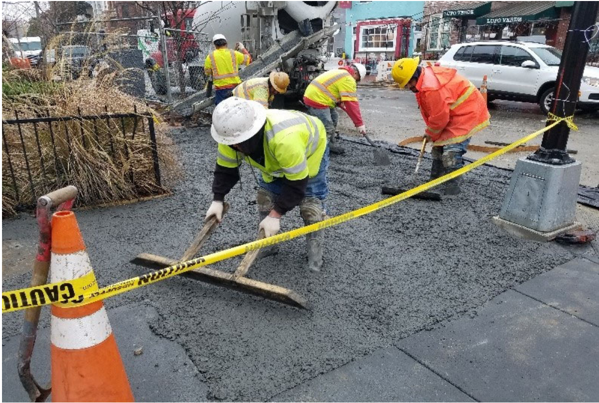
FMCC installing 3 section at L92/TS/PP
