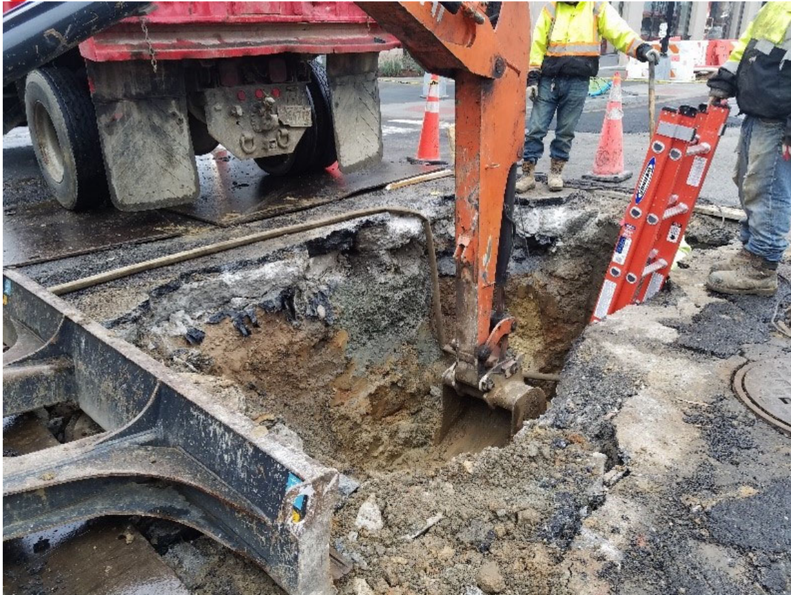
Omni excavating and exposing main at NEC of 14 th & R St
