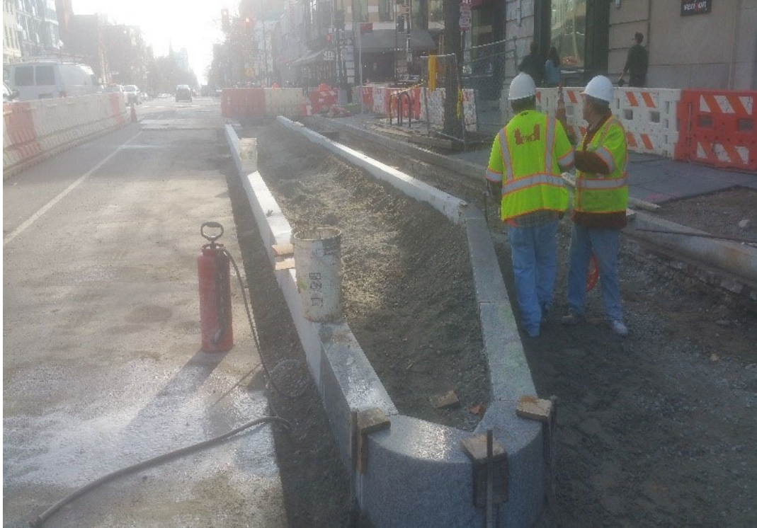
Granite curb placement completed for the day by FMCC
