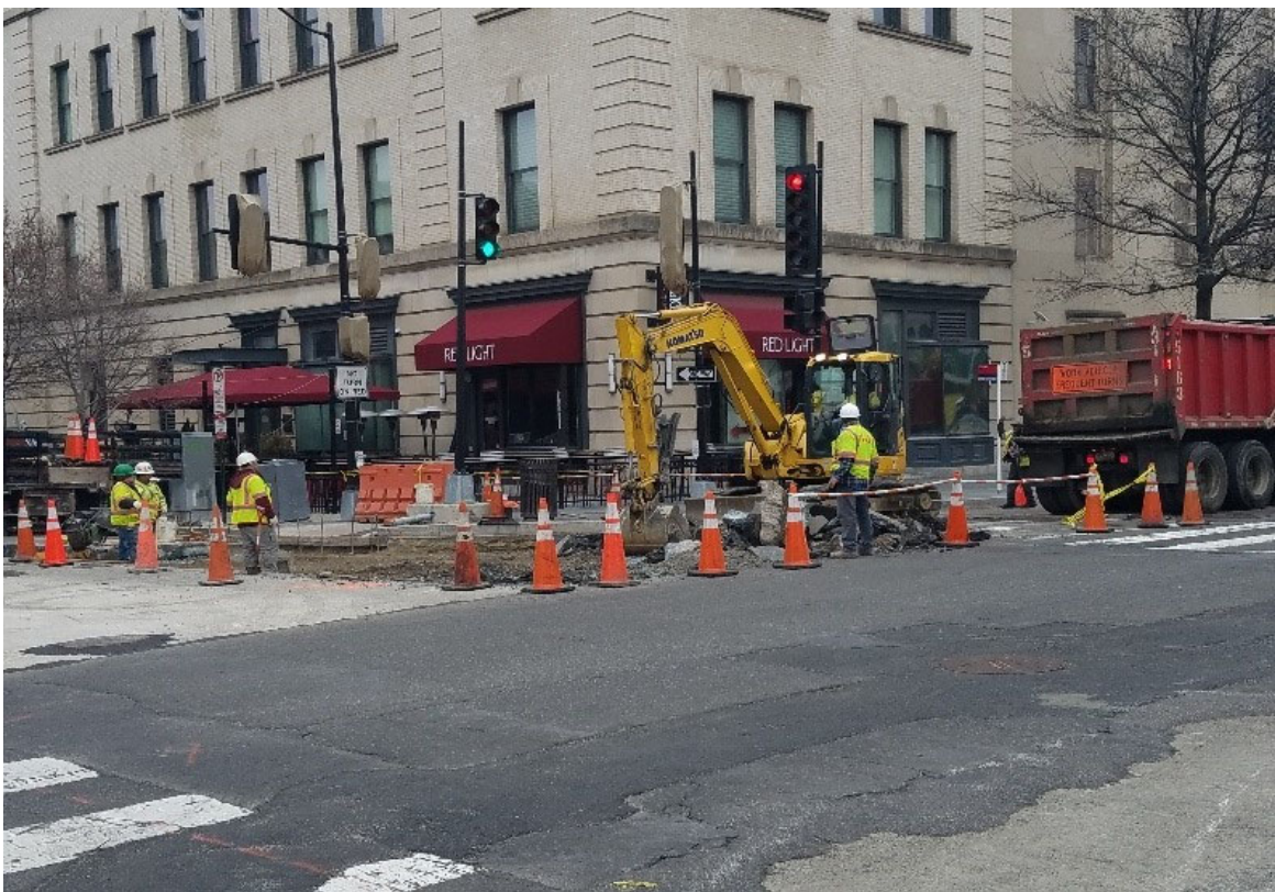
FMCC demolishing full depth roadway at NWC of 14 th & R St
