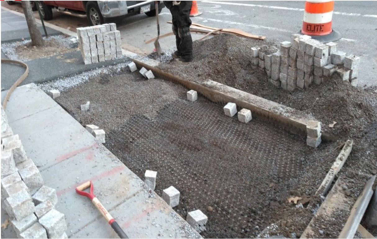
DEN installing the GEO GRID at 1925 14 th Street NW
