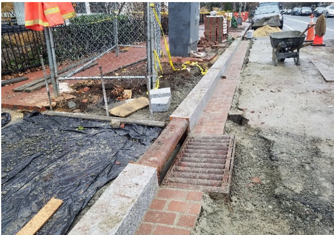
inlet drain at SWC of 14 th & T St
