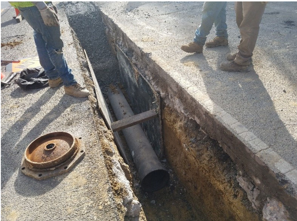
Omni 12" pipe installation completed for the day.
