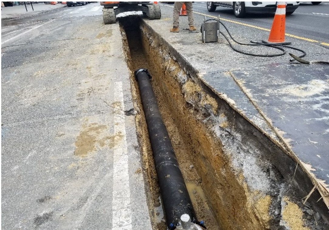
3 20' sections of 12" ductile iron pipe placed by Omni
