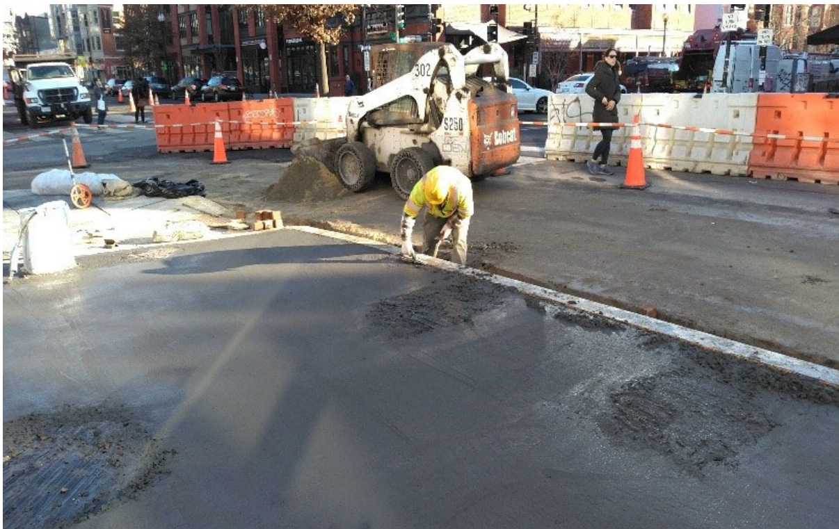
DEN starting to finish the 4" PCC Sidewalk at the SW corner of T Street & 14 th Street NW
