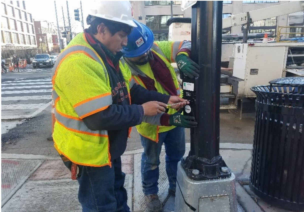
FMCC repairing push button on R St
