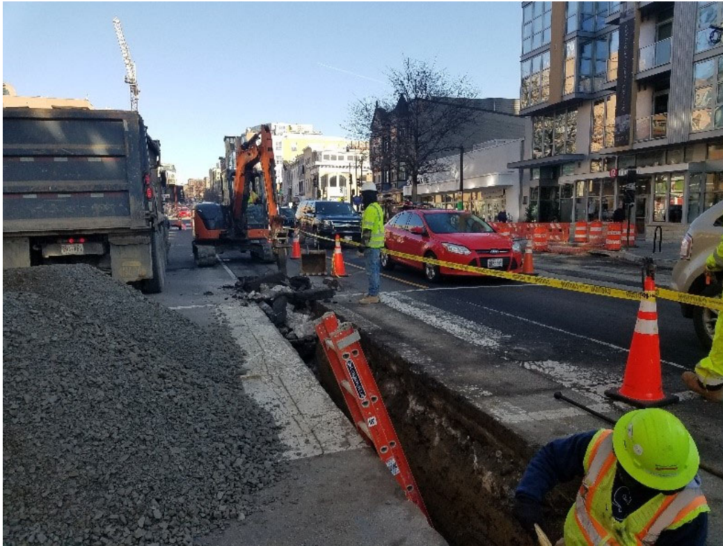
Omni near Wallach St installing 12" D.I.P. for new water main location
