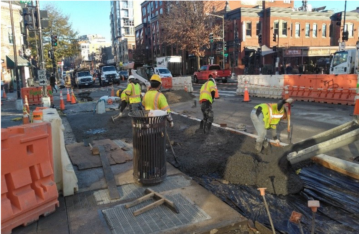
Den poring the 4" PCC Sidewalk at T Street & 14 th Street NW
