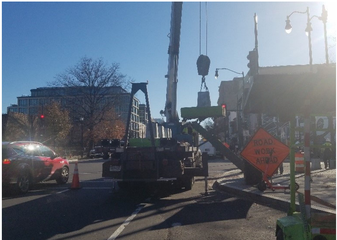
Tbases loaded via boom truck by FMCC
