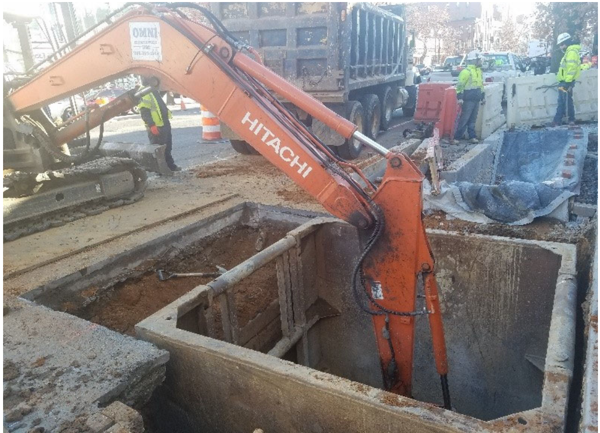
Trench box placed at 1624 14 th St sewer manhole
