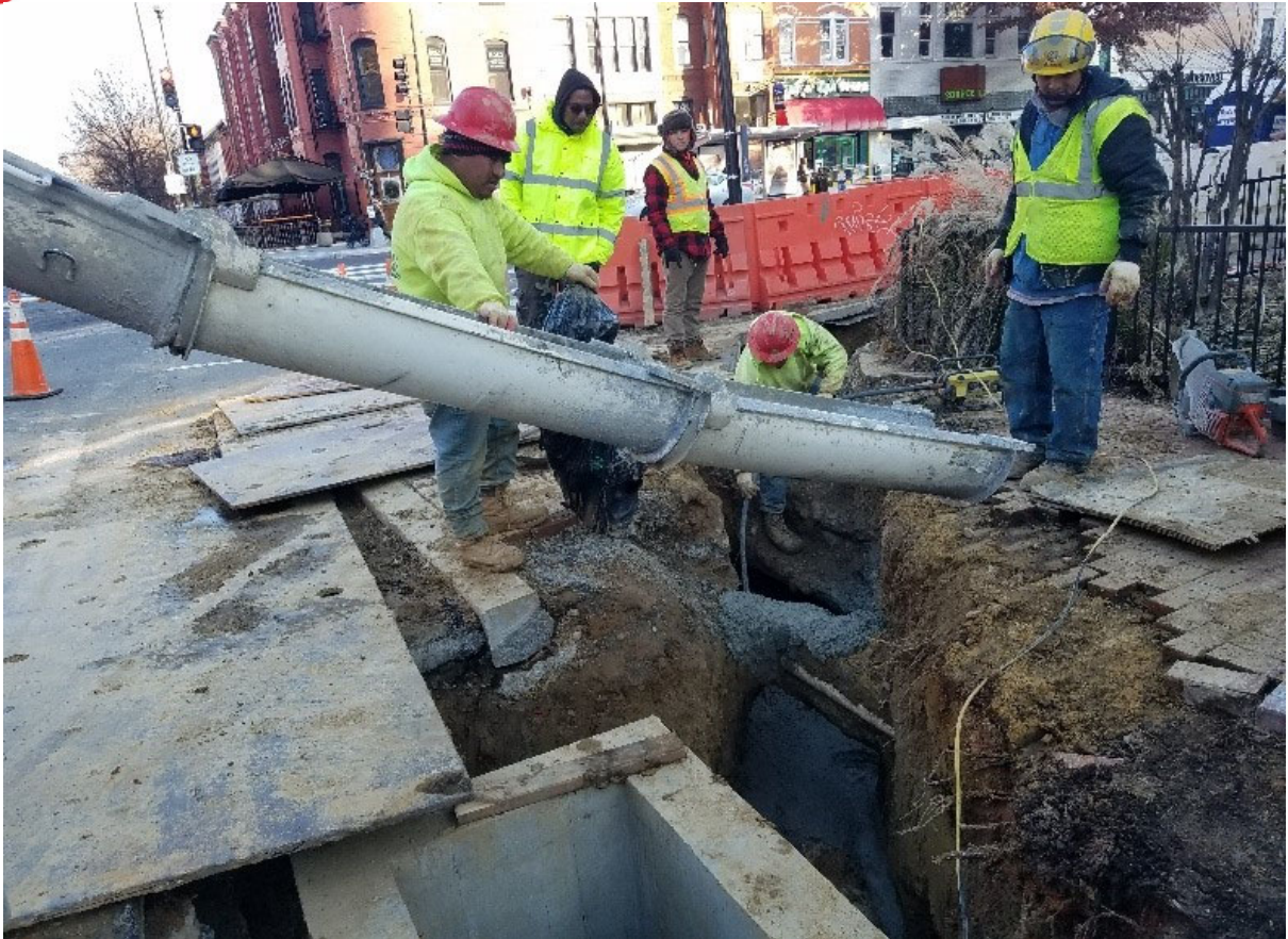
DCWater class concrete placed at connect pipe.
