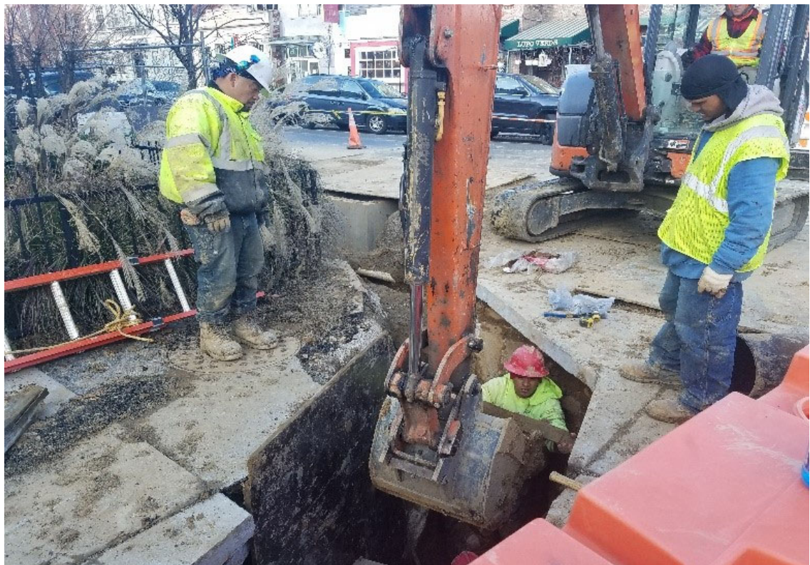
Omni installing 12" ductile pipe at CB-25 at T St
