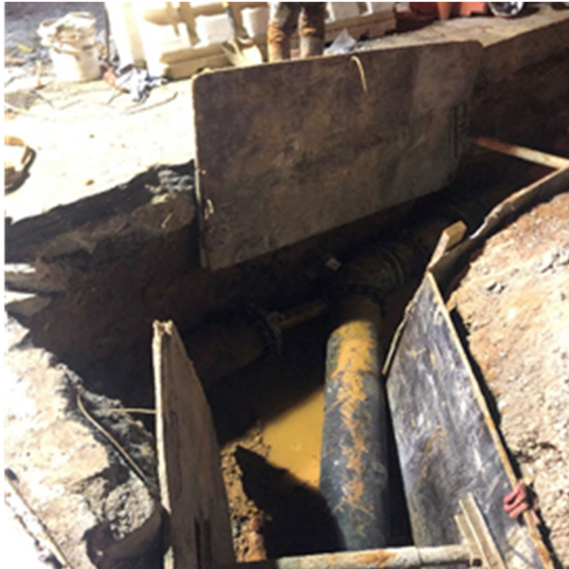
Ductile Iron Pipe Installed 2
