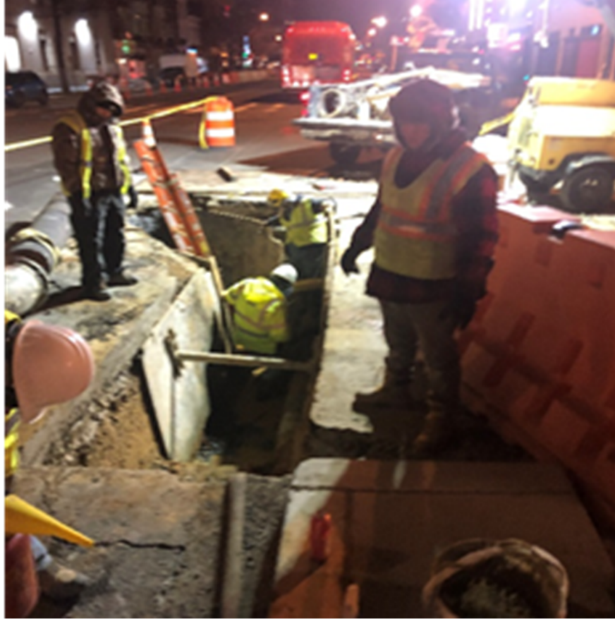
Omni setting up shoring in trench
