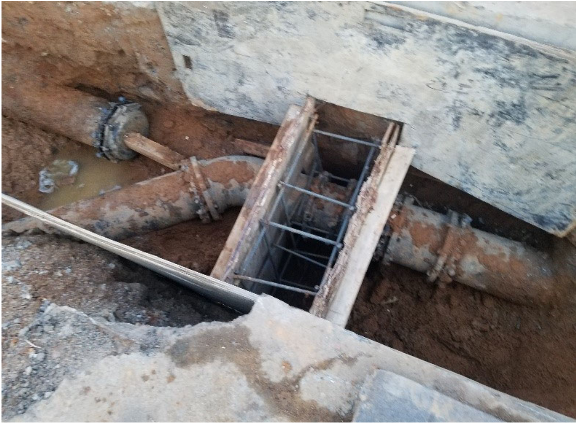
Thrust block form work in place
