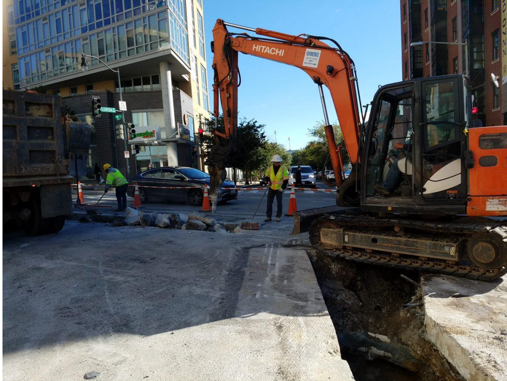
Excavating for Electrical Trench at 14 th and Florida Ave
