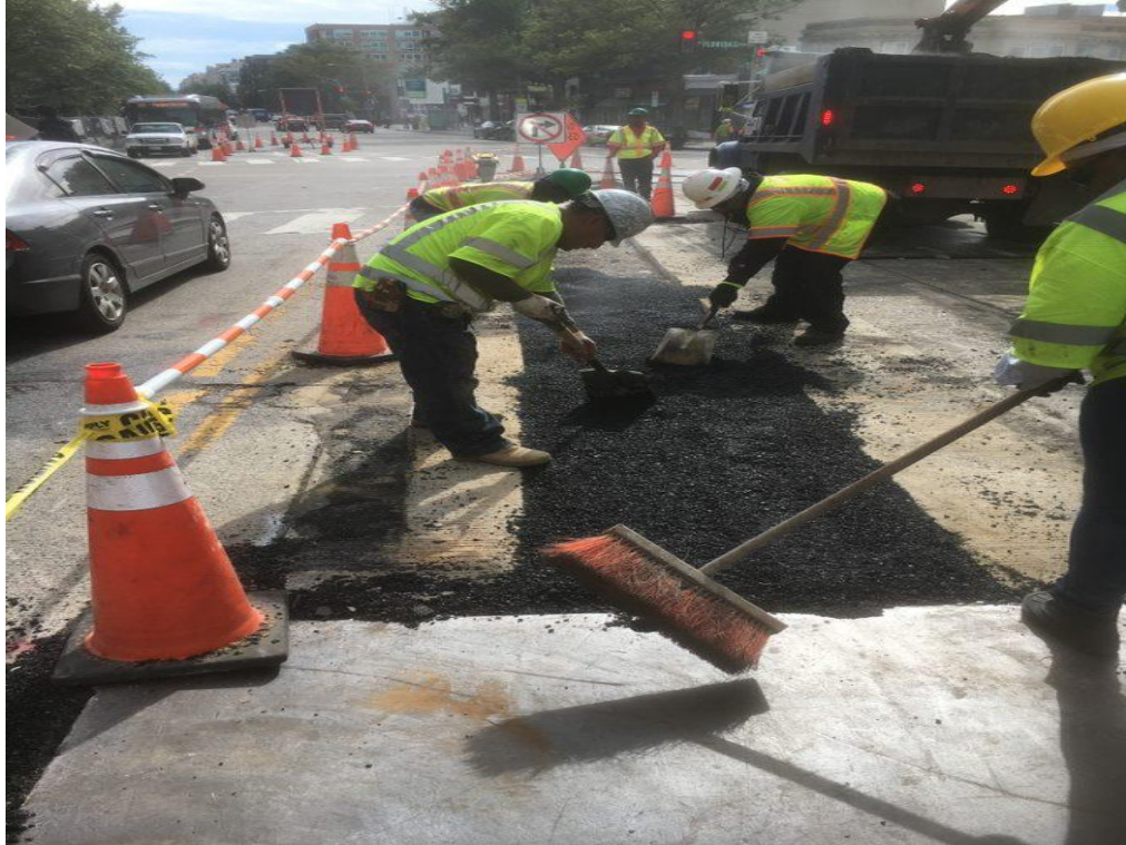
Placing Temporary Asphalt over Electrical Trench at 14 th and Florida Ave
