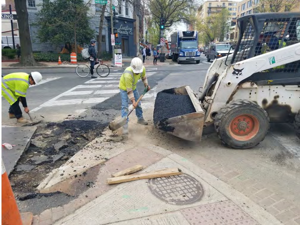
Placing Temporary Asphalt at NEC of Rhode Island Ave
