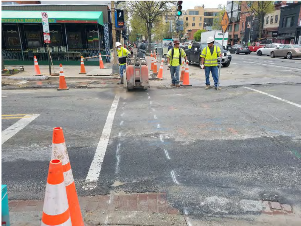
Saw Cutting for PVC Conduit at P Street
