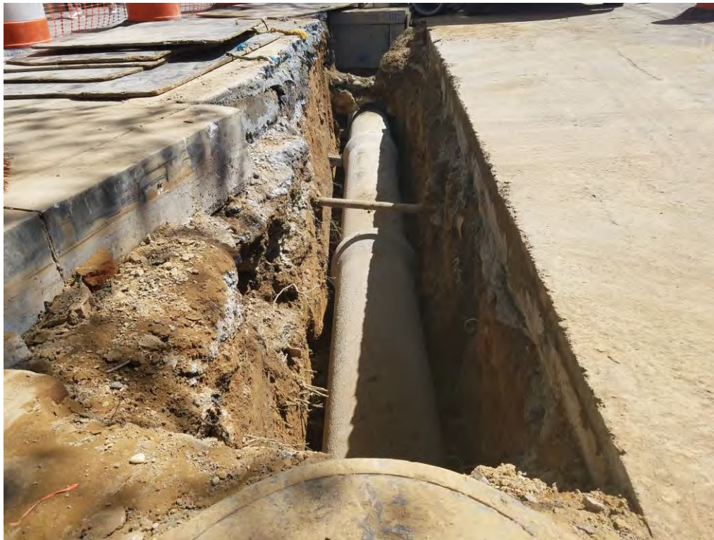
15" PCC Connection Pipe for CB-04
