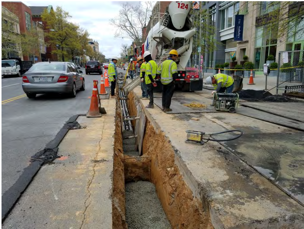
Encasement of PVC Conduit between P Street and Church St.
