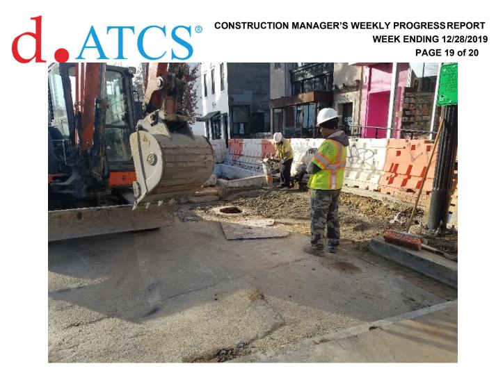
Omni backfilling and compacting sewer manhole M27
