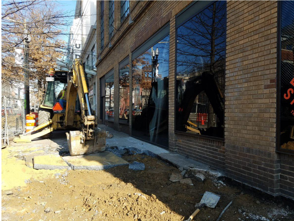
Demo of existing PCC Sidewalk between P Street and Q Street
