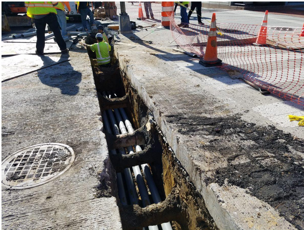
4" PVC Conduit installation at the SW Corner of V Street
