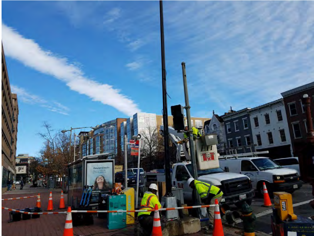
Construction of Temporary Traffic Signal
