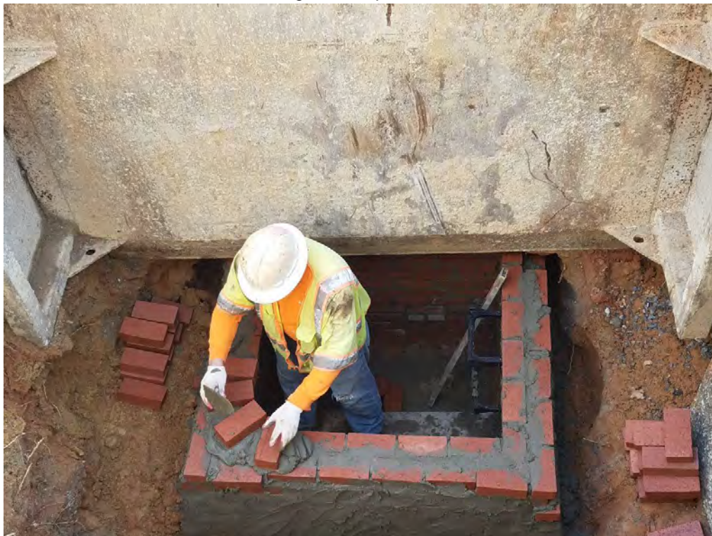
Installation of Brick Combine Sewer at MH23
