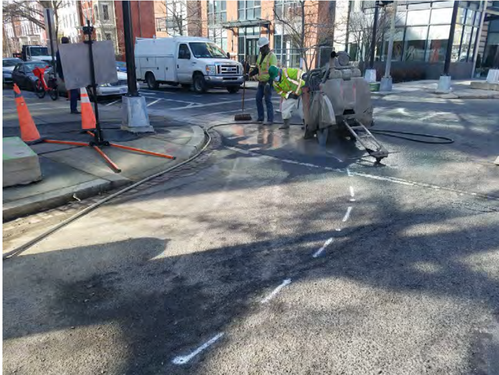
Saw Cutting for Bump Out installation
