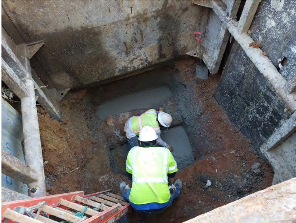
Placement of PCC pad for Sewer Manhole (MH16)
