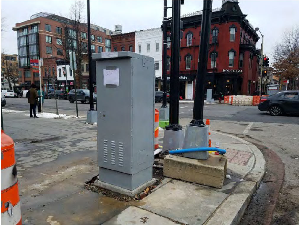
Installation of Traffic Controller Cabinet at P Street
