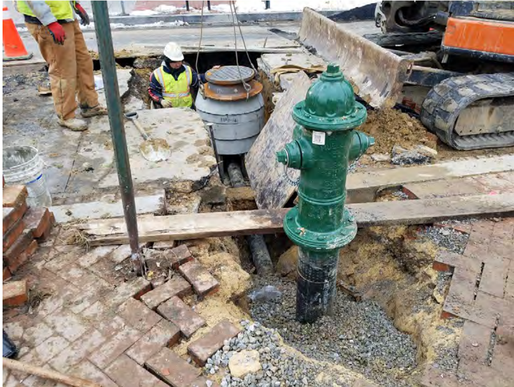
Installation of Fire Hydrant at 14 th and Swann
