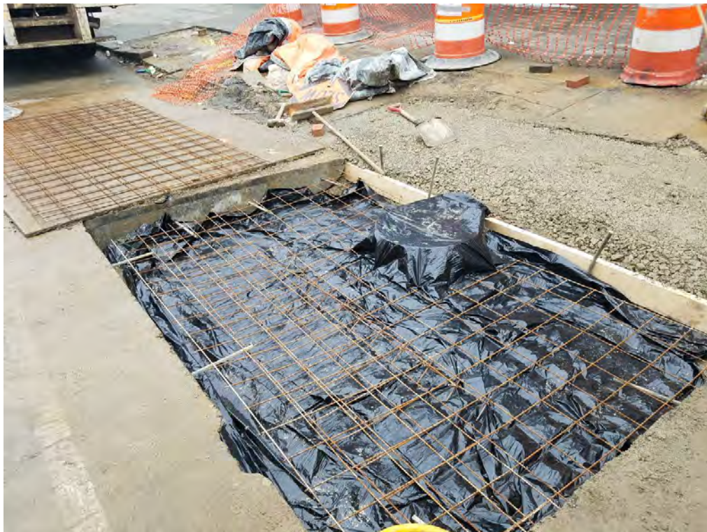
Installation of PCC Base at 14 th and T Street
