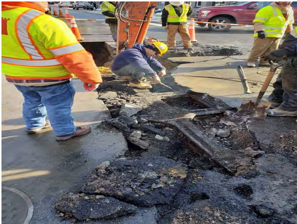
Removal of Streetcar Tracks at 14 th and U Street
