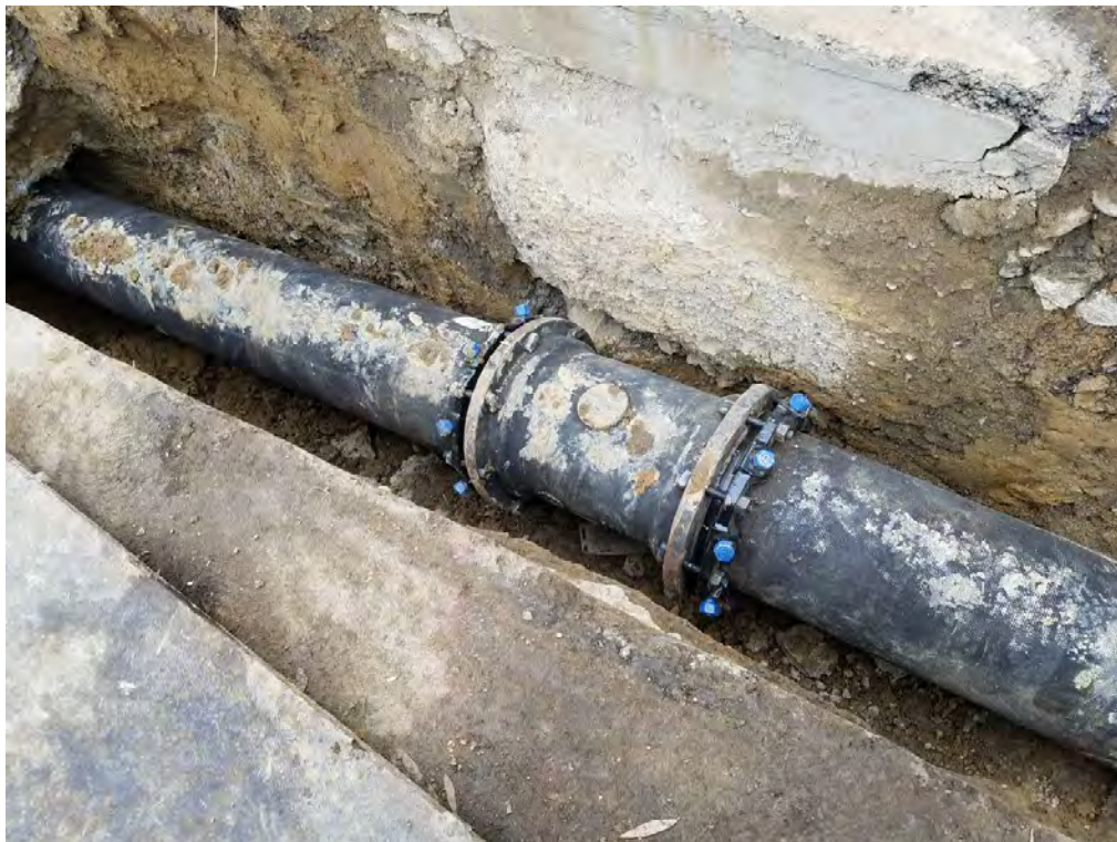
Installation of 8" Water Main on T Street on Westside
