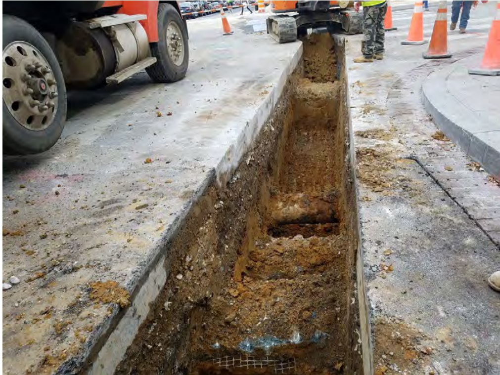
Excavation for PVC Conduit (Electrical Trench) between W and V Street
