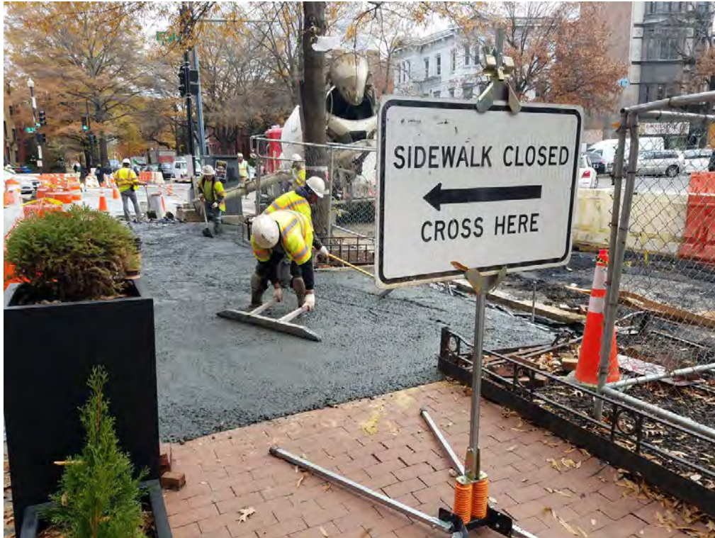
Placing PCC Sidewalk between N Street and Rhode Island Ave
