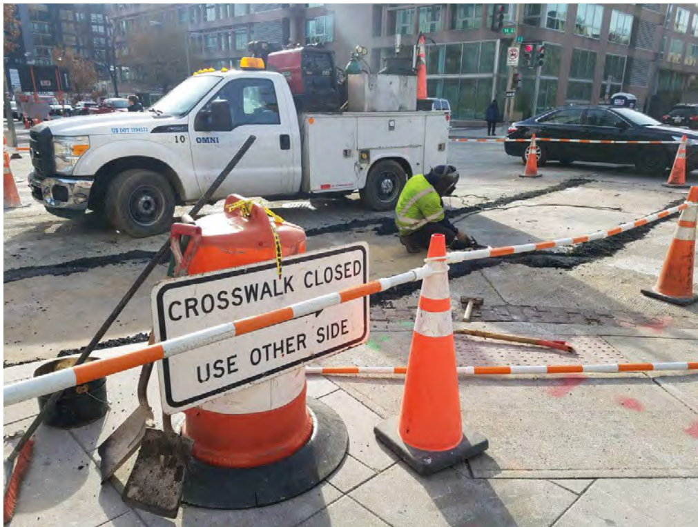
Welding Steel Plate between W Street and V Street
