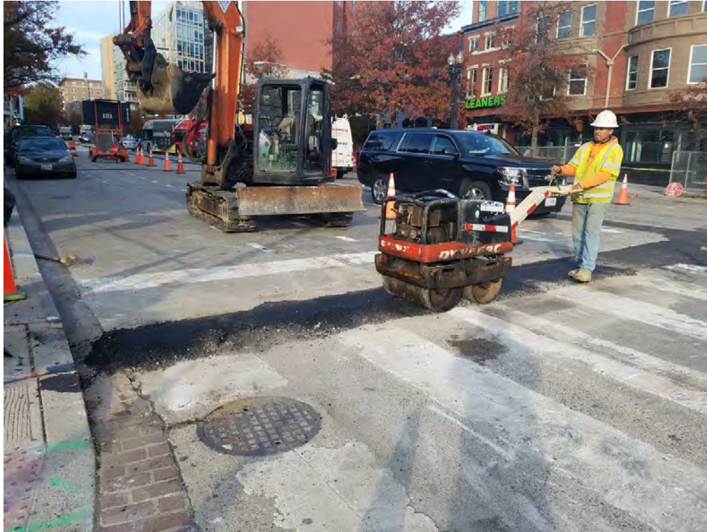
Placing temporary Asphalt over Electrical Trenched between W and V Street
