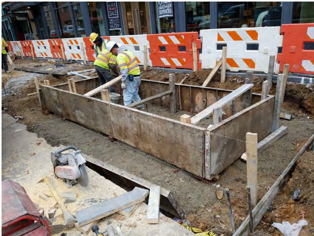
Forming the concrete walls of Bioretention Planter #1
