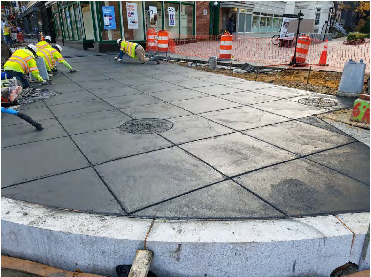
Placement of PCC Sidewalk at SW corner of Rhode Island Ave
