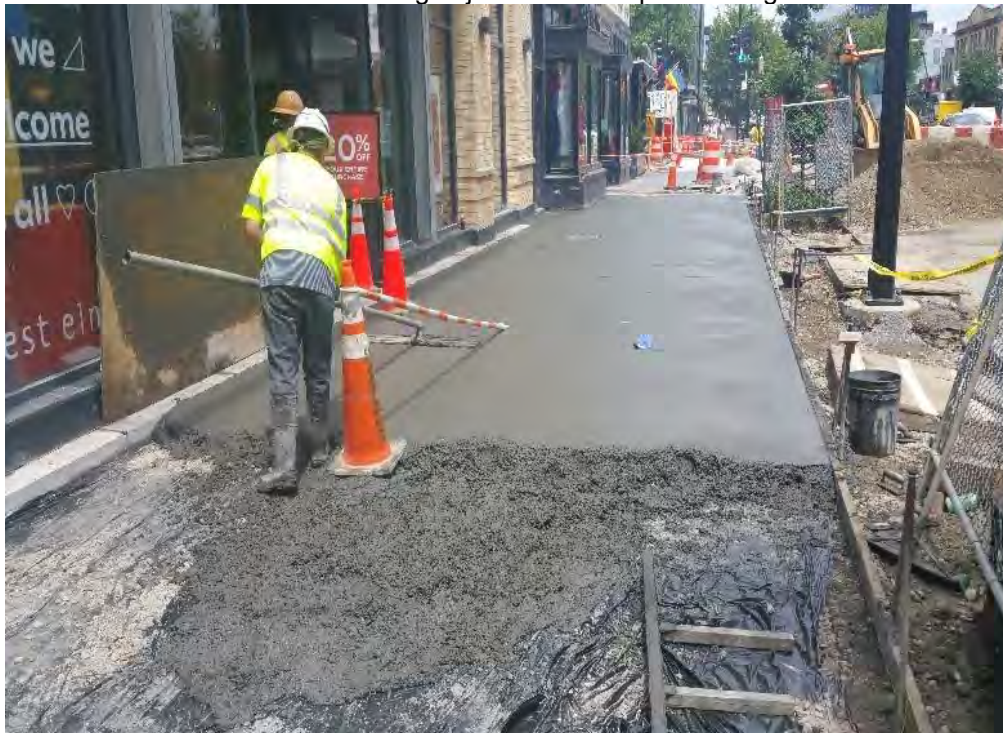
PCC sidewalk placed from 1732 to 1726 14 th St.
