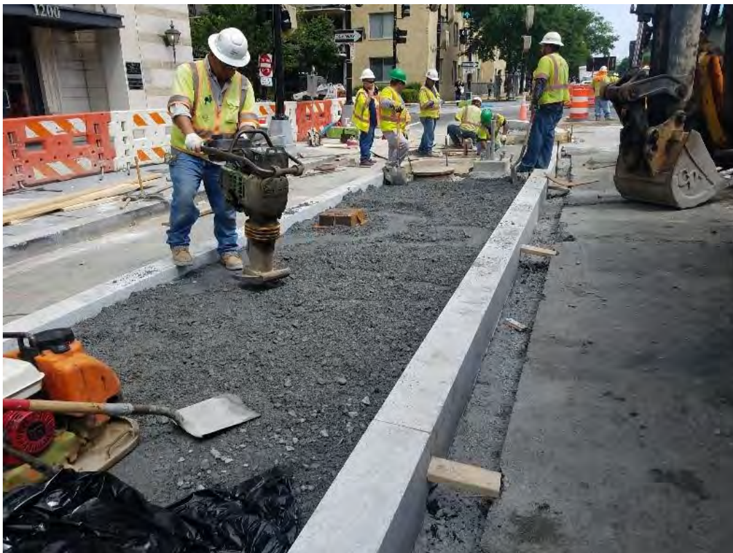
Granite curb installation and grade check by FMCC. .
