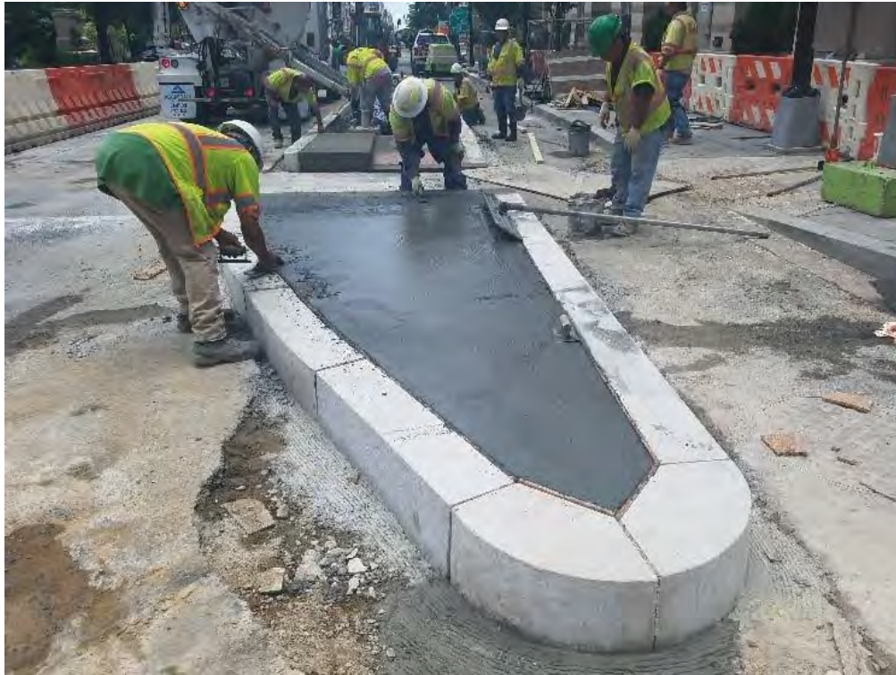
Granite curb installation at north section of bus island.
