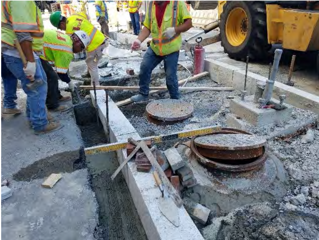
Granite curb installation and grade check by FMCC. .
