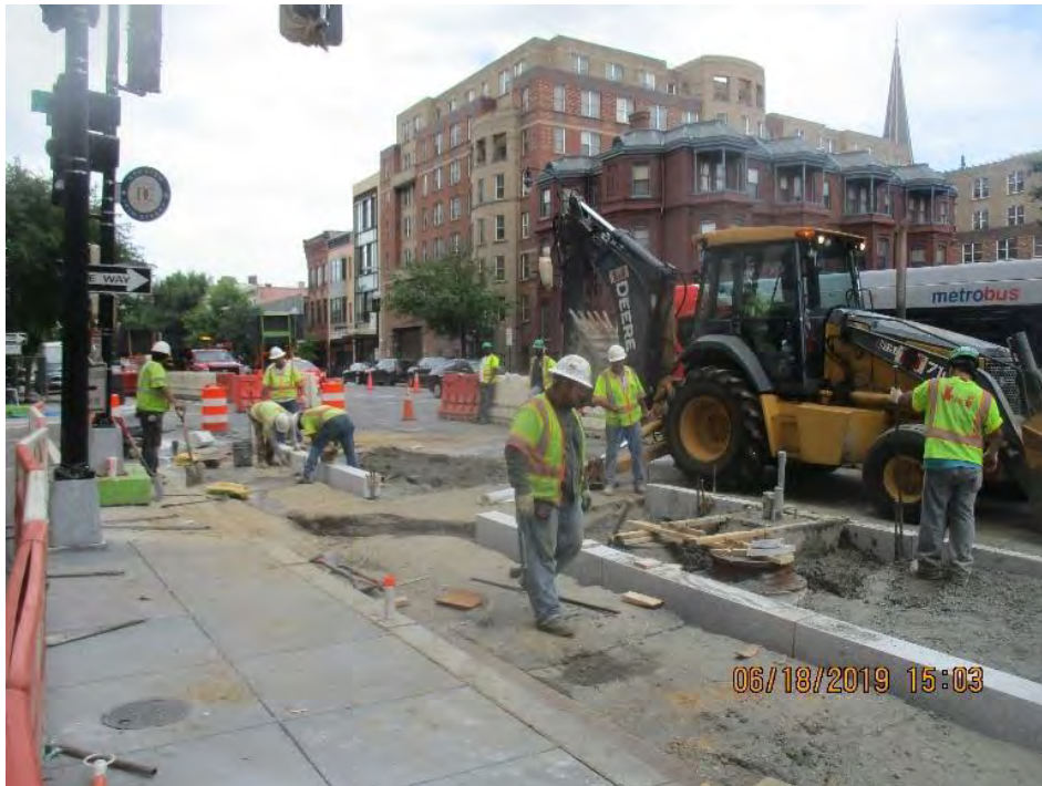
Omni poured the concrete for the Street Light Pole Foundation (TS06) within the area of the proposed Bus Island at 14 th & N Street NW
