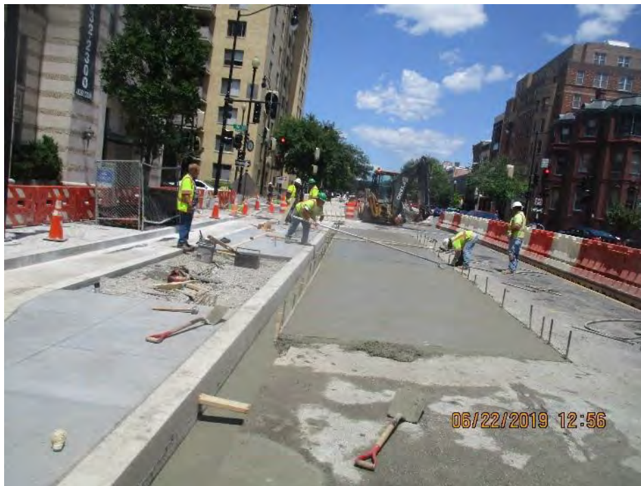
Omni poured the concrete for the Street Light Pole Foundation (TS06) within the area of the proposed Bus Island at 14 th & N Street NW
