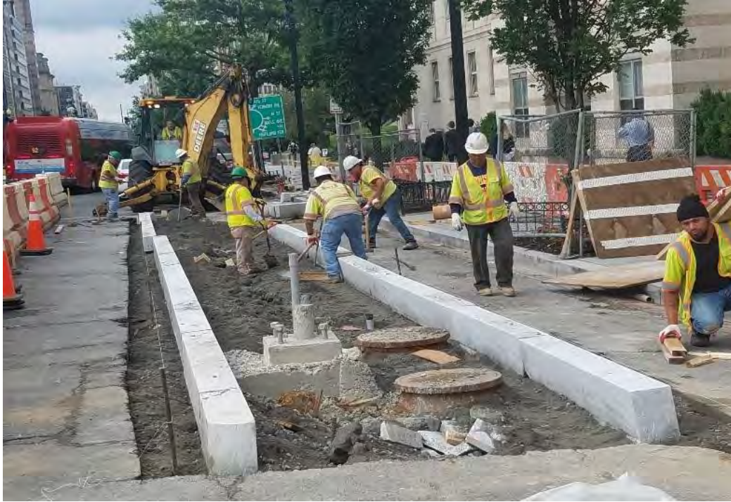
Granite curb being adjusted east as per drawings.
