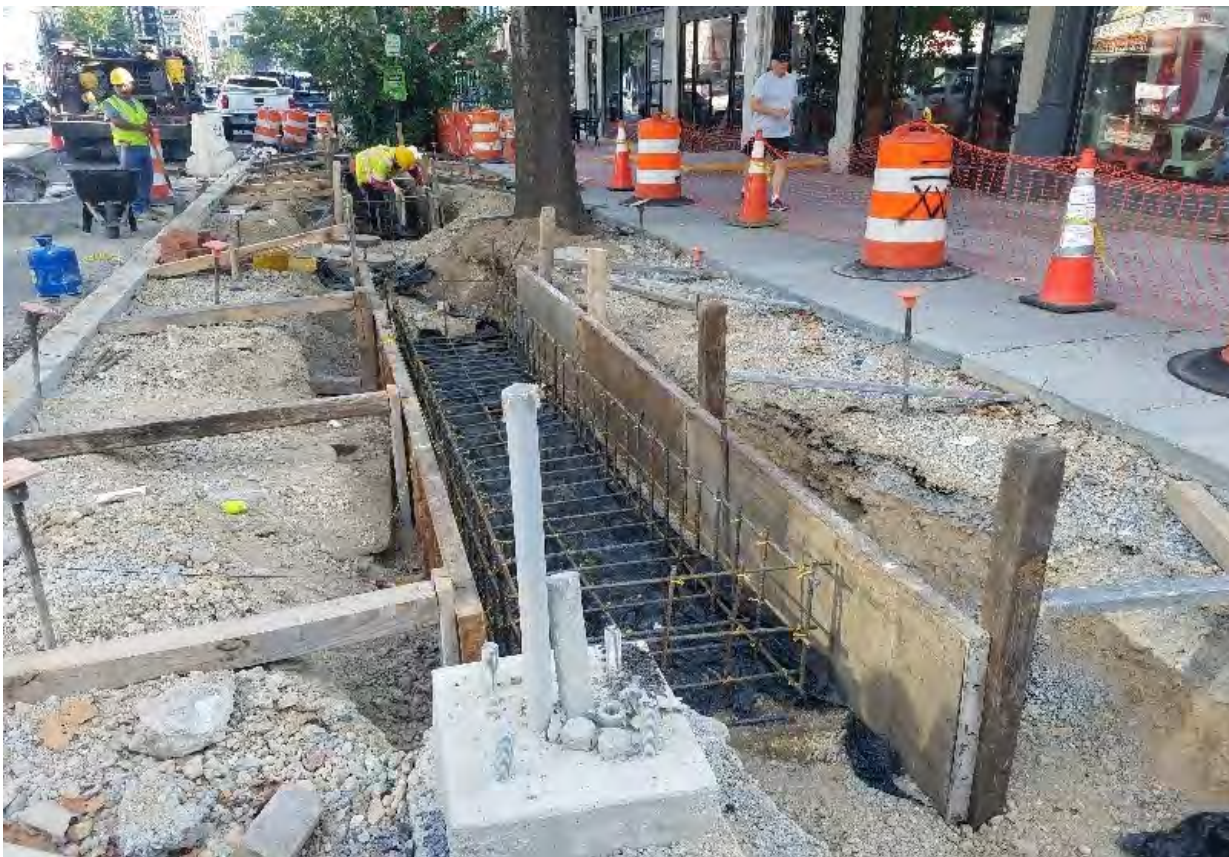
reinforcement for trench drain location at 1819-1825 14 th St by D.E.N.
