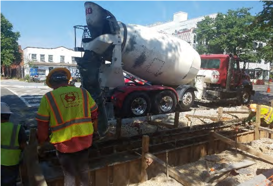
Concrete placement for trench drain underway.
