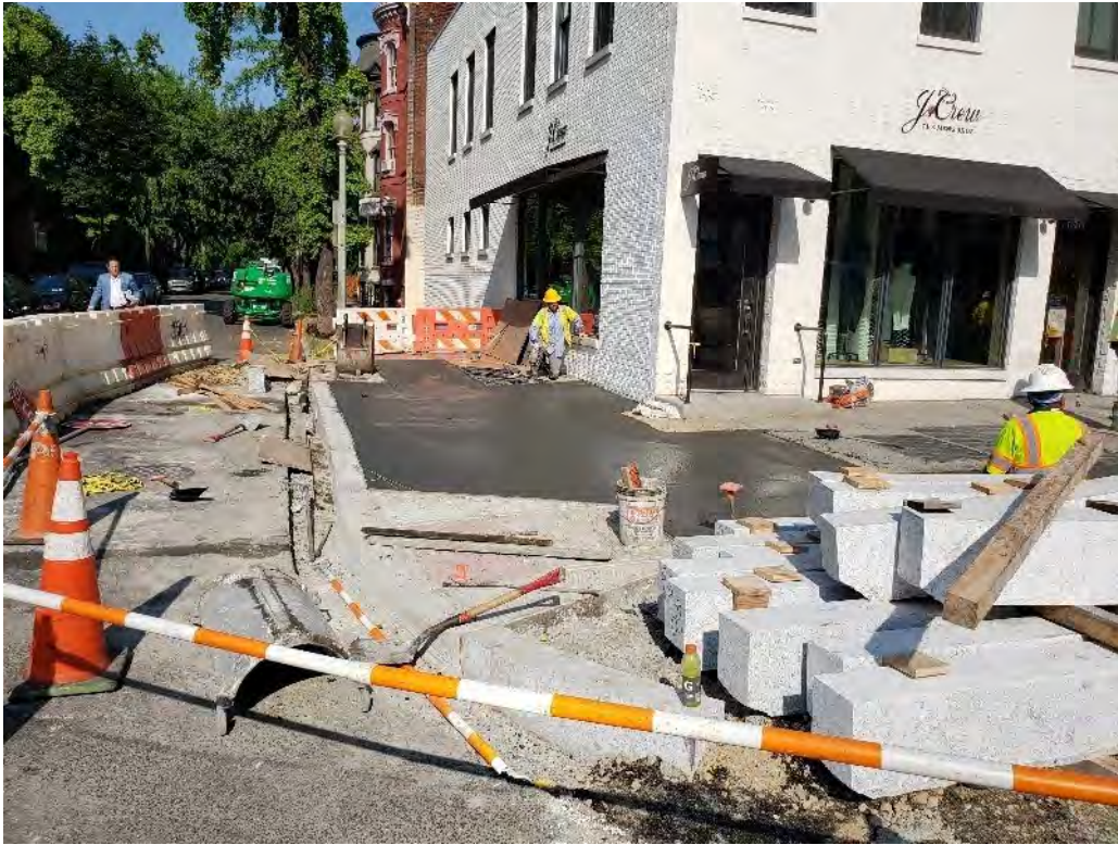
D.E.N. crew sealed off the work zone & set up Cones and Barriers for Wheel Chair and Peds Traffic per MOT Plan.
