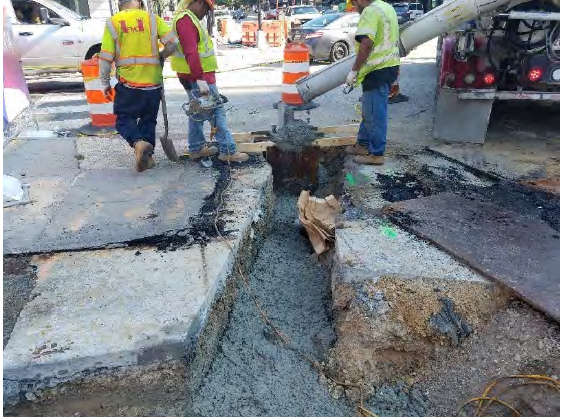
Concrete placed at TS51 foundation
