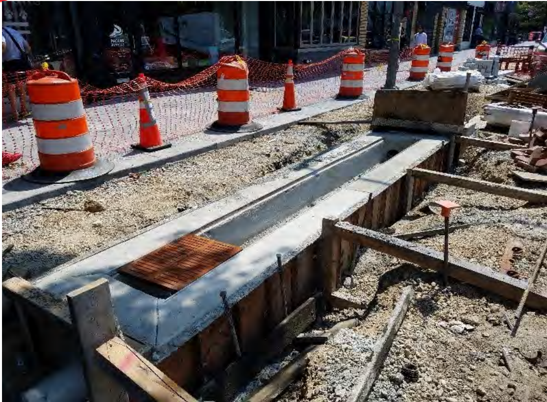
Second section of trench drain at 1821 14 th St
