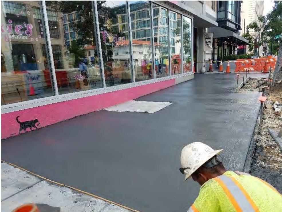
Finishing of PCC sidewalk and view of existing building vault to be replaced
