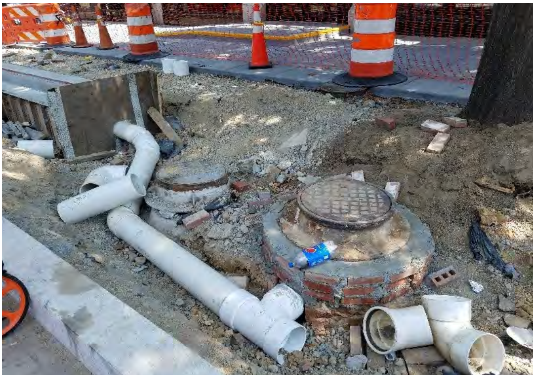
8" PVC pipe from trench drain to existing sewer manhole
