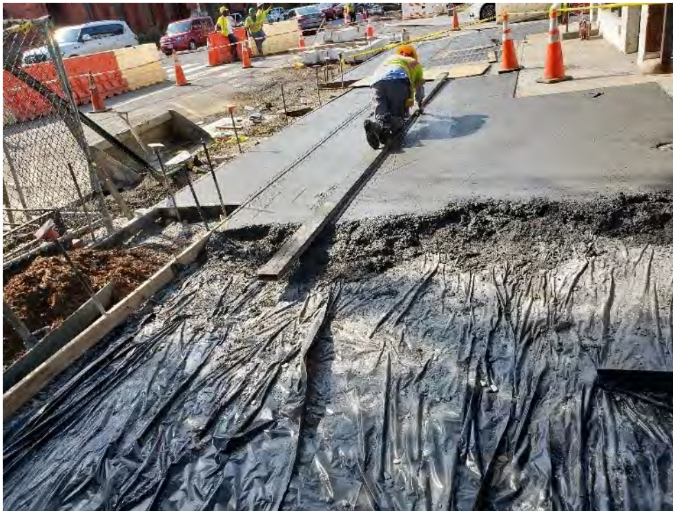
D.E.N. crew sealed off the work zone & set up Cones and Barriers for Wheel Chair and Peds Traffic per MOT Plan.
