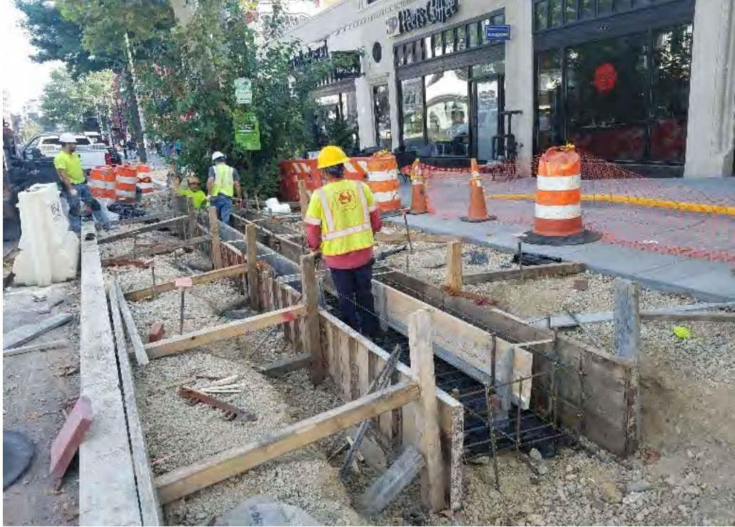
Continued formwork by D.E.N. at trench drain
