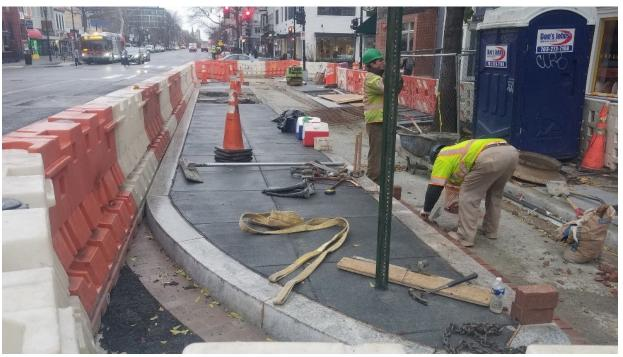
Finished installing brick gutters at the bus island at NWC of T Street
