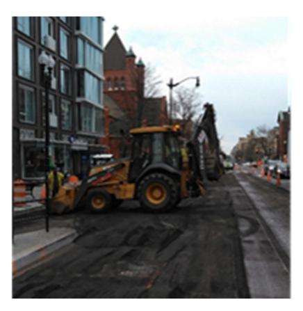
Manual pickup of milling spoils near Corcoran
