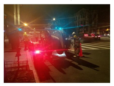
Spool truck to be used to run new cable to Pepco manhole.
