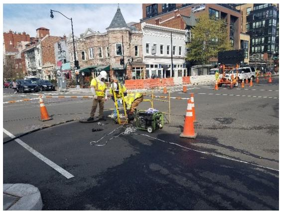
FMCC splicing cable at manhole M66
