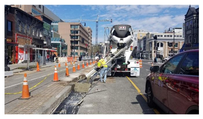
Concrete placement for the trench at SWC of U Street
