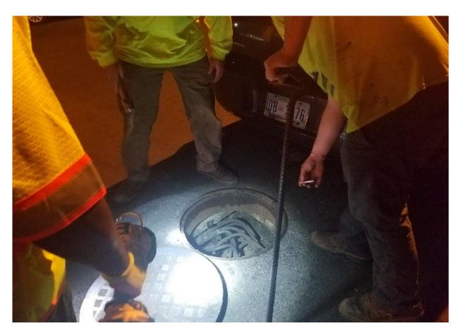
Pepco manhole with communication cable to be removed and replaced.
