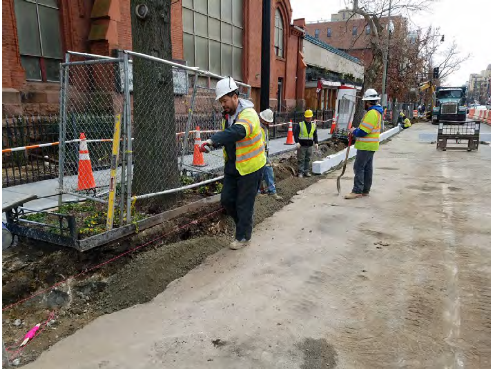
Installation of Granite Curb between Q Street and Corcoran Street
