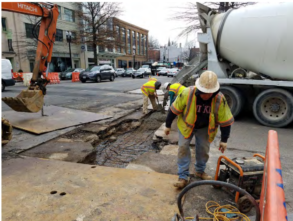
Placement of PCC Base at 14 th and T
