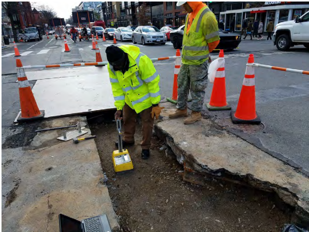
Compaction Testing of Aggregate Base Material
