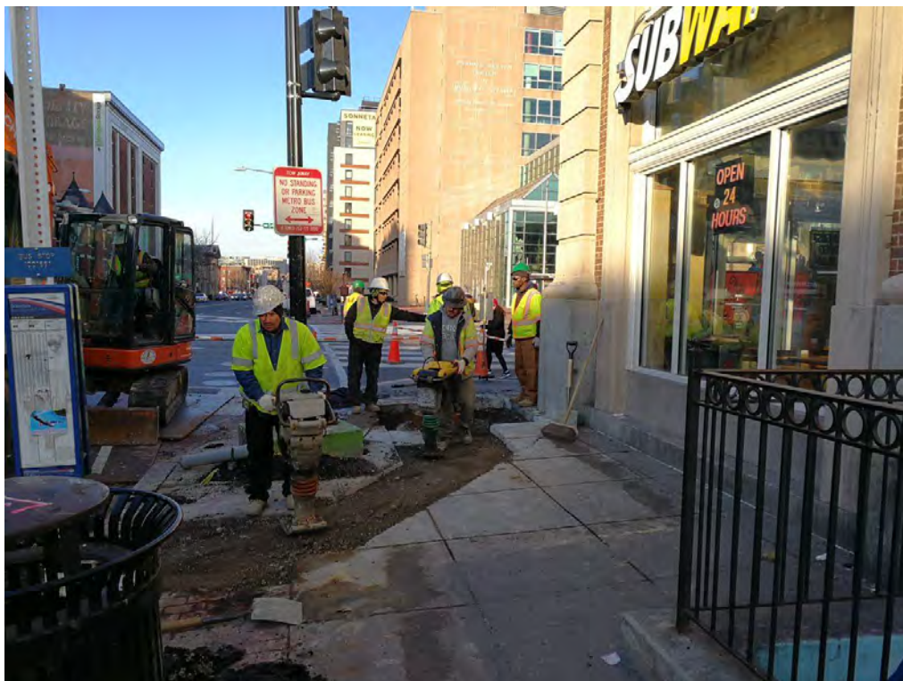
Placing Backfill at the NE Corner of 14 th and U Street
