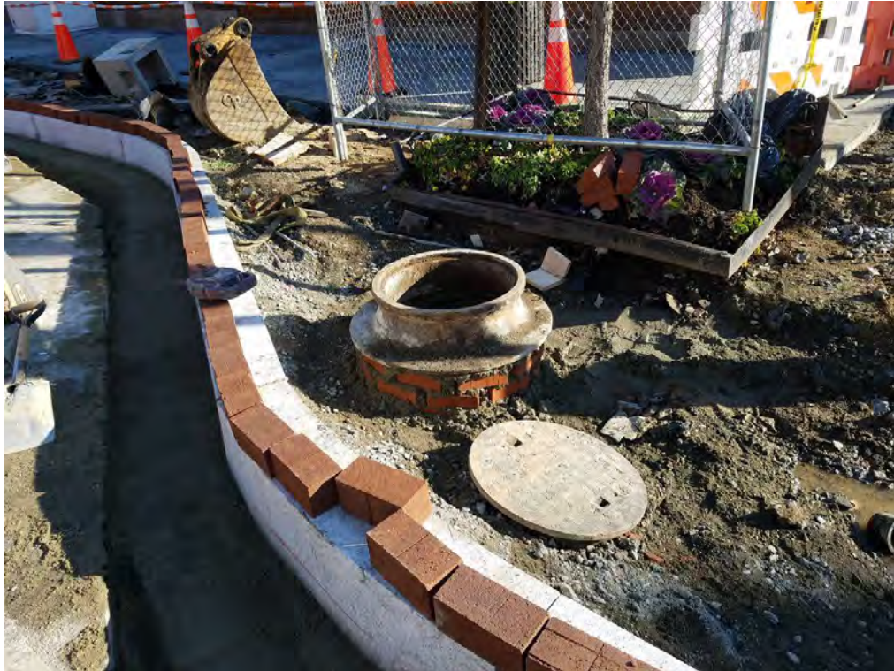
Sewer Manhole Adjustment at 14 th and Q Street
