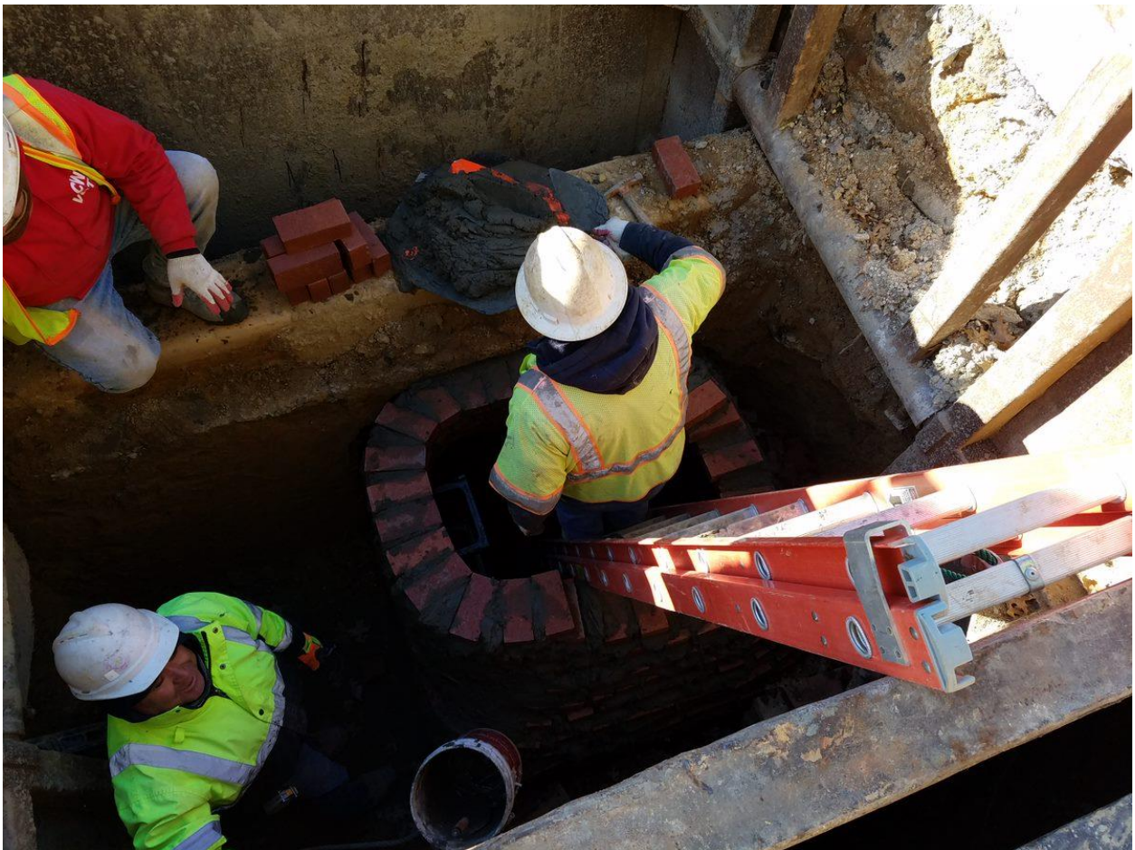
Building Brick Combine Sewer Manhole across from 14 th and Swann
