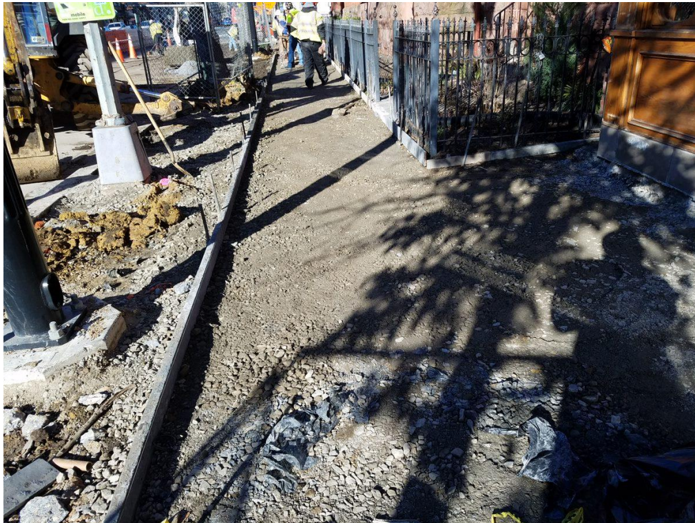
PCC Sidewalk Replacement between Q Street and Church Street
