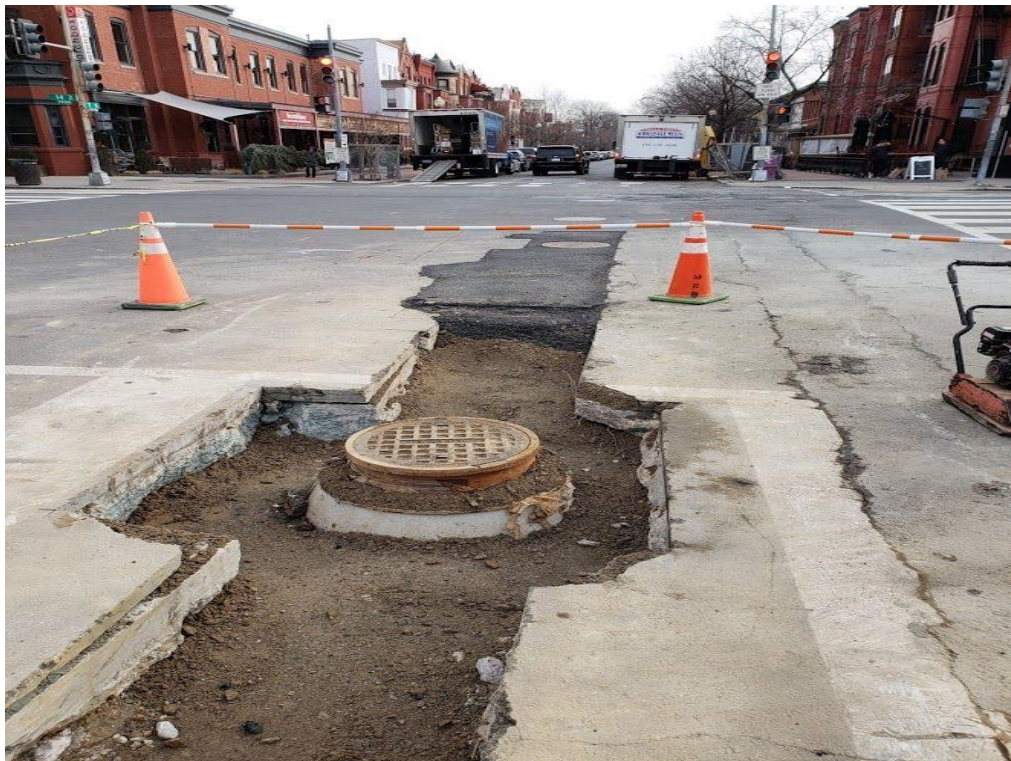
Backfill over 8" Water Main on T Street Westside
