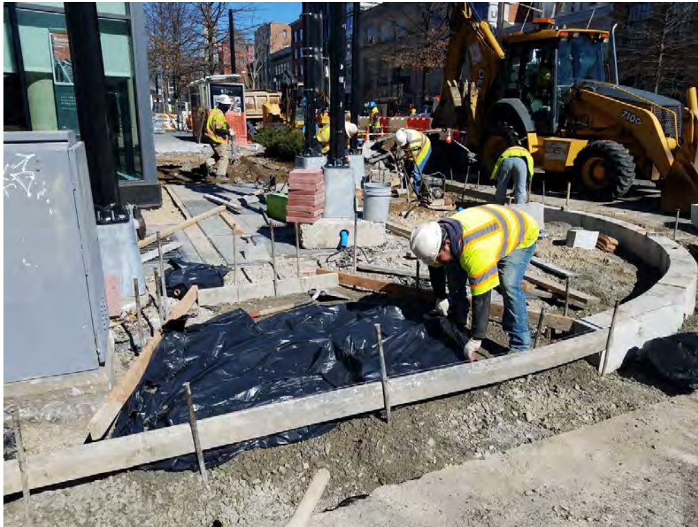
Bump Out at the NW corner of 14 th and P Street
