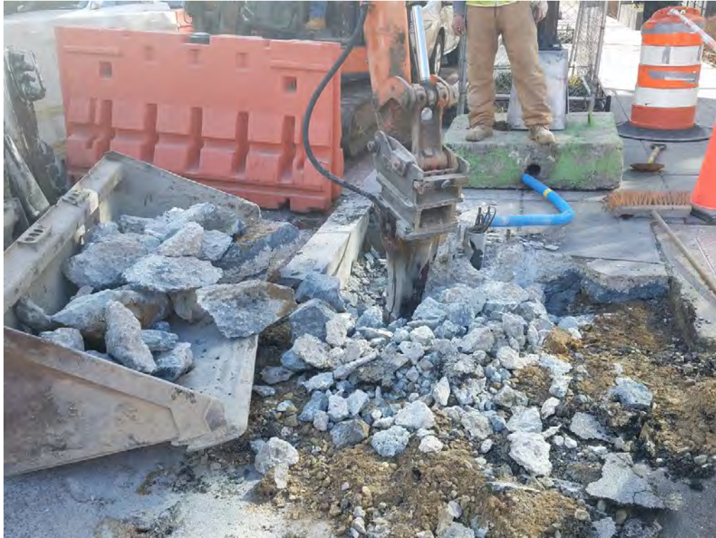
Removing of old Traffic Signal Foundation
