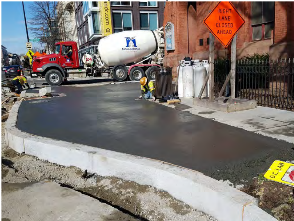
Installation new PCC Sidewalk
