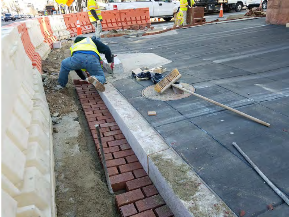
Installation of Brick Gutter
