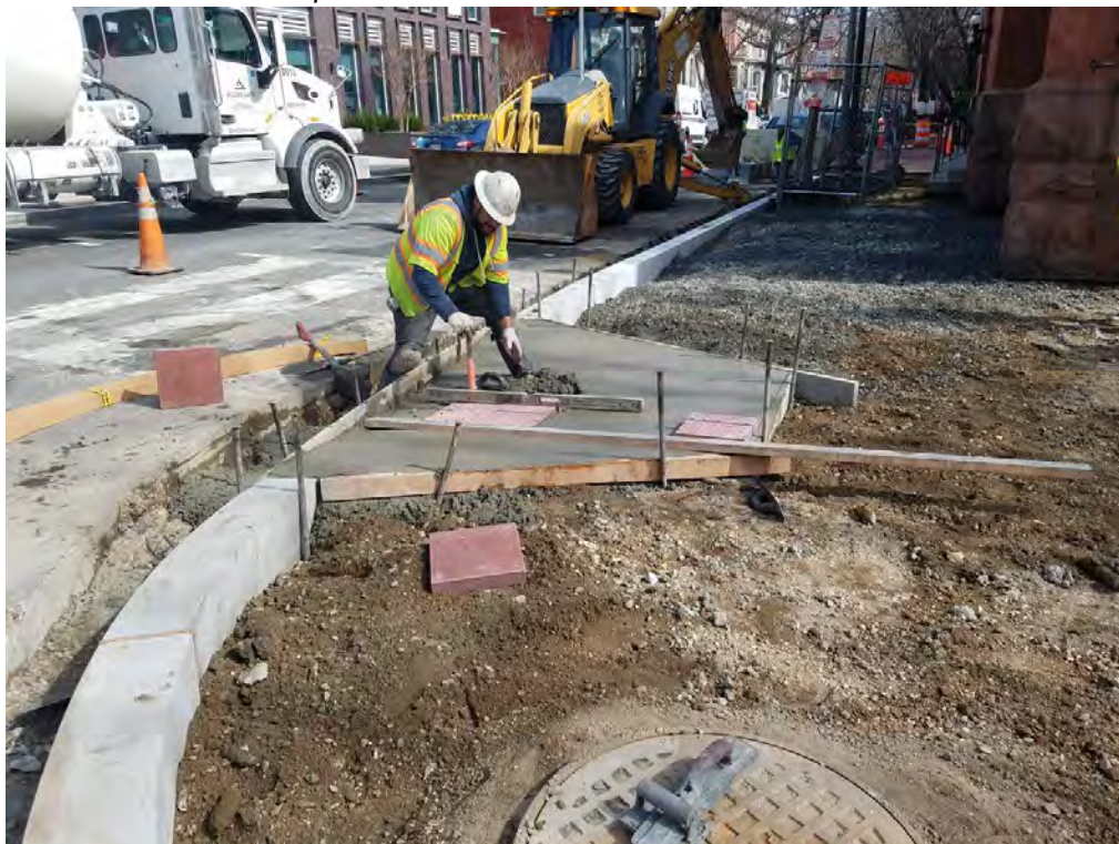
ADA Ramp installed at the SE corner of Corcoran Street
