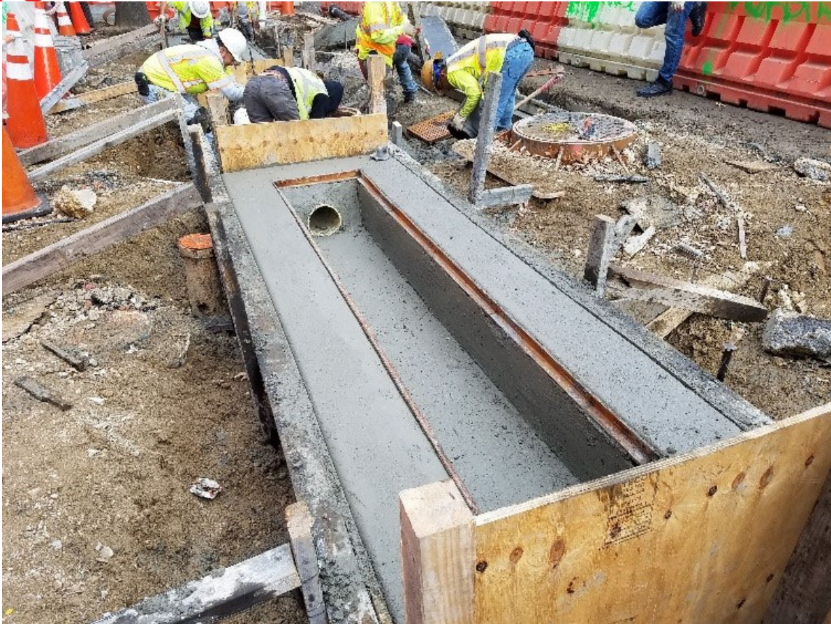
Formwork stripped and finishing underway.
