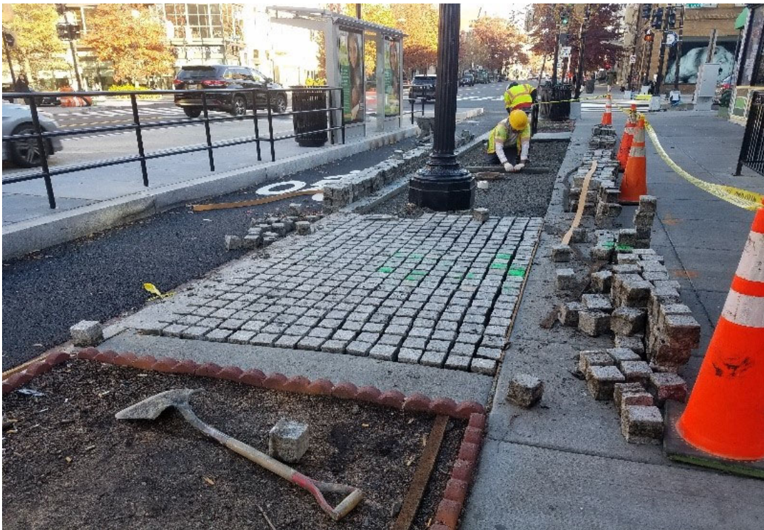
Permeable Pavers repaired at 1400 blk of 14 th St by D.E.N.
