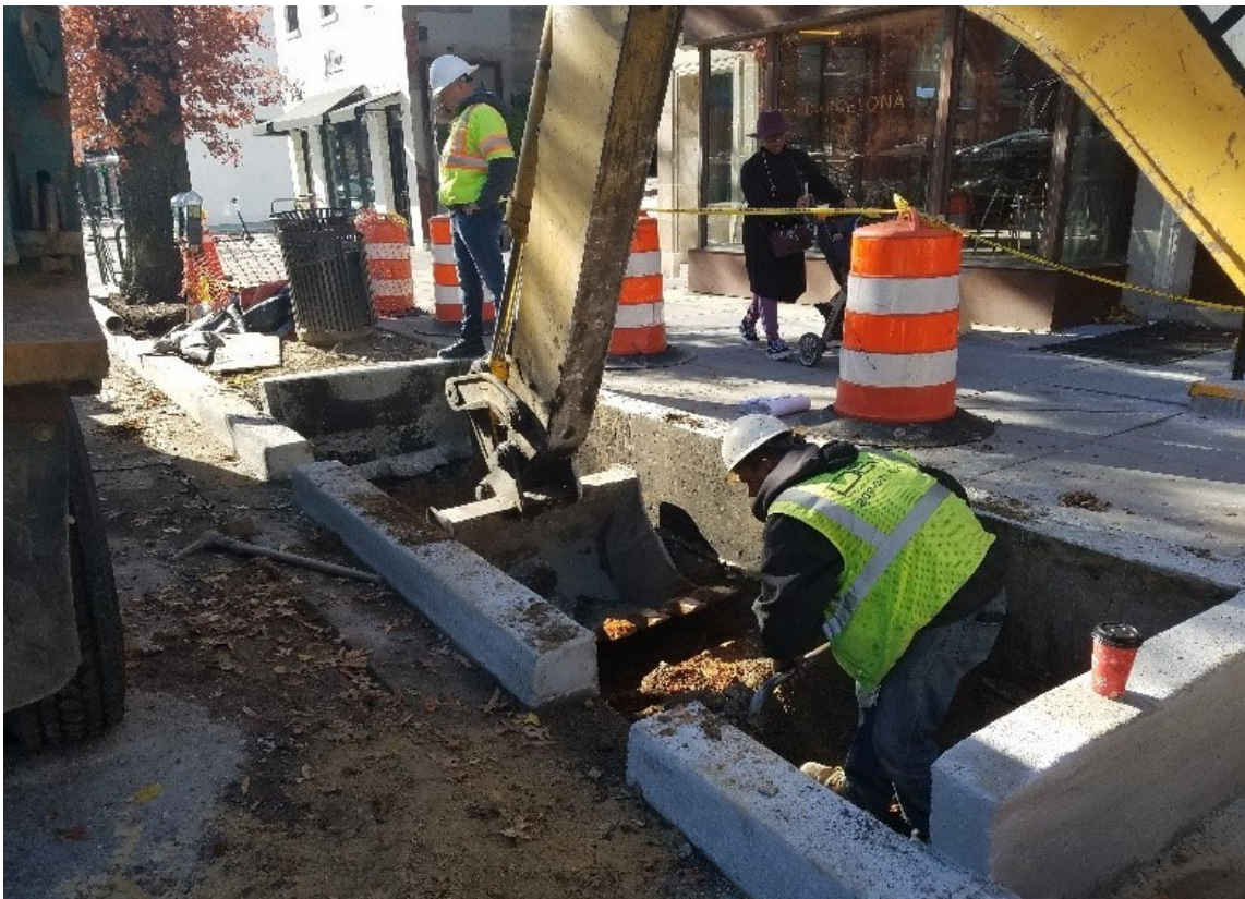
PCC sidewalk removed and subgrade prepared from 1716 to 1722 14 th St
