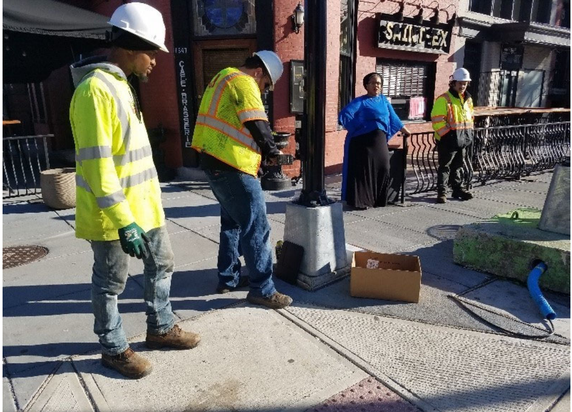
APS Unit installed at T St by FMCC
