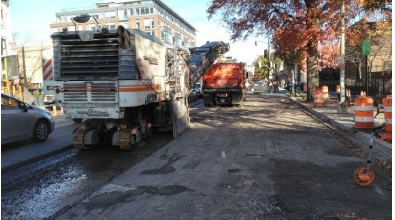
FMCC milling the longitudinal joint NB inside lane on 14th Street NW between Riggs Street and S Street
