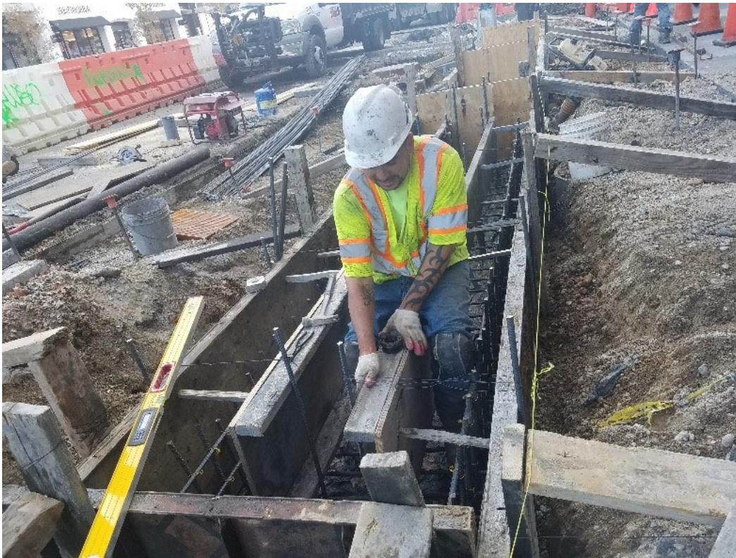
Walls formed for interceptor drain by D.E.N.
