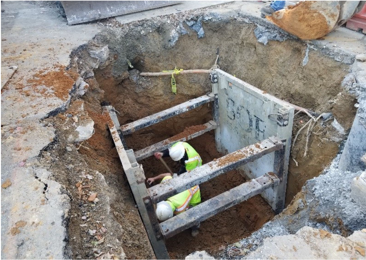
Excavation of trench for sewer manhole to be built by Omni
