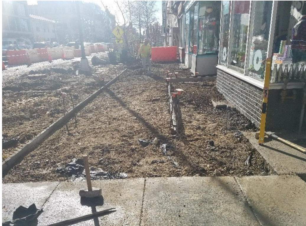
PCC sidewalk removed and subgrade prepared from 1716 to 1722 14 th St
