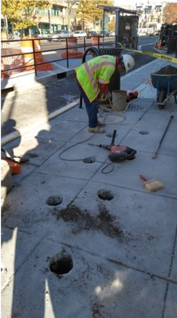
Installing bicycle racks at the NE corner of U street and 14 th Street NW
