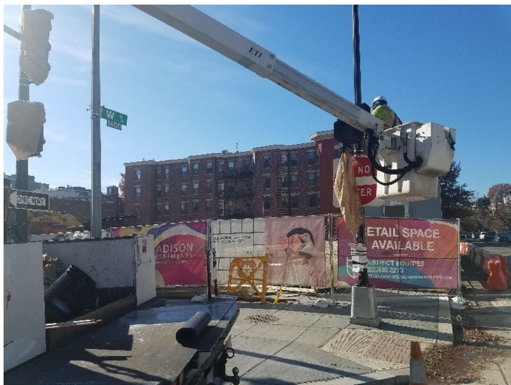
Pedestrian signal installation at SWC of 14 th & W St
