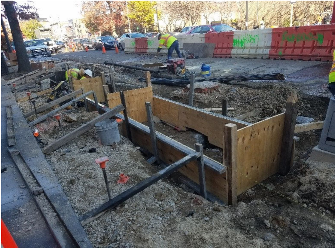
Formwork for interceptor drain underway by D.E.N.
