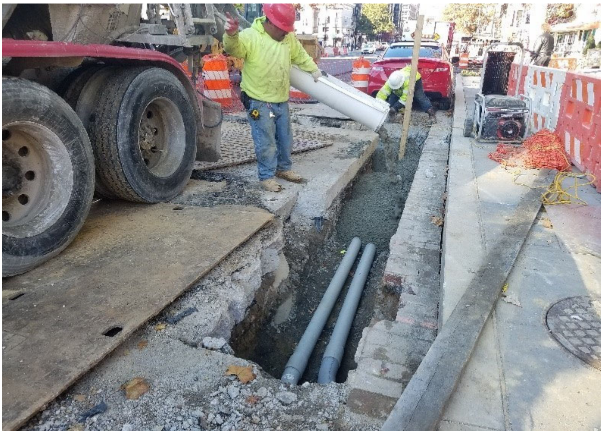
4" PVC encased from Pepco feeder P08 to M63
