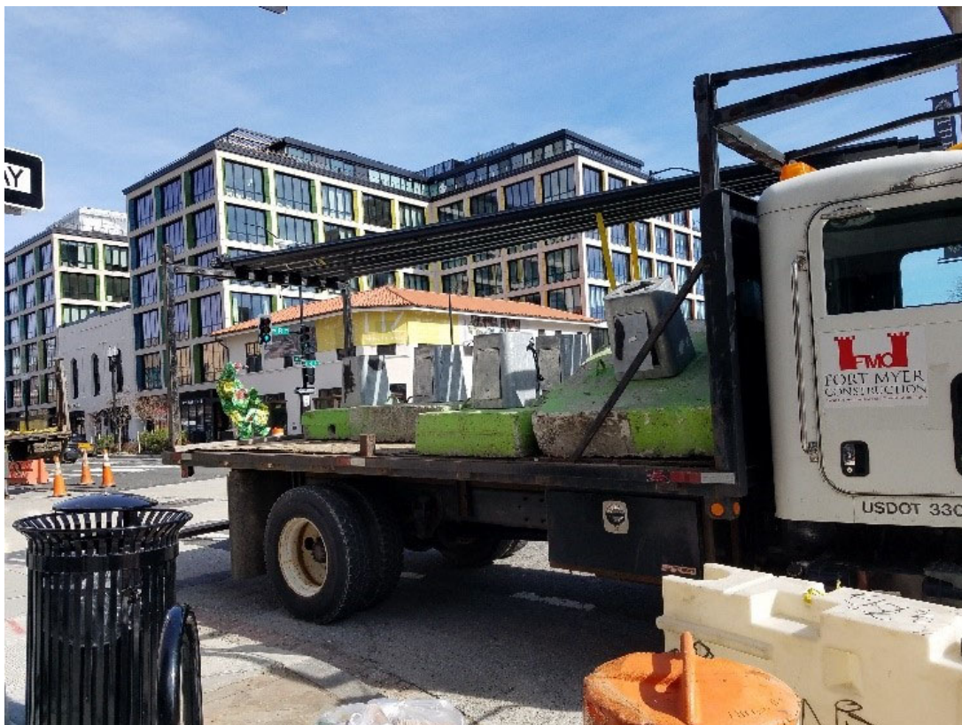
Loading of temporary bases at 14 th & R St intersection
