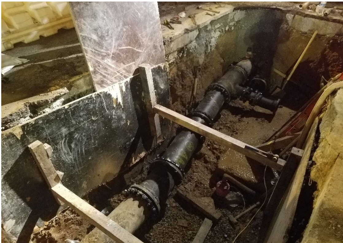
12" water main connections shown at southbound 14 th St
