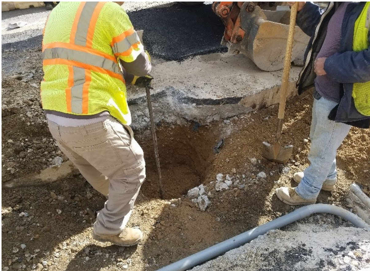
TS-27 foundation hand dug by Omni Excavators
