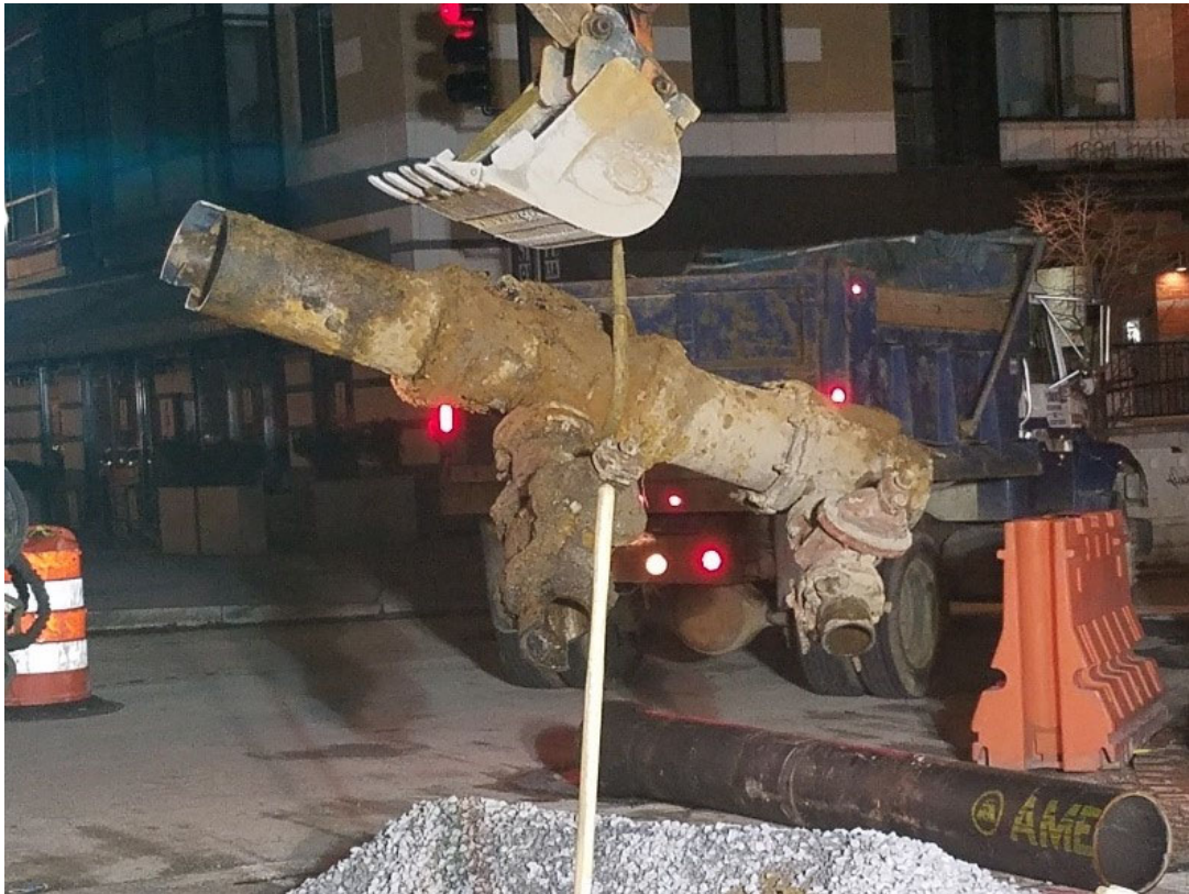
Mini excavator used to remove existing water main
