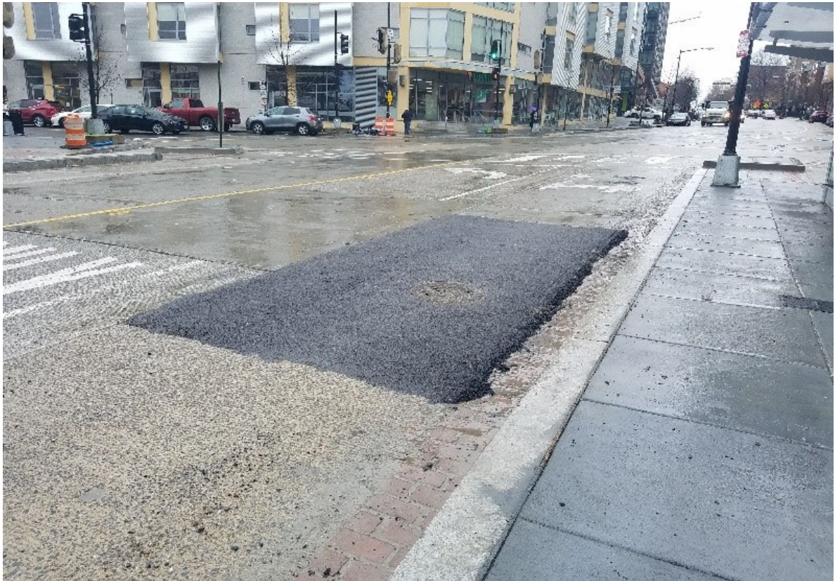
Temporary asphalt placed (7 x 14 x 0.5) at Ellisdale pothole
