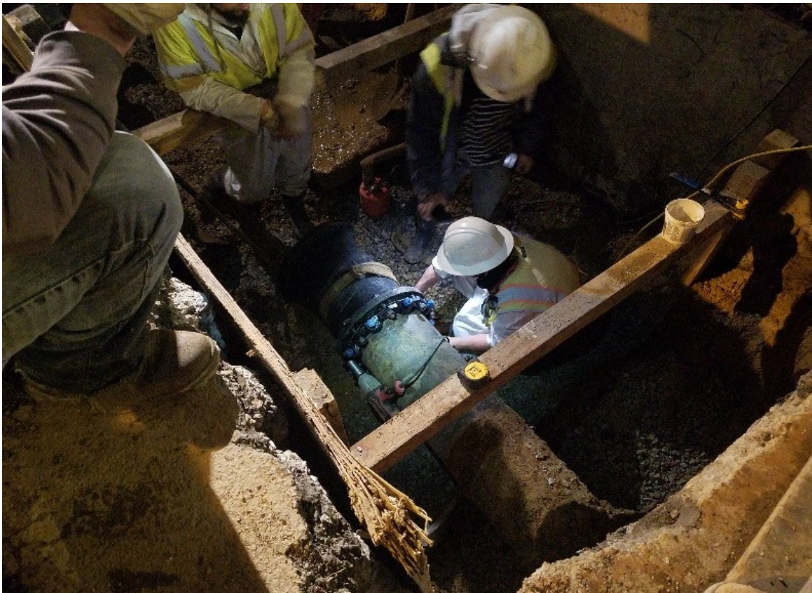
Pipe hardware installed and torque wrenches used to secure connections.
