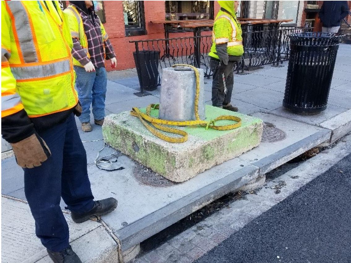
Temporary base prepared for loading
