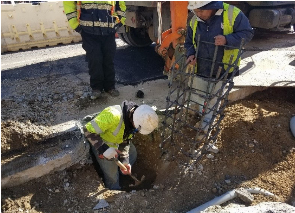
Reinforcement for TS-27 foundation
