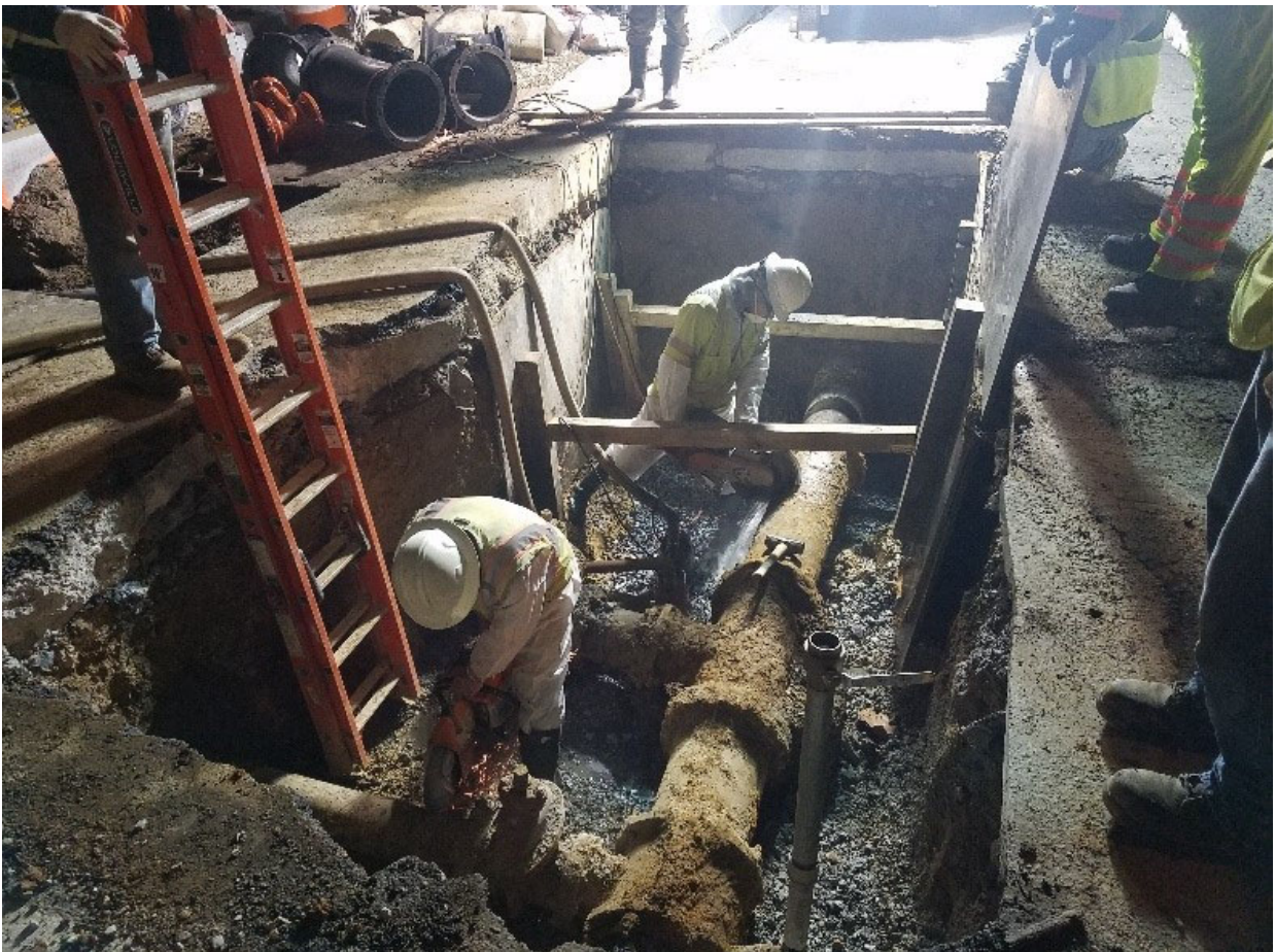
Cutting at existing 6" & 12" main
