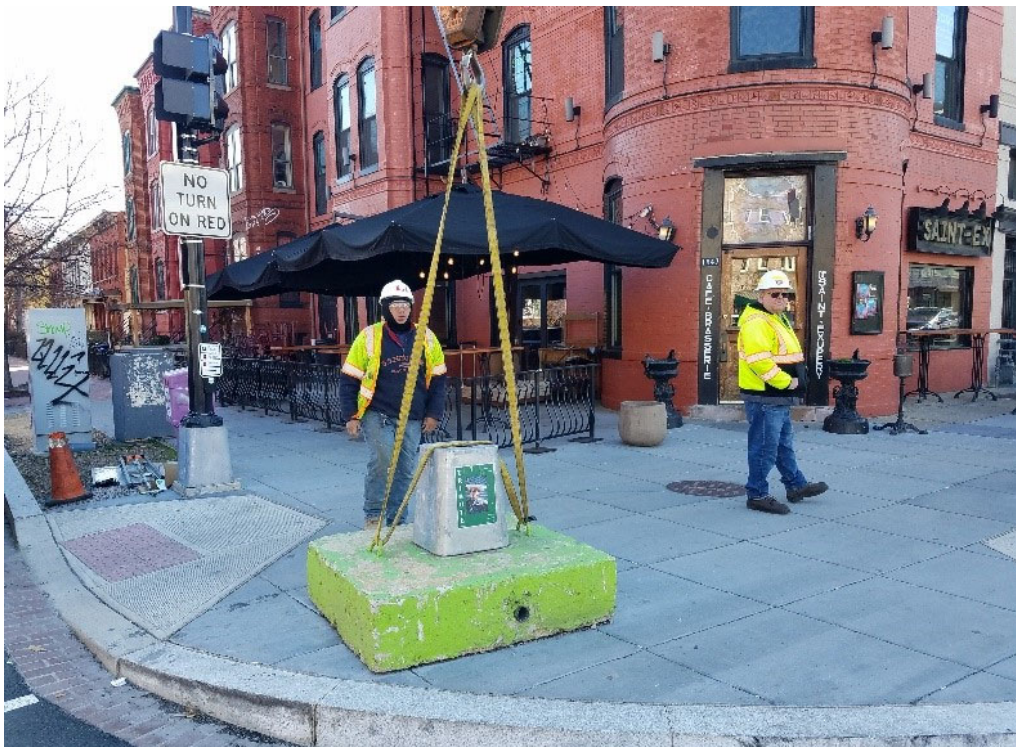
Nylon straps used to remove temporary base from corner
