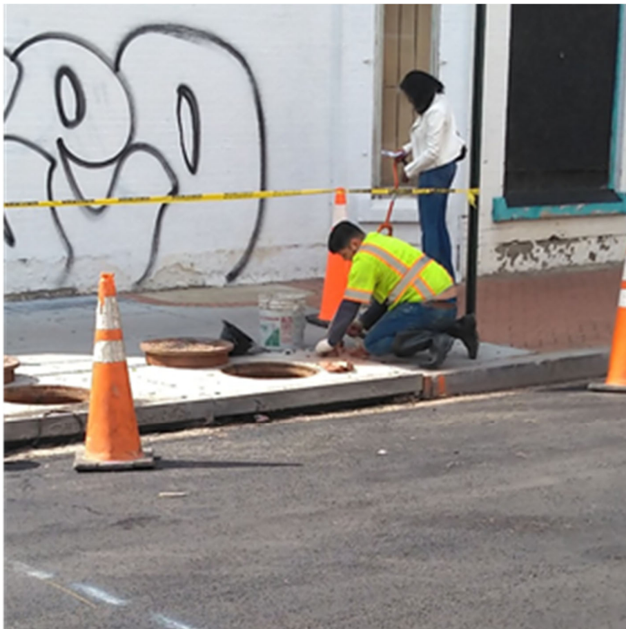
Omni Parging Manholes Corcoran Ave.
