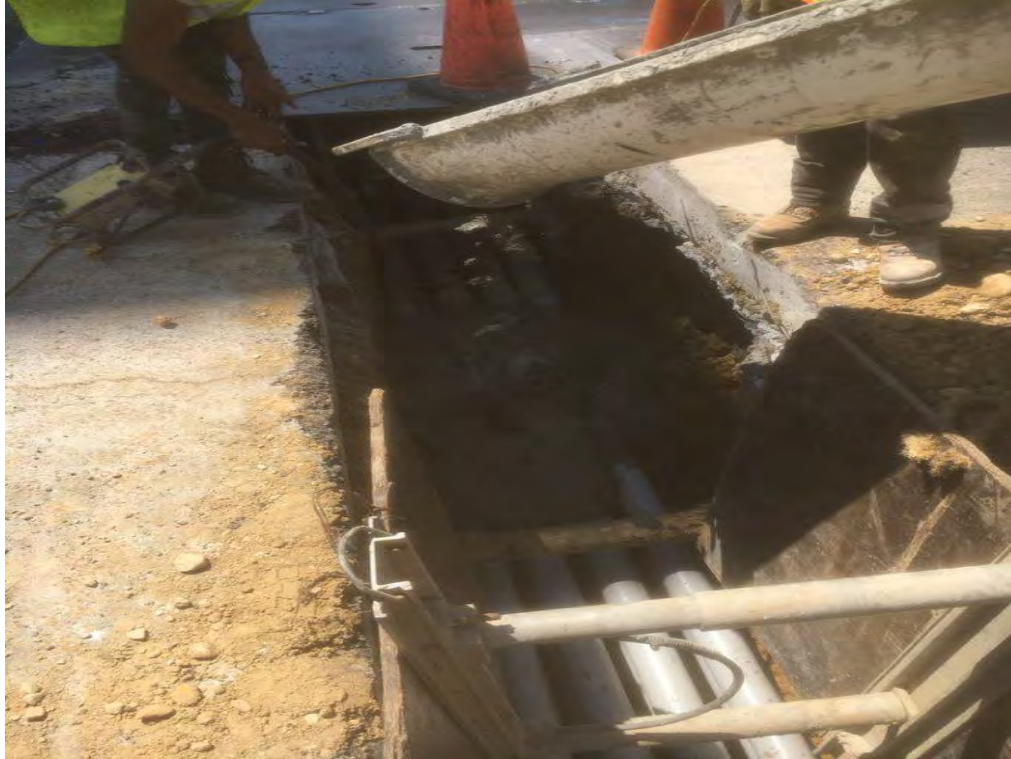
Encasement of PVC Conduit on the Westside of N Street
