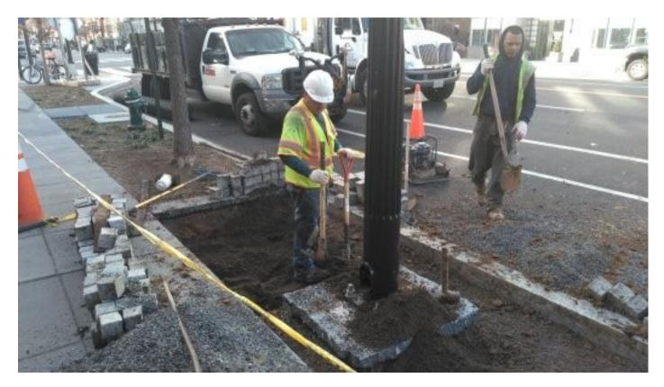
DEN excavating for structural soil prior to reinstalling the permeable pavers at NB 14<sup>th</sup> Street acroos from the LA Diplomate Restaurant
