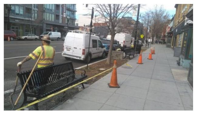
DEN removing the permeable pavers to install geo grid at 1805 14th Street NW
