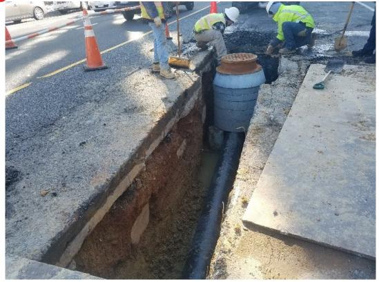
Valve casing installed at gate valve by Omni.
