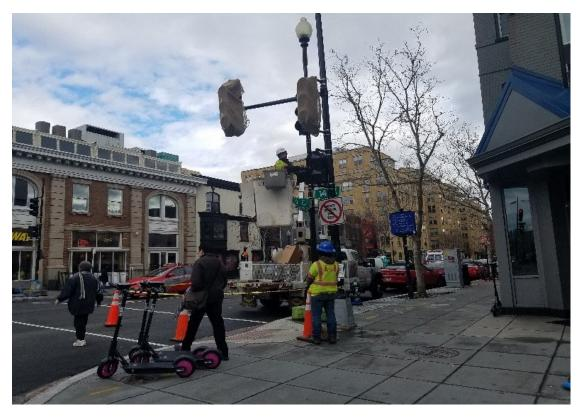
FMCC electrical crew at SEC of 14th & Corcoran St installing flashing beacon system
