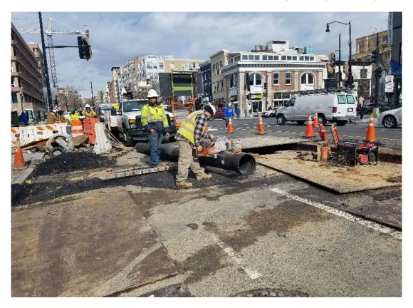
12" ductile iron pipe cut to fit gate valve at water main location
