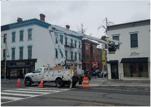
FMCC electrical crew at NWC of 14th & Corcoran St installing flashing beacon system
