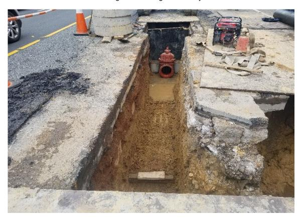
Gate valve previously installed to be connected to 12" D.I.P.
