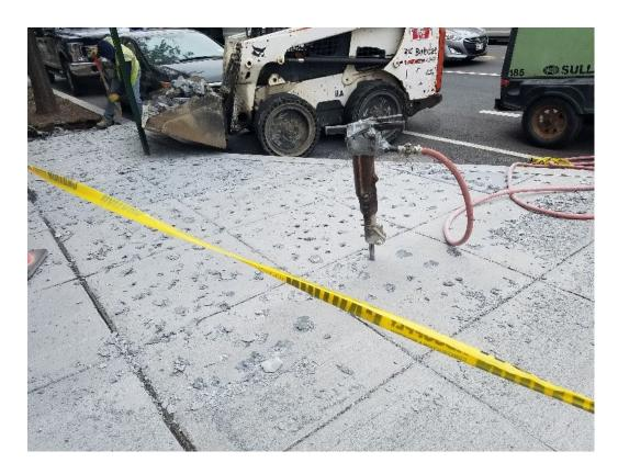
D.E.N. demolished SEC of 14th & Q St PCC sidewalk for tree planter area.
