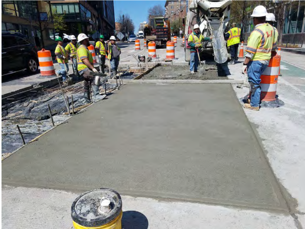
Repair of PCC Pavement at 14 th and Florida Ave
