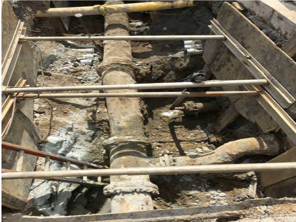
Exposing Water Main at 14 th and T
