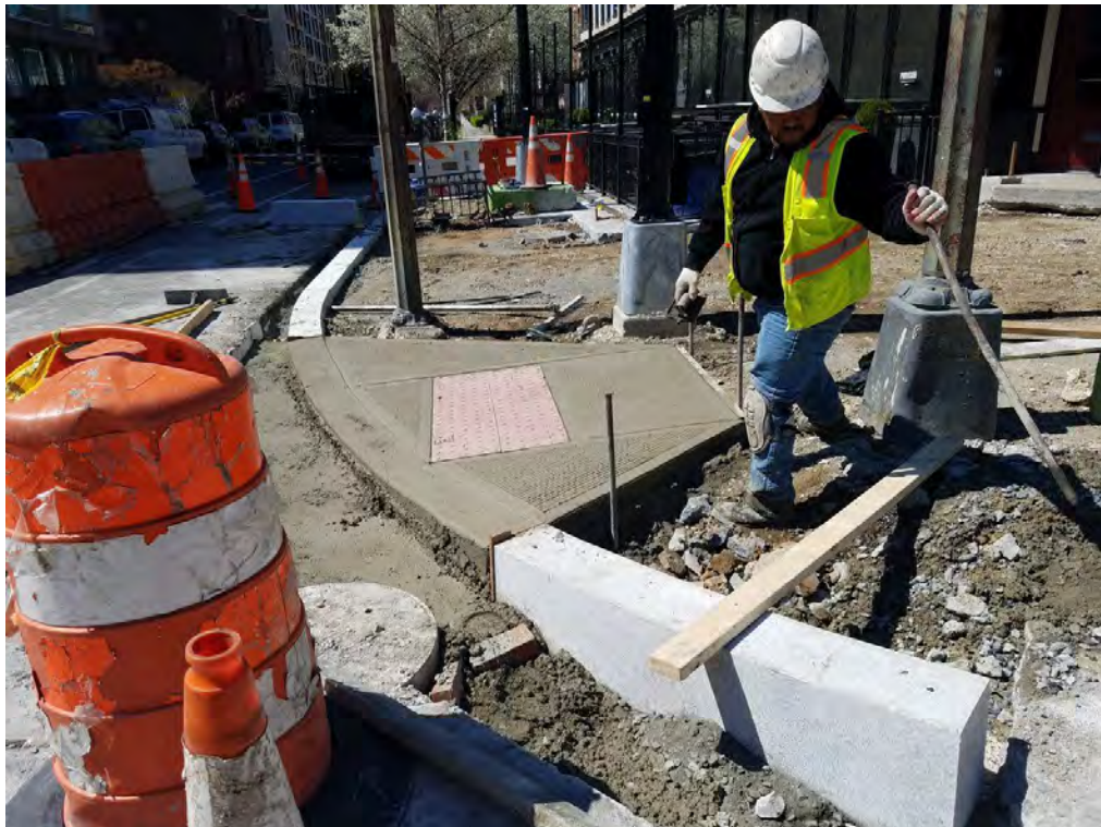
Installation of New ADA Ramp at NW corner of V Street
