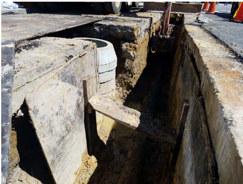
Exposing Water Main at 14 th and V Street for Abandonment
