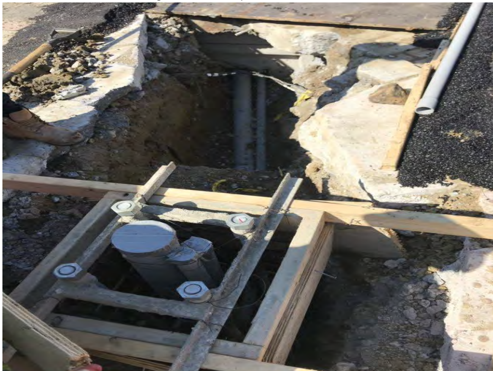
Demo of existing Sidewalk for placement of New PCC Sidewalk
