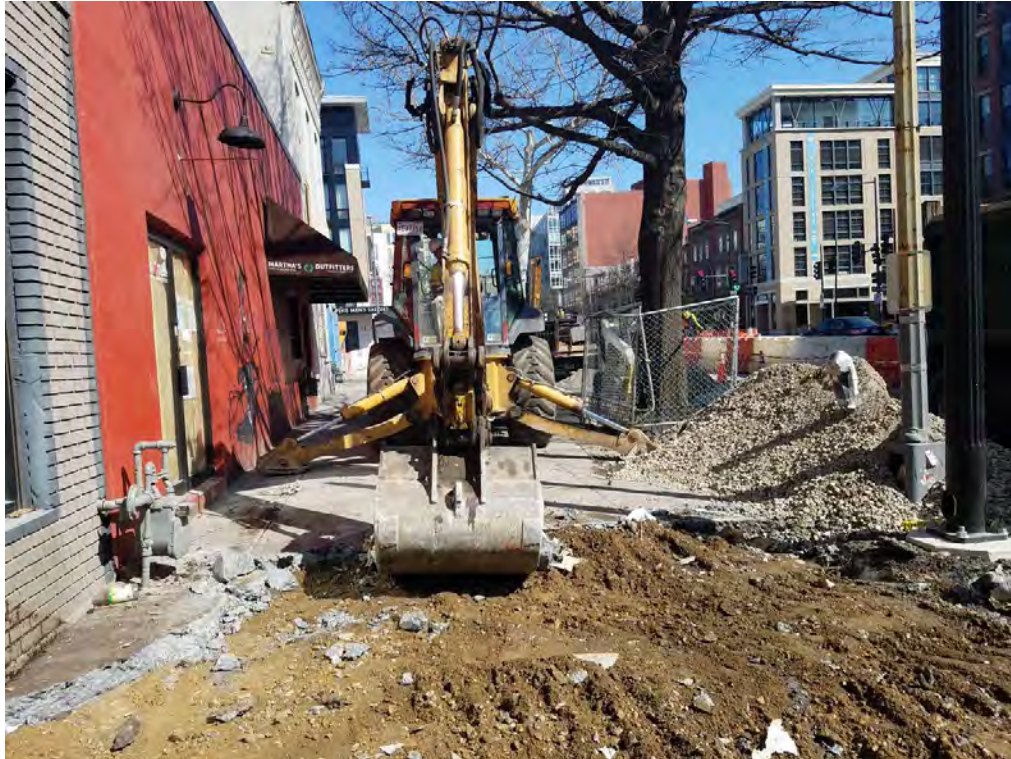
Demo of existing Sidewalk for placement of New PCC Sidewalk
