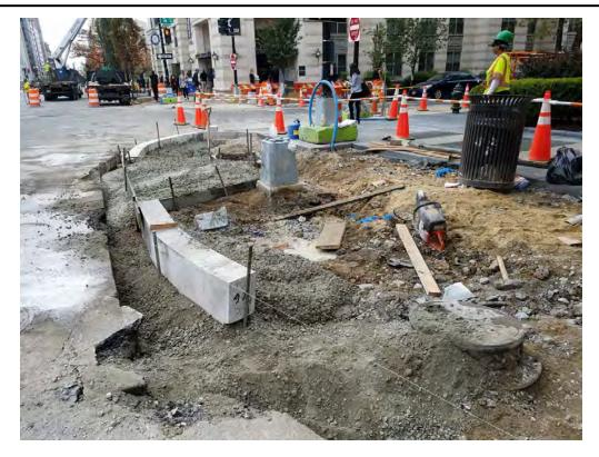
Installation of Granite Curb for Bulb Out at NW Corner of N Street
