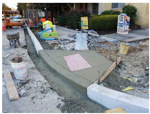
Installation of ADA Ramp at the NW corner of 14th and N Street on the N Street side
