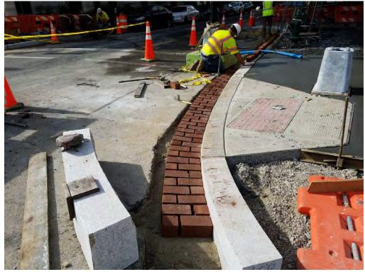
Placing Brick Gutter at the NW Corner of 14th and N Street
