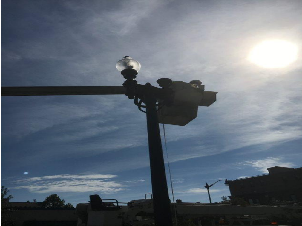
Placing 100-watt LED and Plastic Globe on Twin 20 Street Light Pole
