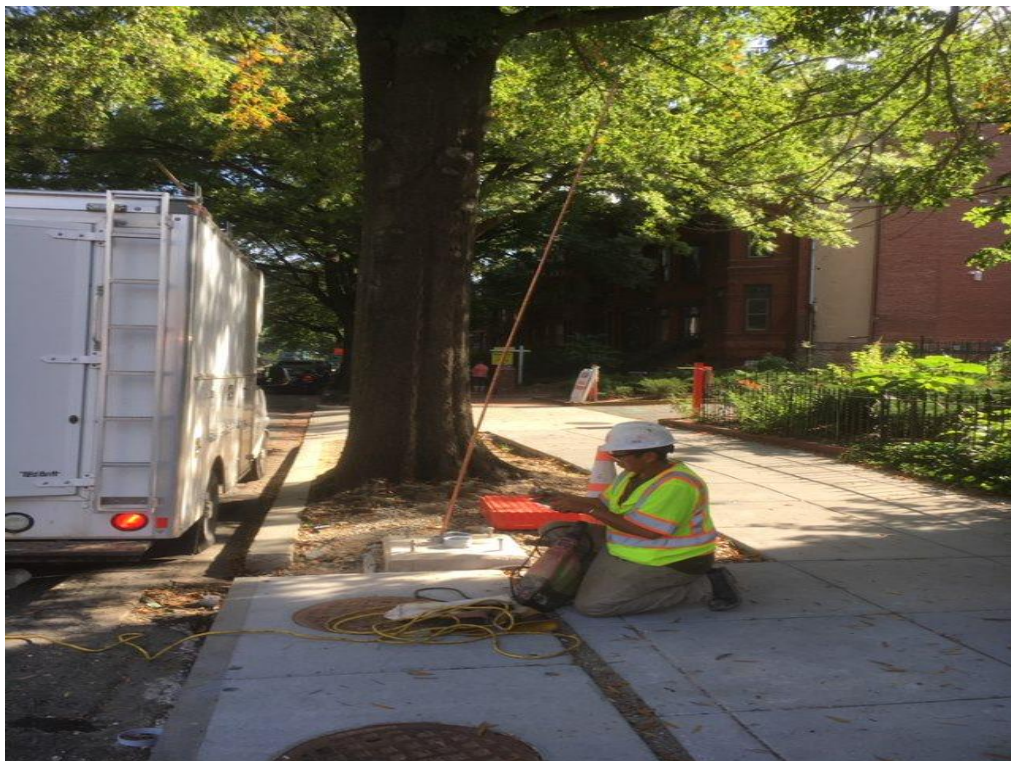
Installing Ground Rod into Traffic Signal Foundation
