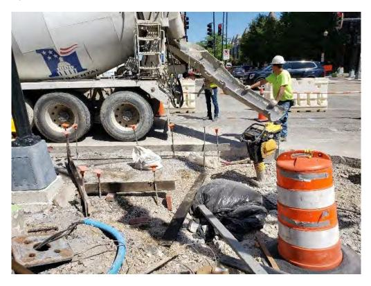
DEN placed Class F, 18 CY for PCC Sidewalk at near Wheel Chair Ramp at Crosswalk at 14th St. & W St. NW.
