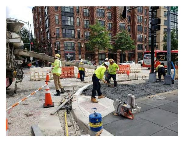
DEN placed 4 CY of Class F (3500 PSI) DC-dot mix at 1 p.m. for PCC Sidewalk plus 9 CY Class F Concrete before Noon. On 8/26/2019 for Sidewalk at 14<sup>th</sup> & W St. NW.
