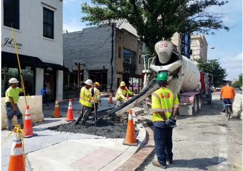
D.E.N. re-pouring PCC sidewalk due to poor quality placement on 8/23/19.
