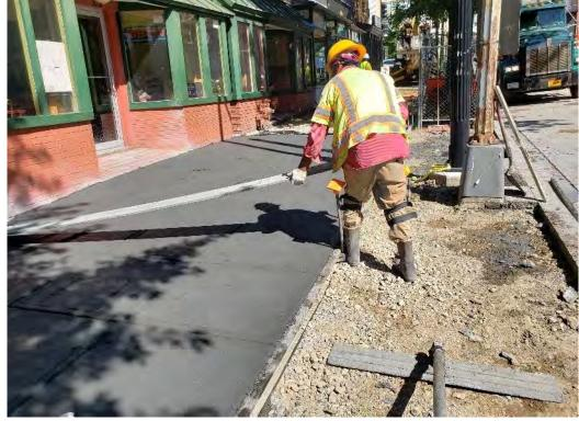
D.E.N placed and finished Concrete sidewalk from 2208 thru 2212 Blocks of 14th St. NW at SB.
