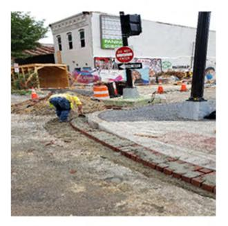
D.E.N. crew also installed and placed 63.4 LF of Brick Gutter at 14th St. & W St. Crosswalk area.
