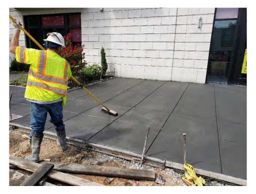
DEN Concrete finishers placed and finished Sidewalk PCC at NWC of 14th ST. and W St. NW.
