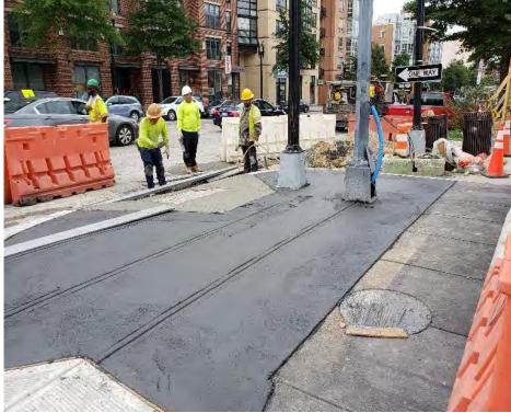
DEN crew adjusted 2 Utility Manholes at the Sidewalk at NWC of 14th ST. & W St. NW.
