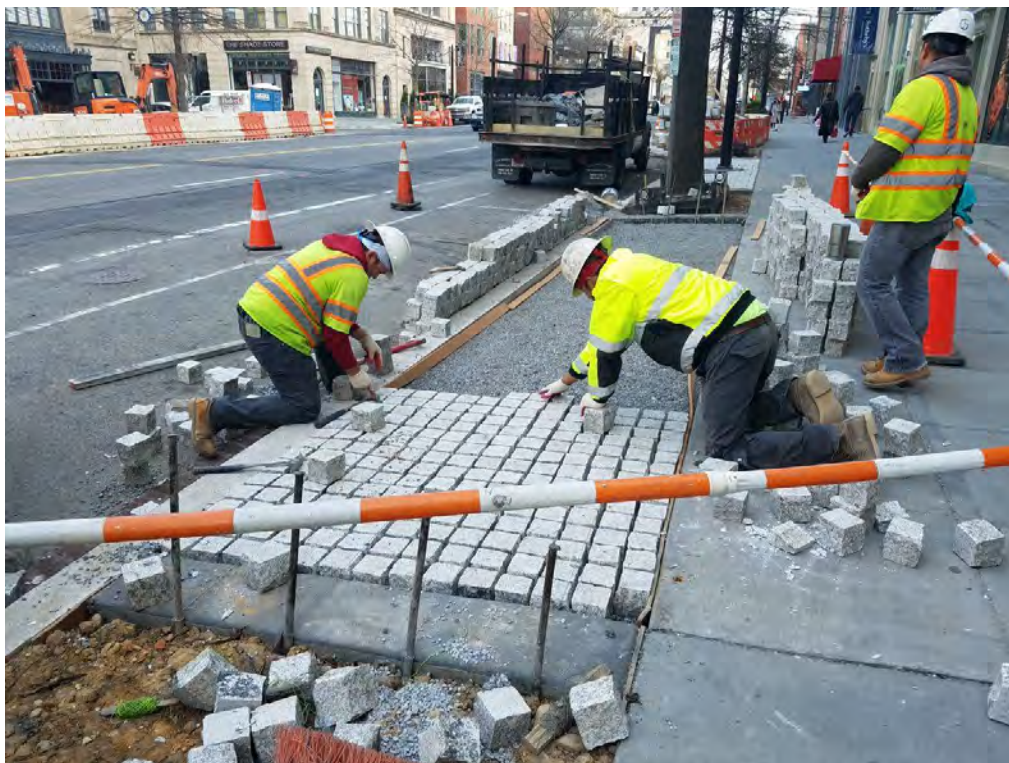
Installation of Granite Cobble Stone between P and Q Street
