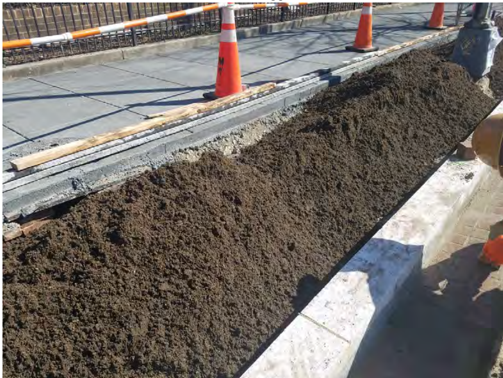
Installation Structural Soil in Tree Box area
