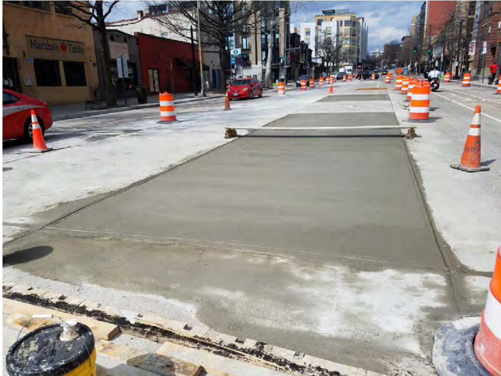
PCC Pavement Repair between V and W Street
