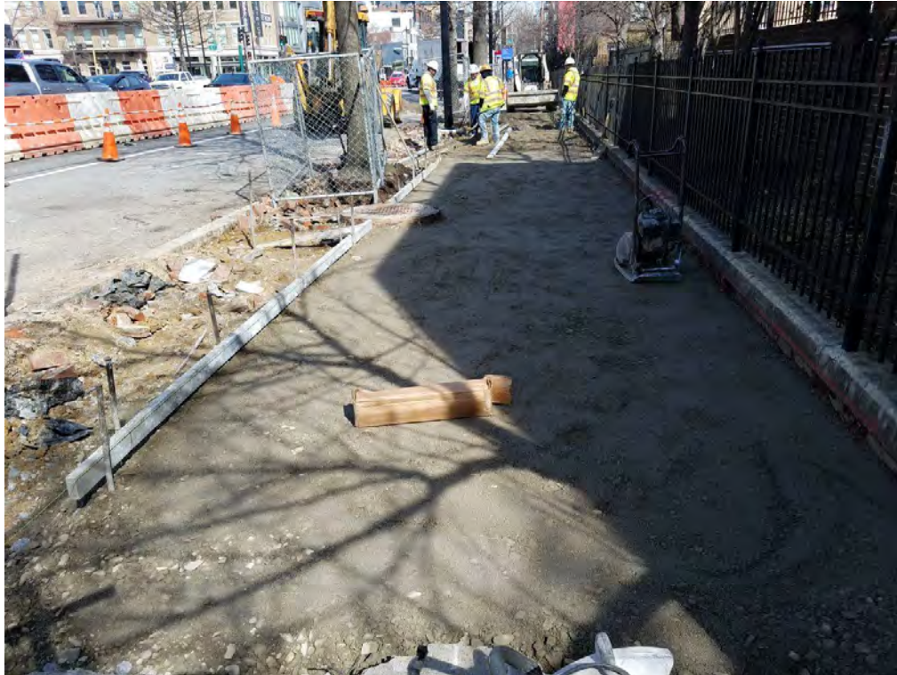
Placement of GAB prior to PCC Sidewalk replacement
