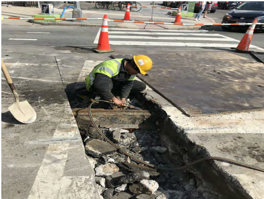
Removal of Old Street Car track at 14 th and S Street
