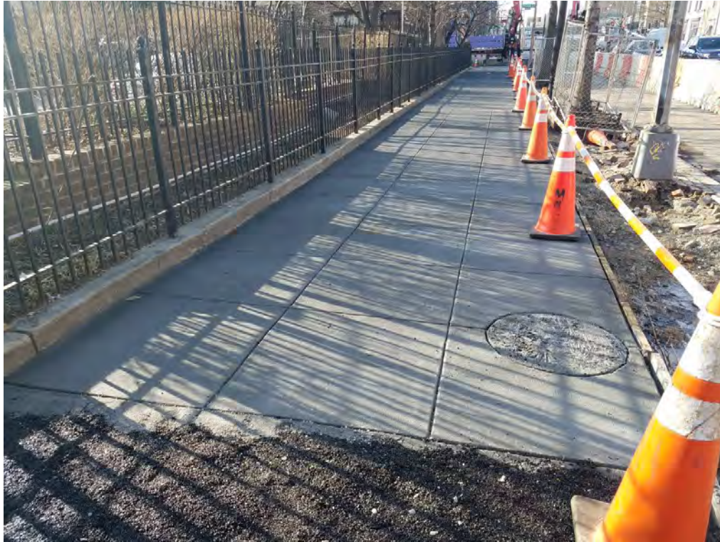
New PCC Sidewalk between Riggs and S Street Eastside
