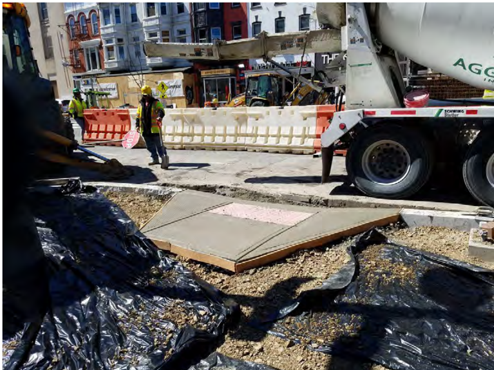
ADA Ramp at the NE Corner of 14 th and Riggs
