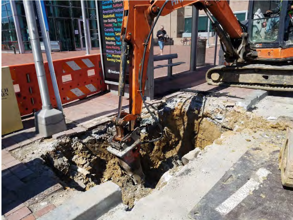
Demo of existing Catch Basin and Connection Pipe
