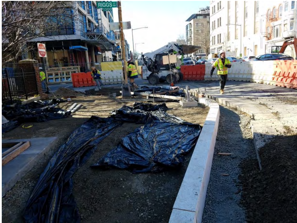
Installation Bump Out at 14 th and Riggs Street
