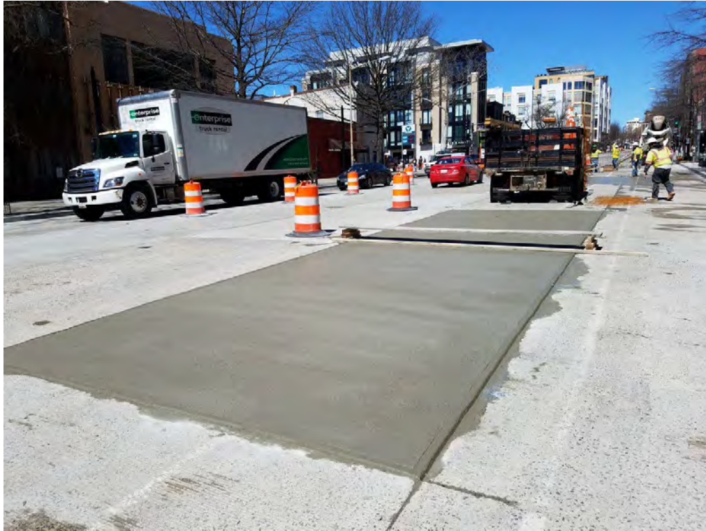
PCC Pavement Repair between Florida and W Street
