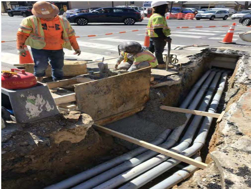
Installation 2" and 4" PVC Electrical Conduit
