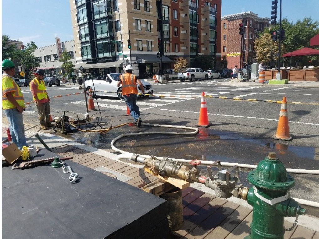
Pressure test gauge losing pressure at NEC of 14 th & R St down 20 psi.
