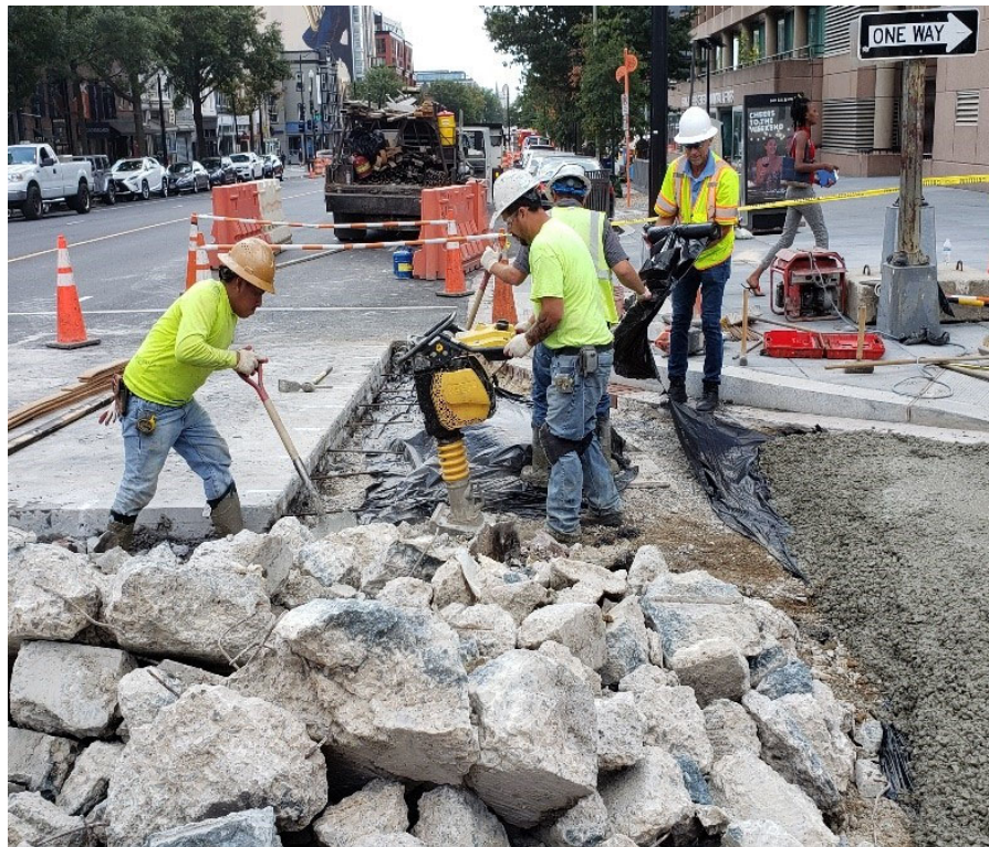
D.E.N crew poured PCC 10" Class E with Roadway Dowels drilled into PCC Base & Wire Mesh at W St. NW & 14 th St. Intersection.
