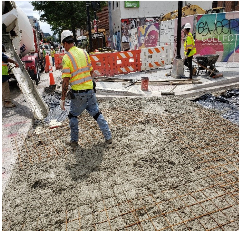
D.E.N crew poured PCC 10" Class E with Roadway Dowels drilled into PCC Base & Wire Mesh at W St. NW & 14 th St. Intersection.
