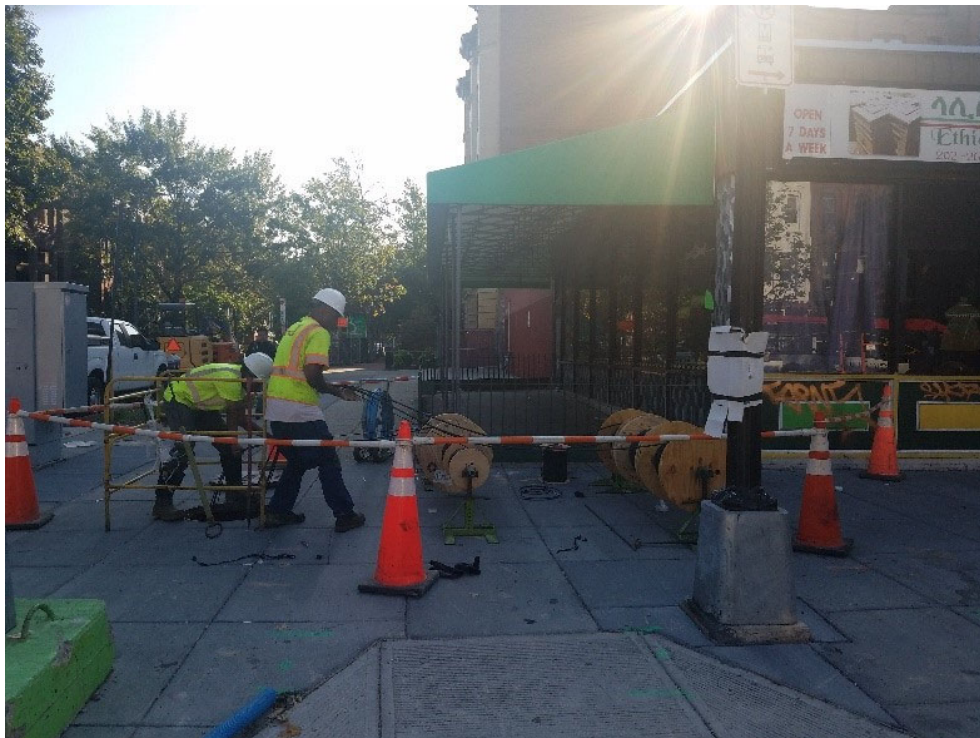
FMCC electrical crew at manhole M26 at SEC of 14 th & P St pulling cable
