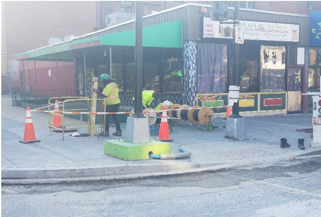
FMCC electrical crew at manhole M26 at SEC of 14 th & P St pulling cable
