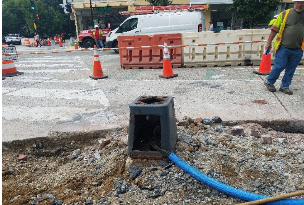
Light pole foundation L95PP/TS to be removed by D.E.N.
