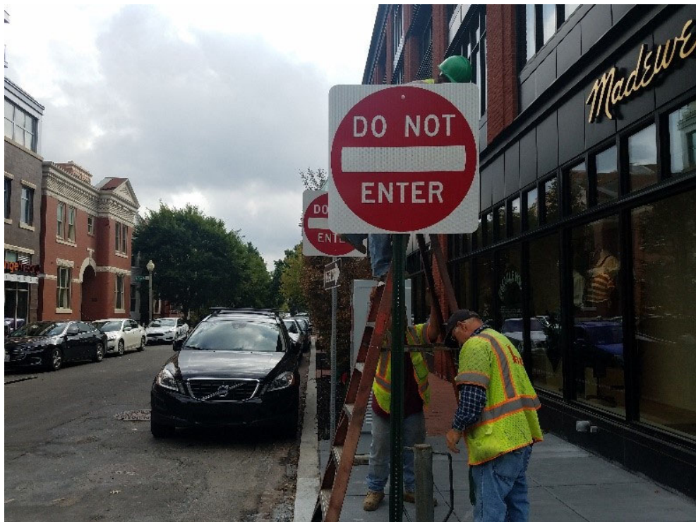
FMCC sign crew installing new signs at 14 th & Wallach St
